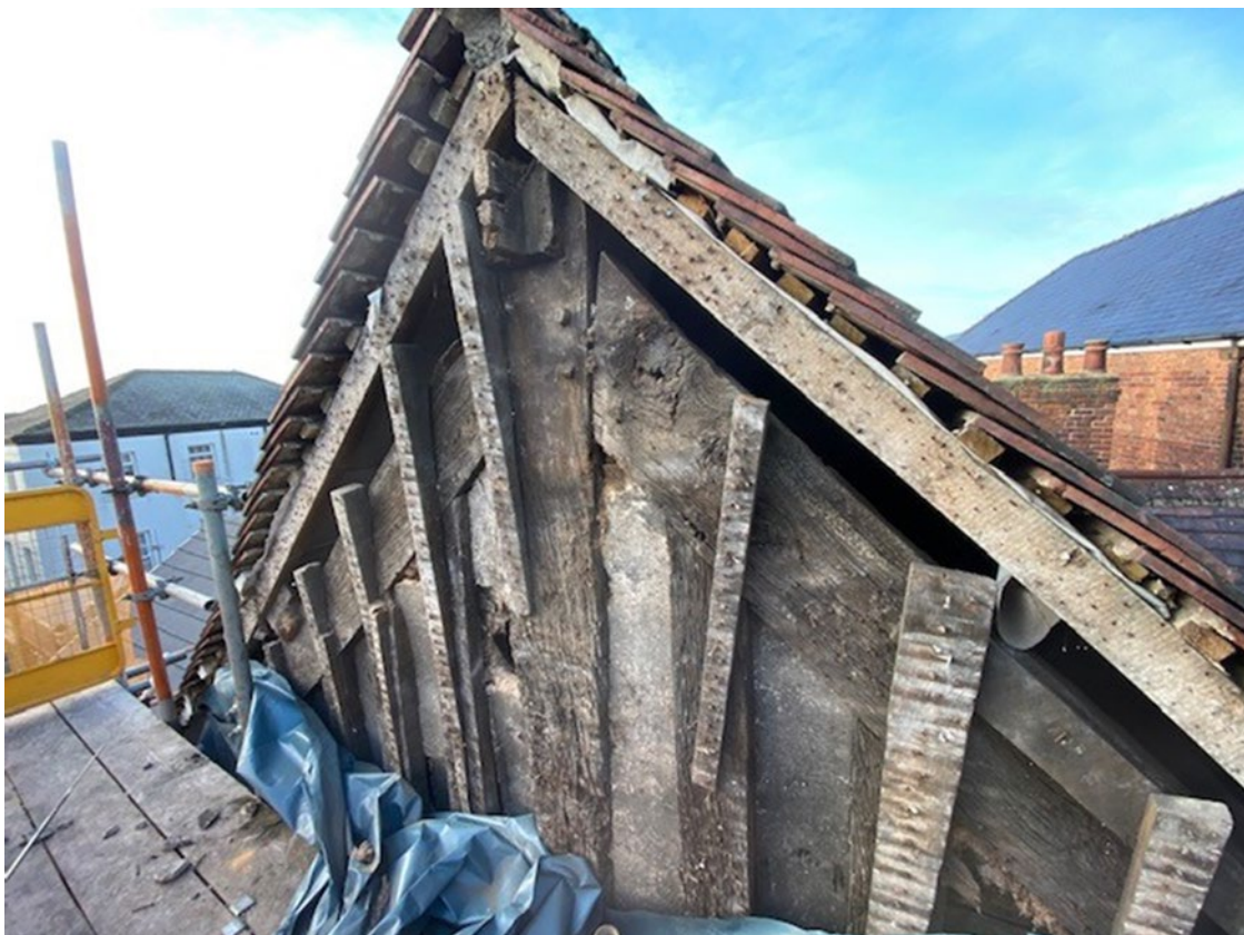
Figure 4: King-post roof, photograph taken from the south-west. [Photograph: Alison Arnold]
