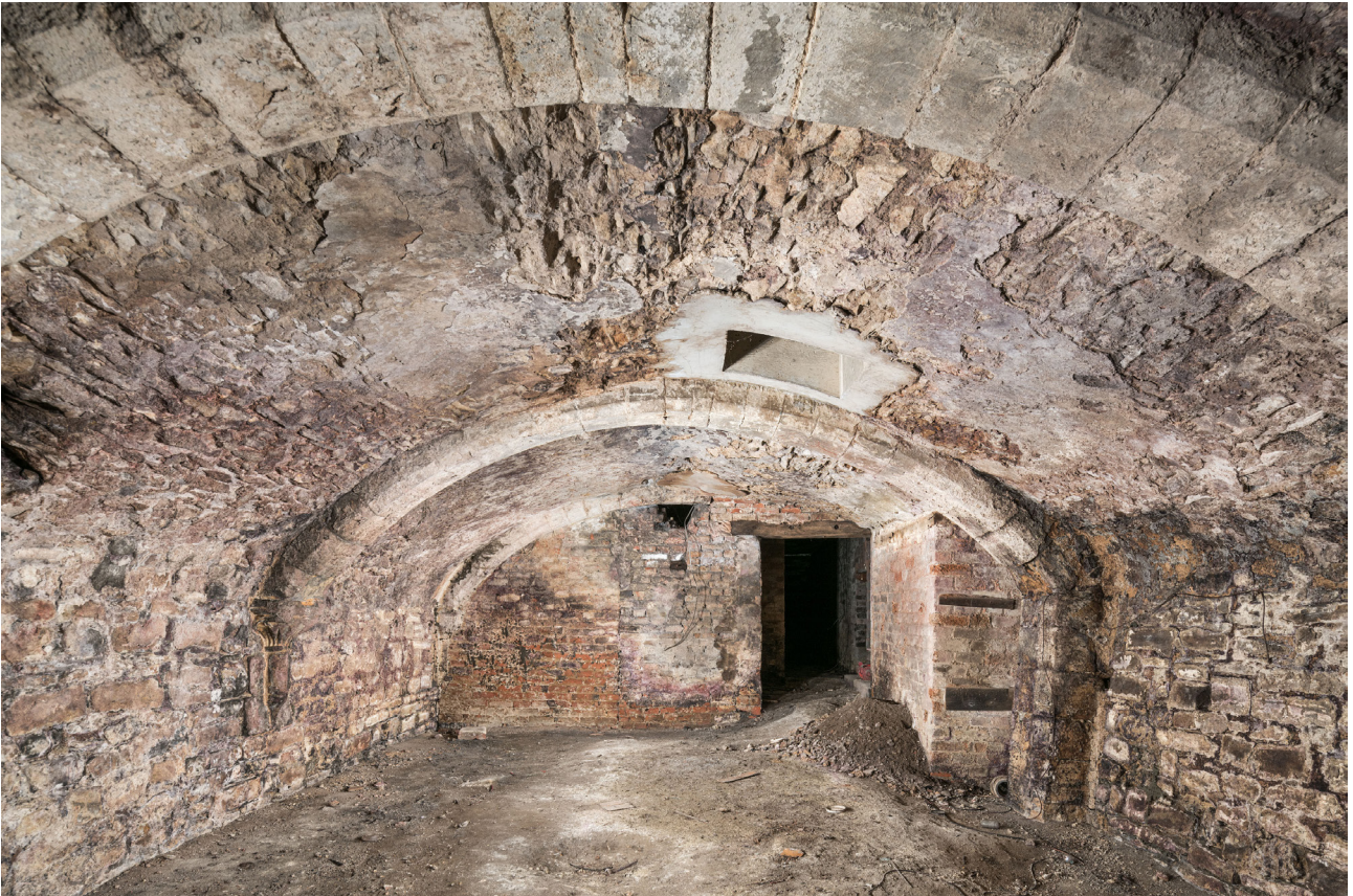
Figure 80: Looking south in the undercroft underneath no. 76 Westgate Street at a later brick transverse partition. [DP325713]
