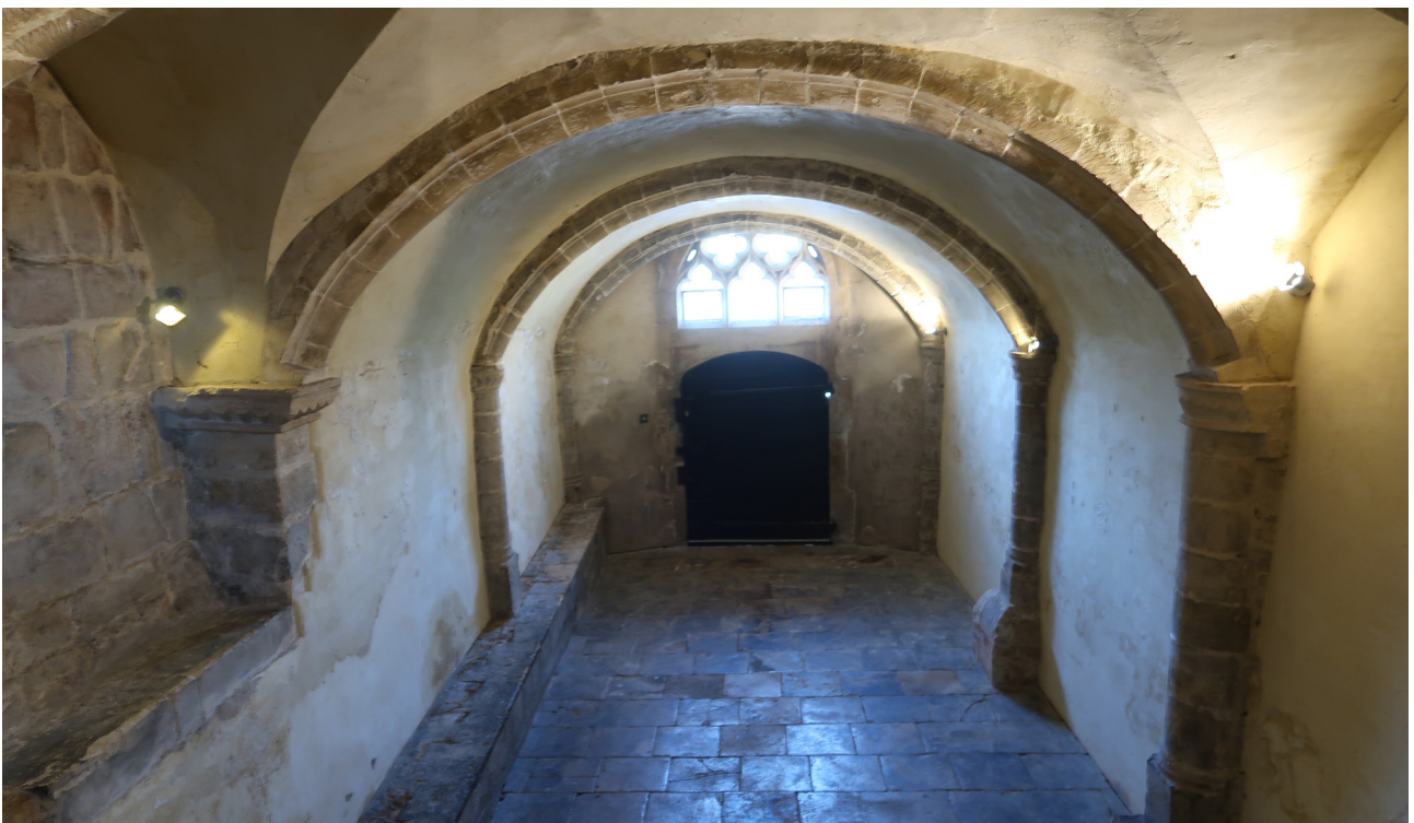
Figure 89: The western slype beneath the former chapel in the abbot's lodgings, looking west, again showing a barrel vault and supporting pillars with scalloped capitals. [Abigail Lloyd © Historic England]
