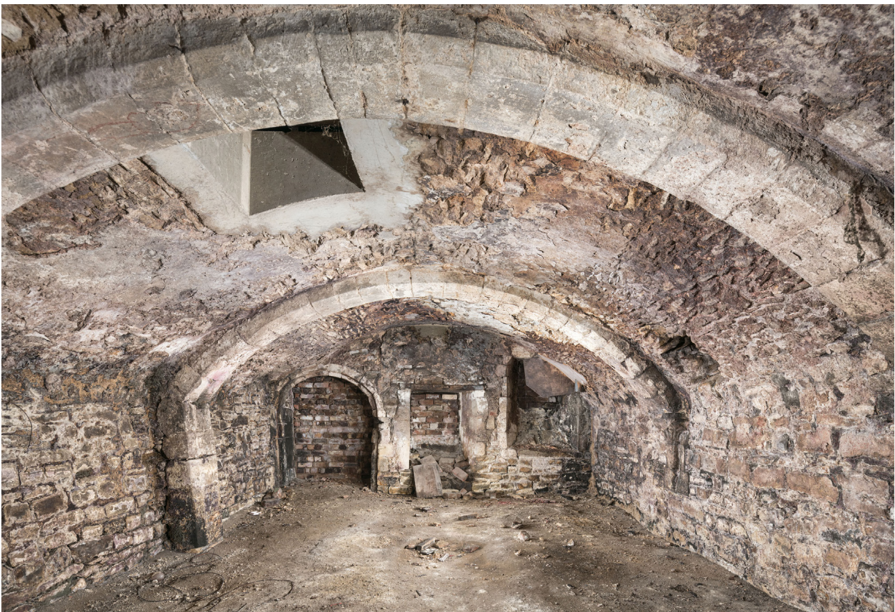
Figure 57: The undercroft at no. 76 Westgate Street looking north. [DP325714]
