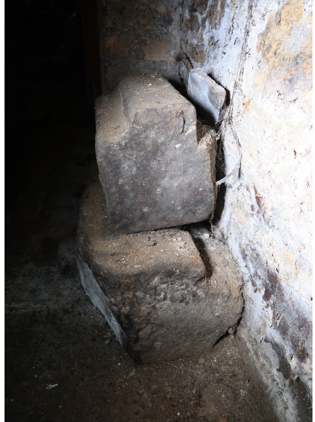
Figure 32: Two stones from the eastern jamb of the doorway from the undercroft of no. 33 Westgate Street, now lying on the floor out of their original position. [Abigail Lloyd © Historic England]
