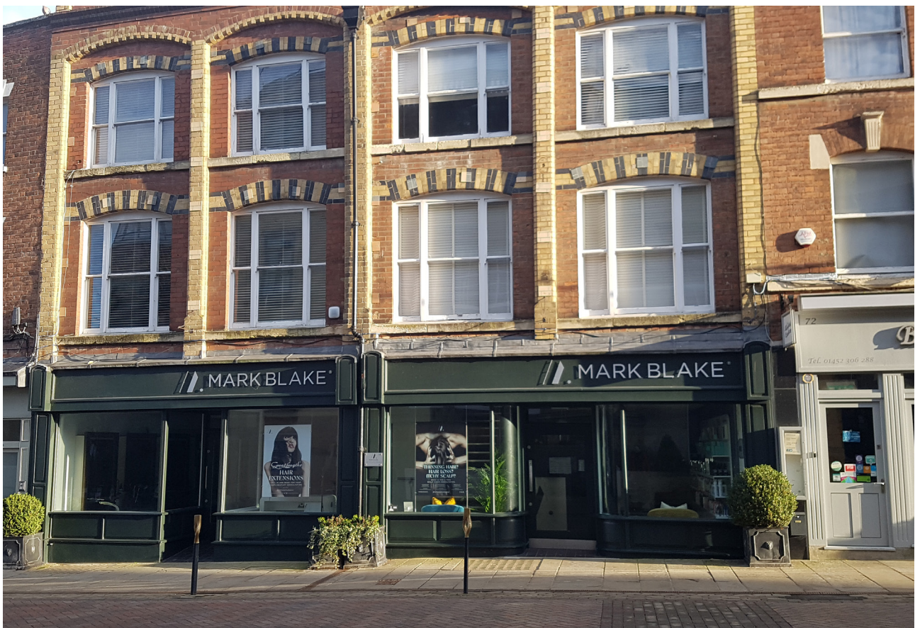
Figure 53: The street frontage of nos. 74 and 76 Westgate Street presenting a unified architectural elevation in March 2023. [Abigail Lloyd © Historic England]
