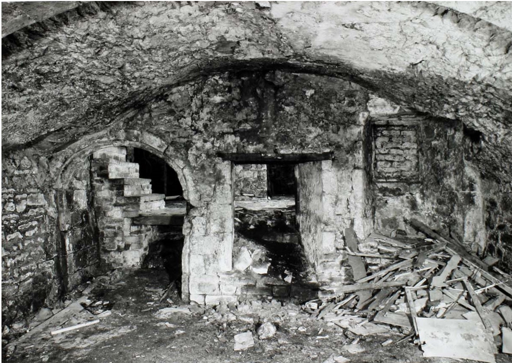
Figure 68: The north wall of the undercroft at no. 76 Westgate Street photographed by the Royal Commission in 1972 when the doorway and central opening were not blocked. [BB72/5668]
