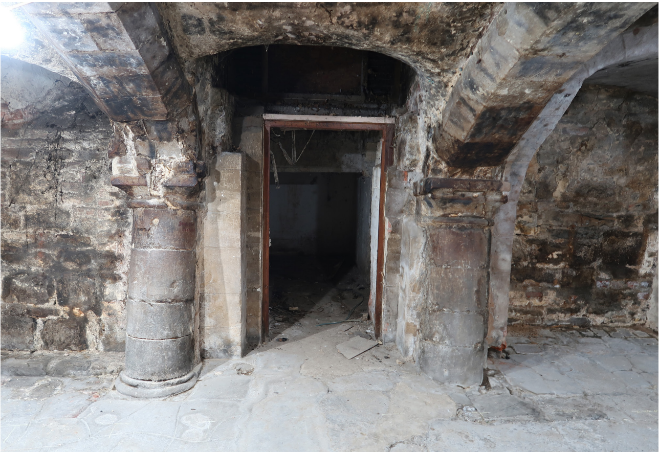
Figure 28: A doorway inserted into an earlier opening in the third bay from the south of the undercroft at the Fleece, leading to an ancillary semi-subterranean room. [Abigail Lloyd © Historic England]
