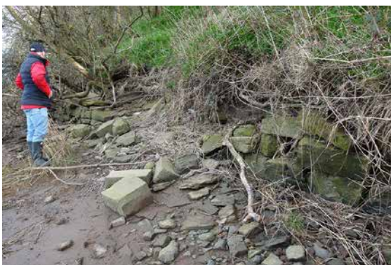
Figure 24: (above left) Short stretches of dry-stone revetment wall at the highwater line on the south bank of the River Tweed, immediately west of Canny Shiel. March 2022. [© Historic England]
