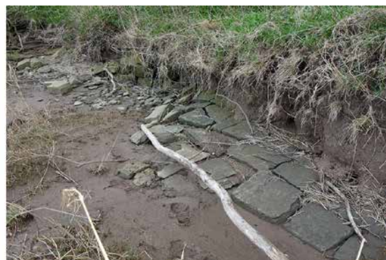
Figure 24: (above left) Short stretches of dry-stone revetment wall at the highwater line on the south bank of the River Tweed, immediately west of Canny Shiel. March 2022. [© Historic England]
