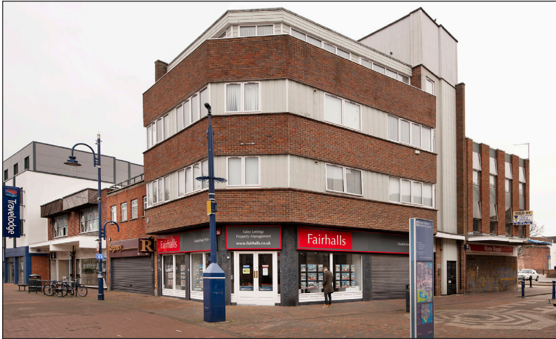
Figure 19: former Leeds Permanent Building Society, 1974-5 [James O. Davies © Historic England Archive, DP276894].
