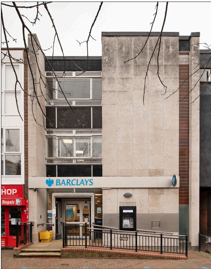
Figure 20: Barclays Bank, 1967 to the designs of Kelsey, Hunter & Partners [James O. Davies © Historic England Archive, DP276931].
