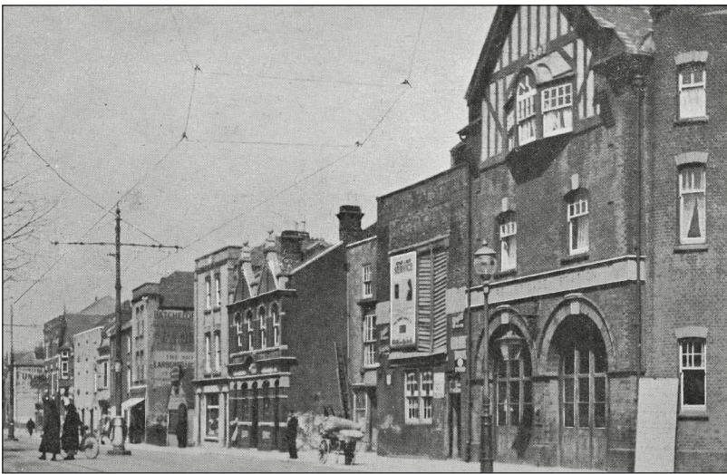
Figure 28: Clarence Road in an old postcard, early 1900s. [Historic England Archive, pen01_11_02_25098a].
