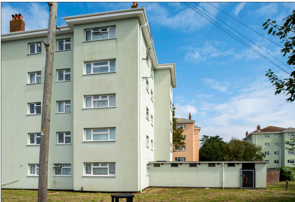
Figure 10: Five-storey Wimpey blocks on Church Path [Elain Harwood, EH00110].
