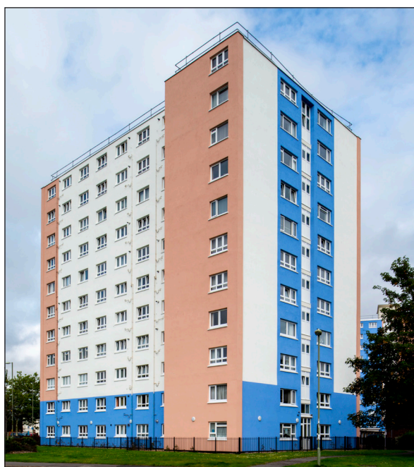
Figure 11: Blake Court, 11-storey Wimpey Block, Haslar Road [Elain Harwood, EH09803].
