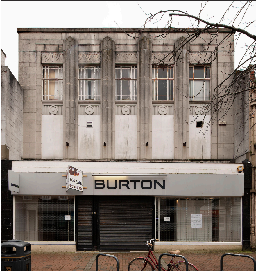
Figure 21: Burton's store, 1930, ground floor remodelled c. 1970 [James O. Davies © Historic England Archive, DP276970].
