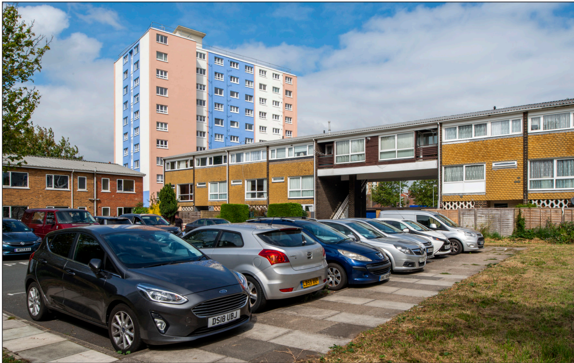
Figure 14: The Mews, with Blake Court behind [Elain Harwood, EH00108].
