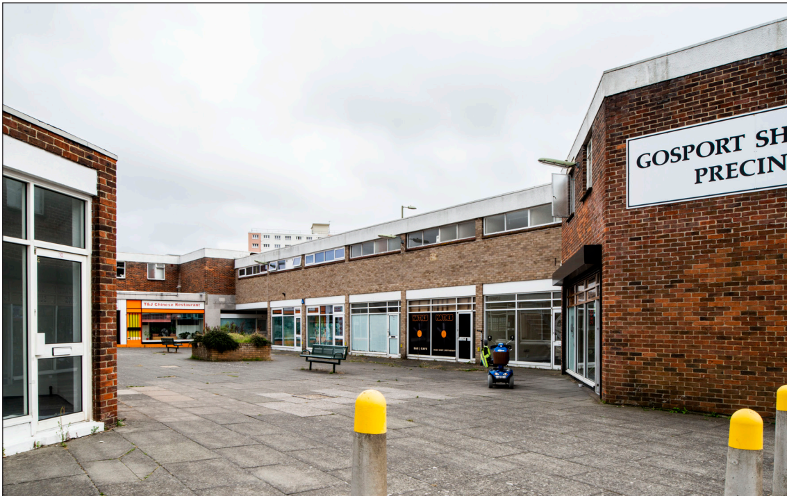
Figure 23: Gosport Shopping Precinct, South Cross Street, 1966-8, architect unknown [Elain Harwood, EH09788].
