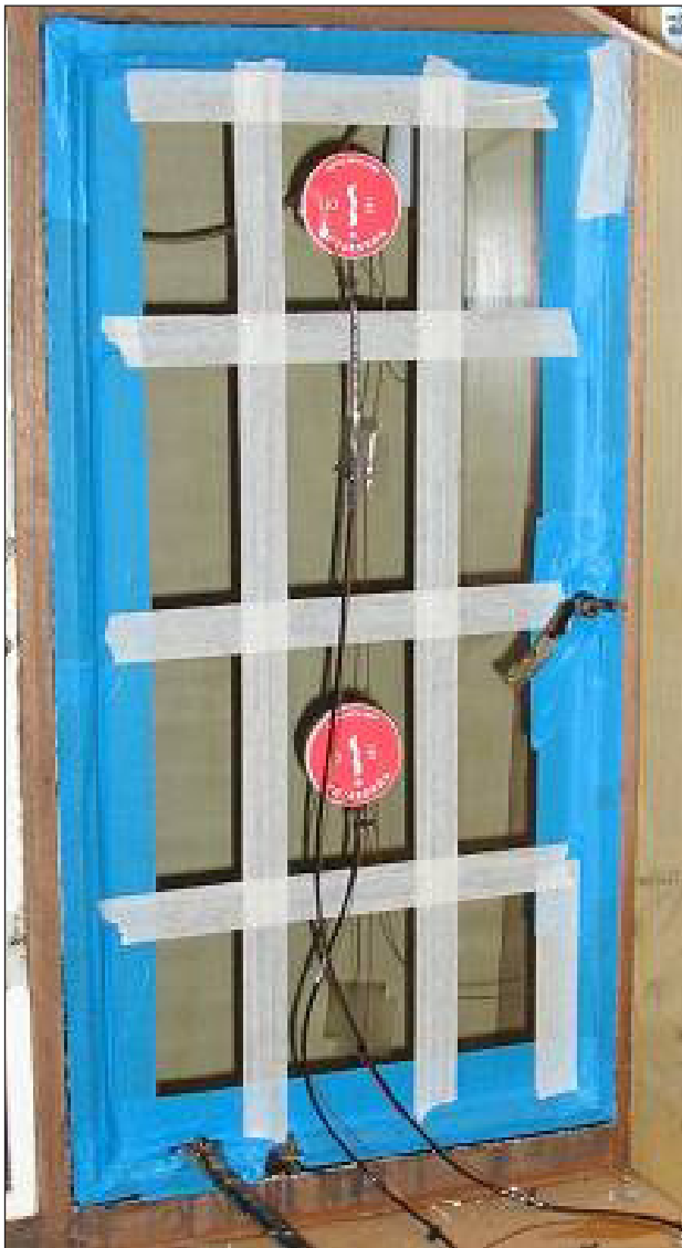
Figure 16: Potential air leakage paths taped over for the measurement of background leakage.
