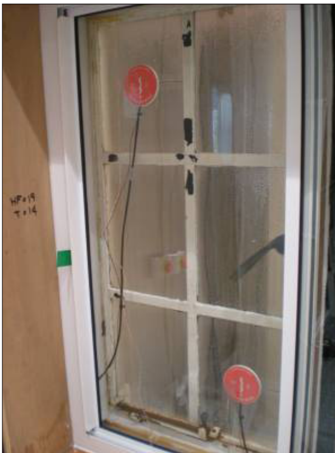
Figure 22: Condensation test with secondary glazing slightly open.
