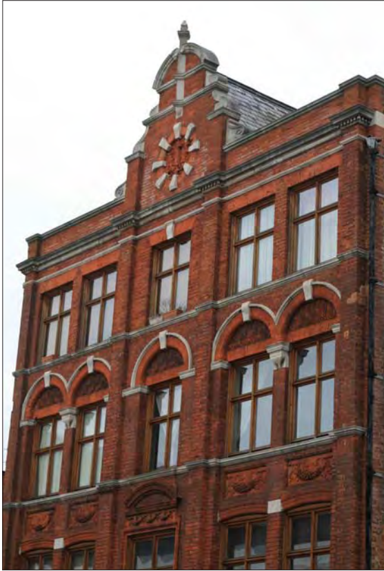
Figure 83. The Balfour factory, 50 Guildford Street. © Katie Carmichael
