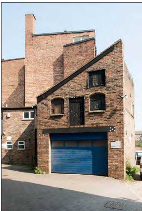
Figure 51. The stables to the rear of 41-43 Guildford Street. © English Heritage NMR DPI41928.
