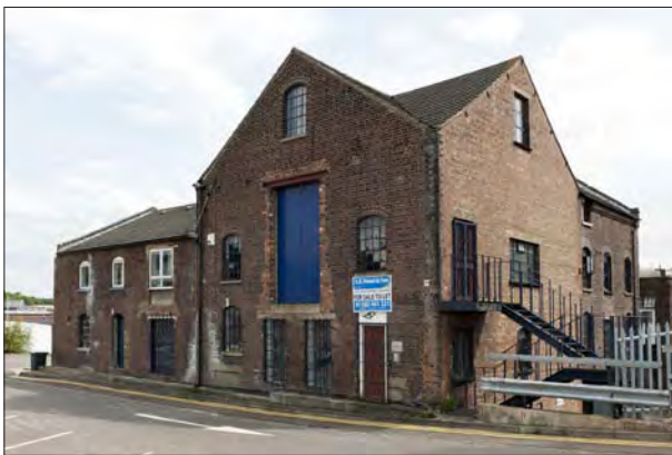
Figure 82. Great Northern Steam Mills to the rear of Guildford Street.
