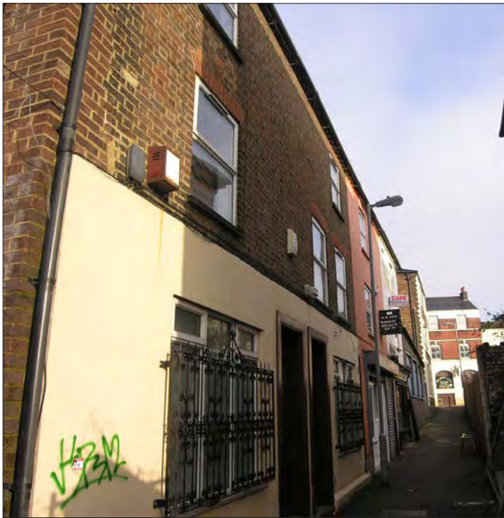
Figure 30. View looking north along Barber's Lane to Guildford Street. © Katie Carmichael.
