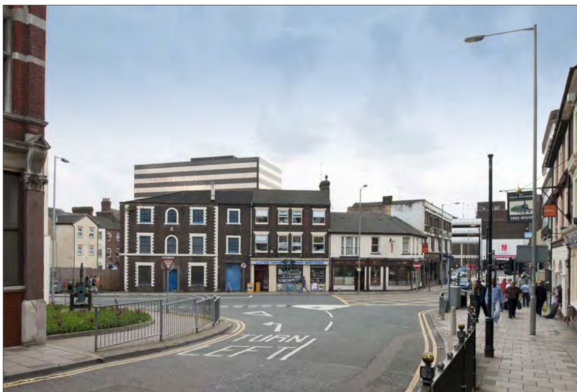
Figure 25. View of the Bute Street/Guildford Street intersection. This is the hub of the Conservation Area and frames most people's view of Plaiters' Lea. © English Heritage NMR DPI46080.
