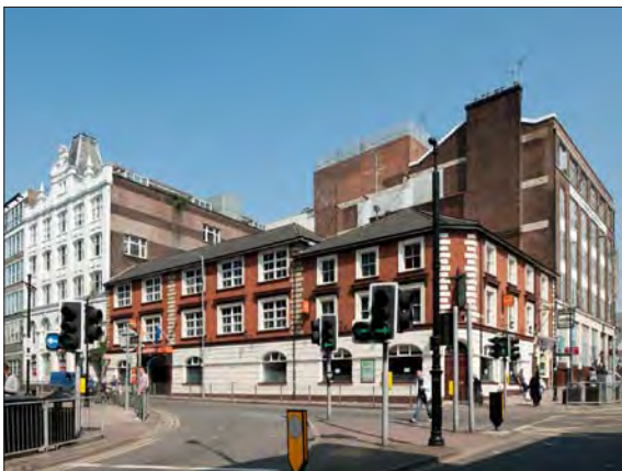
Figure 36. The easyHotel. © English Heritage NMR DPI41936.
