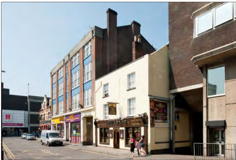
Figure 79. The 'Desert Rose' restaurant, formerly 'The Cooper's Arms', was built in the mid-19th century. The rebuilt Vyse factory lies on its left-hand side in the photograph with 'The Engine' public house beyond this. ©English Heritage NMR DPI41920.
