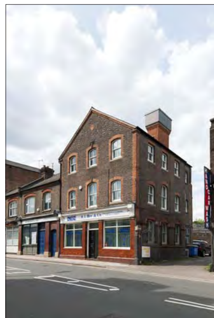
Figure 27. 24 Guildford Street and the entrance to the former Great Northern Steam millyard. © English Heritage NMR DPI46065.
