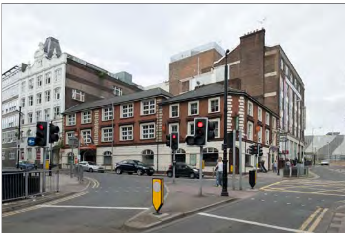
Figure 56. 40a Guildford Street. © English Heritage NMR DPI46075.
