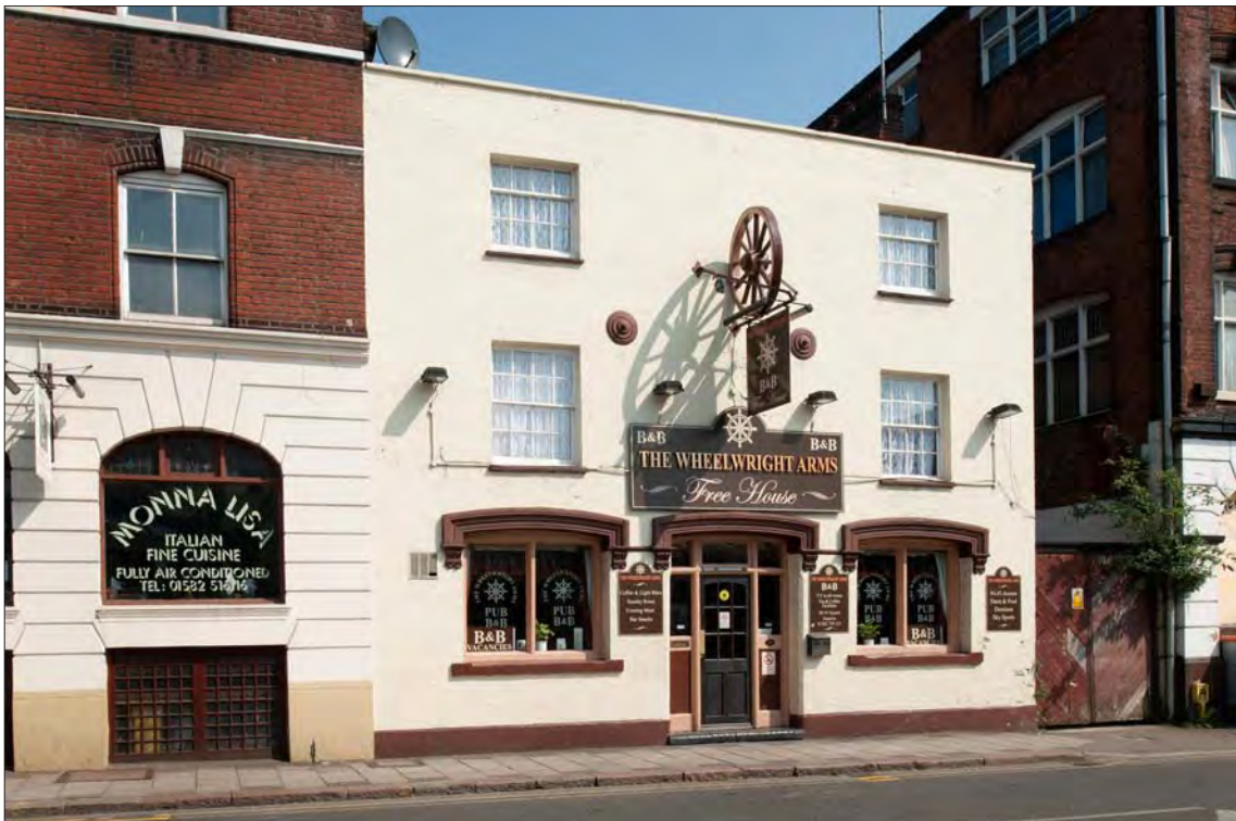
Figure 35. The 'Wheelwright Arms', built c.1840, is one of the most distinctive buildings in the Conservation Area. © English Heritage NMR DPI41931.
