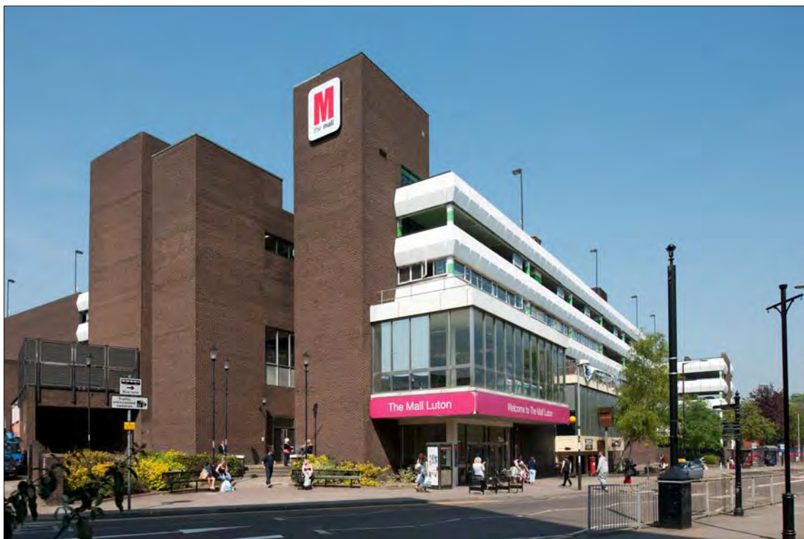
Figure 85. The eastern approach to the Arndale, Luton.
