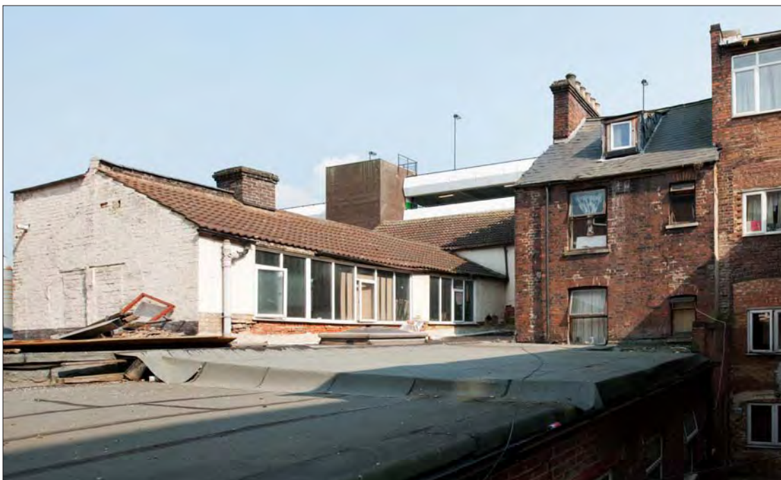
Figure 86. Buildings in a poor state on Melson Street
