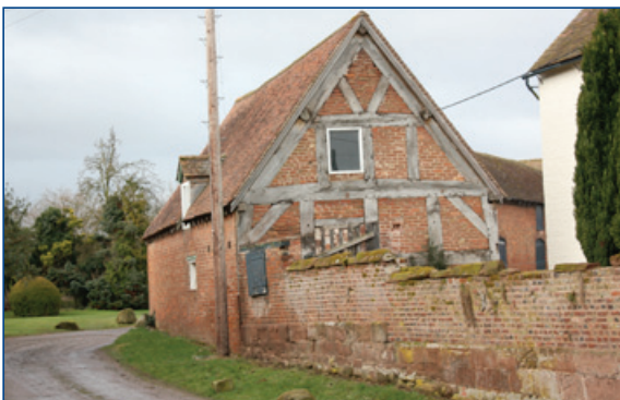
In north Shropshire in particular it is not uncommon to find timber-framed barns that have been clad in brick; in this case the framing of the gable has been left exposed but where the cladding is on all sides only internal inspection can identify the early origins of the barn (Shropshire, Cheshire and Staffordshire Plain).
