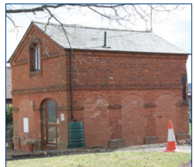
Granaries over cartsheds could allow the loading of sacks of grain straight into carts below through trap doors in the floor (Left and centre: Clun and North West Herefordshire Hill. Right: Arden).
