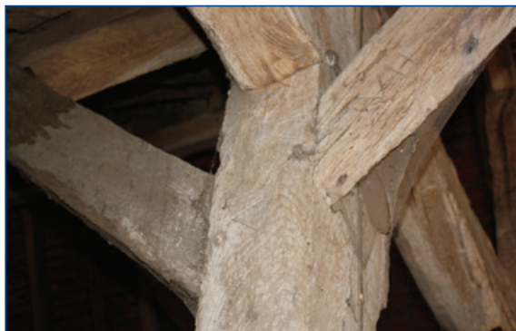
Carpenter's marks on timbers of a timber framed barn (Herefordshire Lowlands).
