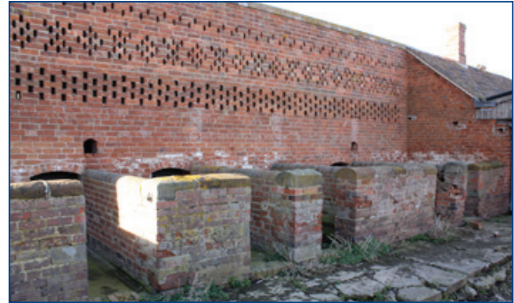
A 'poultiggery' – a series of pigsties with a hen house over forming part of a large regular courtyard farmstead on a dairy farm. The pigsties are located near the farmhouse and dairy (Shropshire, Cheshire and Staffordshire Plain).
