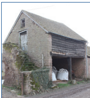
Granaries over cartsheds could allow the loading of sacks of grain straight into carts below through trap doors in the floor (Left and centre: Clun and North West Herefordshire Hill. Right: Arden).
