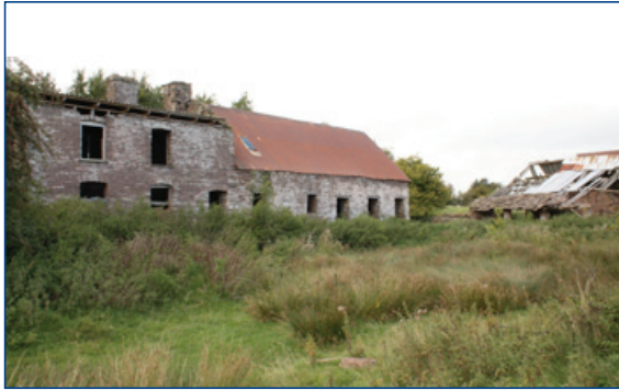
A longhouse in the Black Mountains. Longhouses, where people and animals were housed in a single linear range and shared the same entrance, are more common across the border in Wales.
