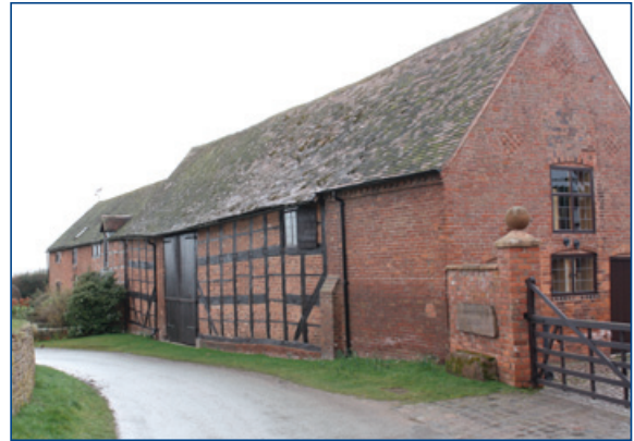
Granaries can be located in the end bay of barns, indicated by a small loading door or external steps (Top: Shropshire, Cheshire and Staffordshire Plain. Right: Shropshire Hills).
