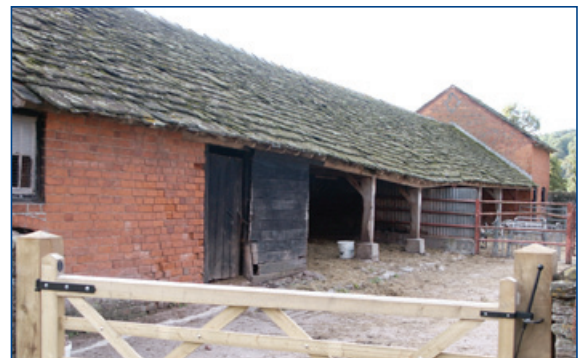
Open-fronted shelter shed facing into a cattle yard where the manure could be trampled with straw before being returned to the fields ((Black Mountains and Golden Valley).
