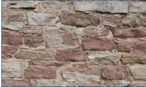
Sandstone rubble is a common material used in the west of the region.
