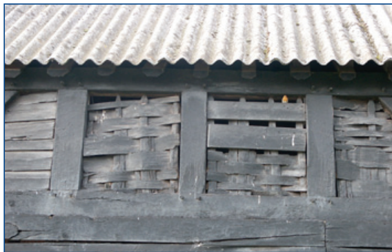
The use of woven laths to fill the upper panels of timber-framed buildings is a characteristic of barns in Herefordshire (Black Mountains and Golden Valley).
