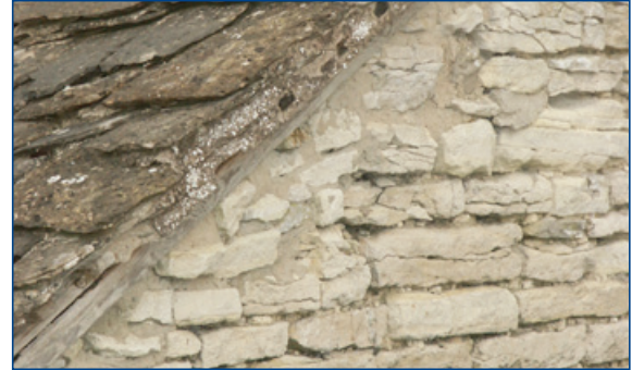
The limestone of the Cotswolds is a distinctive building material used for walling and stone slate (Cotswolds).
