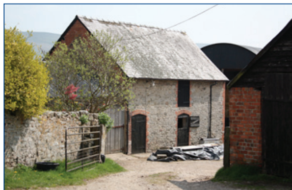
Detached stable building on a medium sized farm (Shropshire Hills).
