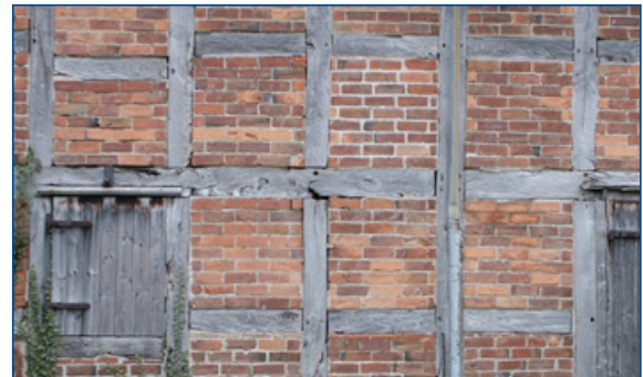
Timber-framing, here with brick infill panels, was a common method of constructing buildings until the 18th century (Herefordshire Lowlands)
