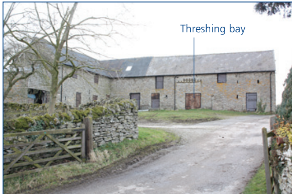
Barns in the West Midlands often formed part of combination ranges incorporating stabling, cattle housing and grain and fodder storage. In this range, the threshing bay has been partially blocked (Shropshire Hills).
