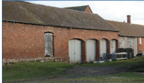
Cartshed bays set into the external wall of a regular planned farmstead (Shropshire, Cheshire and Staffordshire Plain).
