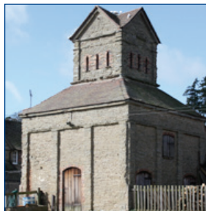
An elaborate dovecote set above a stable. This building forms part of the farmstead associated with an estate (Shropshire Hill).
