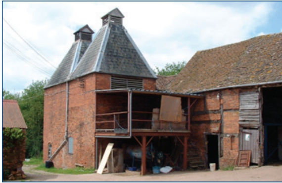
A pair of square kilns with modern staging to give access, indicating the recent continued use of the kiln for drying hops (Herefordshire Lowlands).
