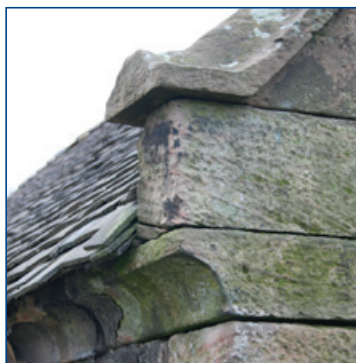
Detail of a fine eaves detail on the gable of a stone cow house (Potteries and Churnet Valley).
