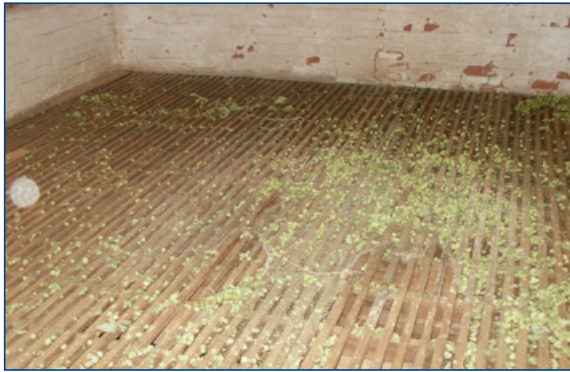
The slatted drying floor of a kiln (Herefordshire Lowlands).
