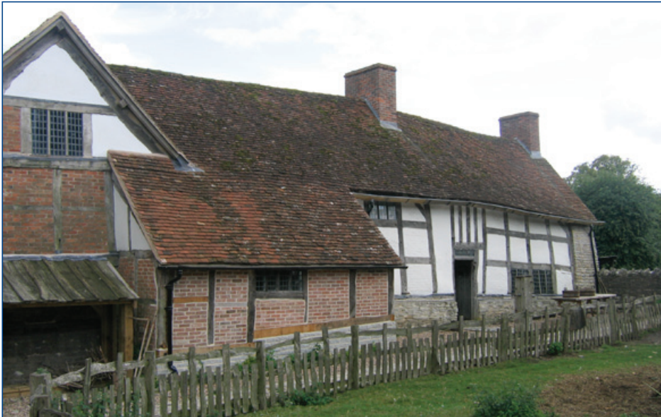
Dairies were often attached to the north side of the farmhouse as a lean-to (Severn and Avon Vales)
