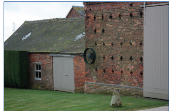
A flywheel attached to the exterior of a barn which would have been powered by a portable steam engine (Cannock Chase).
