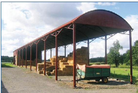
Prefabricated iron framed hay barns became widespread in the late 19th century. Often disregarded, early examples could be of significance especially if they form part of a well-preserved group.
