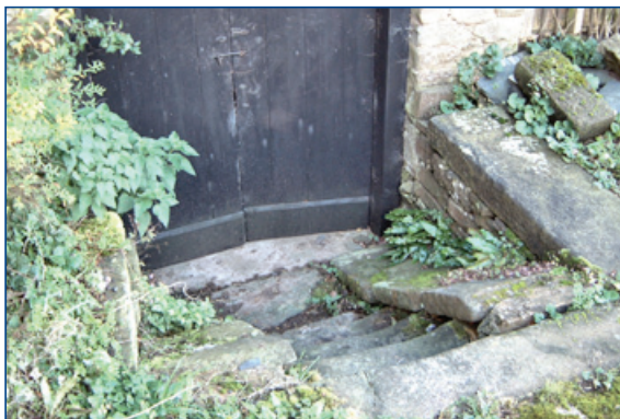
Steps to a cider cellar where the barrels would be stored. Stone ramps either side of the steps aided rolling the barrels in and out of the cellar (Herefordshire Lowlands) © Joan Grundy
