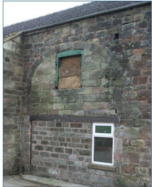
Changing farming practice could leave buildings redundant; the reversion of arable to pasture across much of the north of the region and in more marginal upland areas meant that barns were either replaced or converted to new uses – often resulting in the blocking up of the threshing doors (White Peak).
