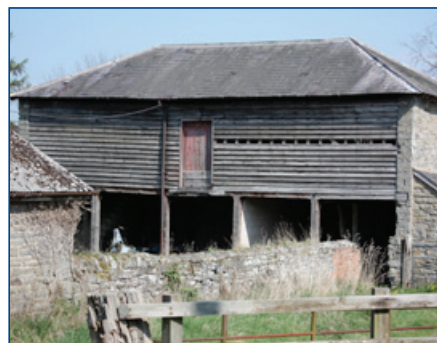
Granaries over cartsheds could allow the loading of sacks of grain straight into carts below through trap doors in the floor (Left and centre: Clun and North West Herefordshire Hill. Right: Arden).
