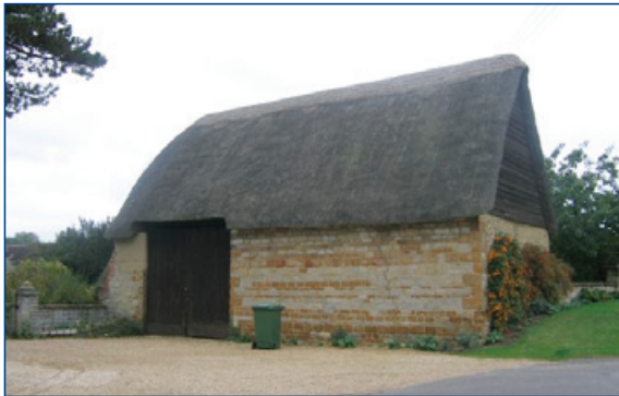
Straw thatch was a common roofing material used in arable areas but it was often replaced with plain tile or pantile. Surviving examples of thatched farm buildings are concentrated in southern Warwickshire (Dunsmore and Feldon).
