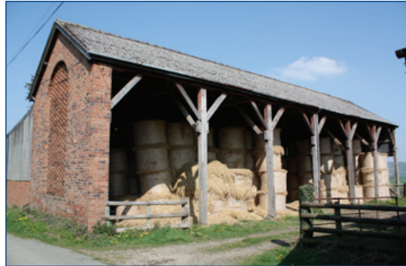
Hay barn with brick gable walls with a large panel of ventilation holes (Clun and North West Herefordshire Hills).
