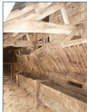
Hay racks within a shelter shed (Clun and North West Herefordshire Hills).
