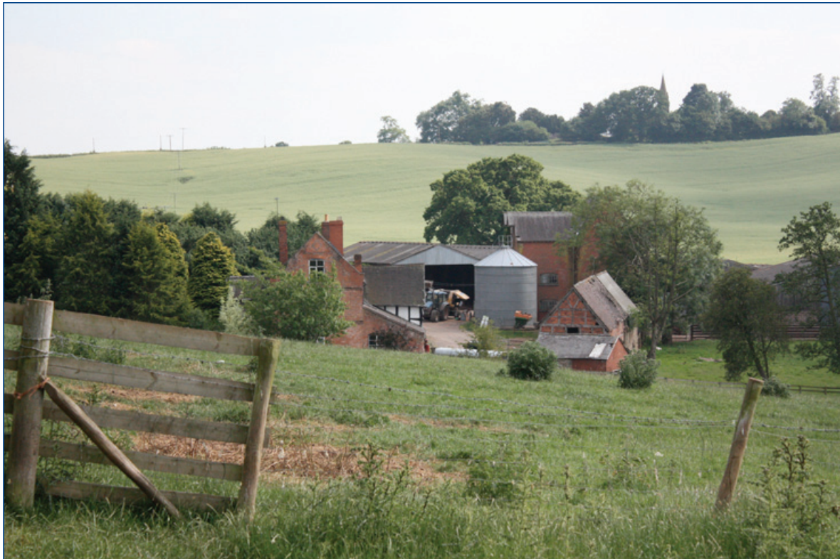
Historic farmsteads often consist of buildings spanning a wide date range and a variety of materials.
