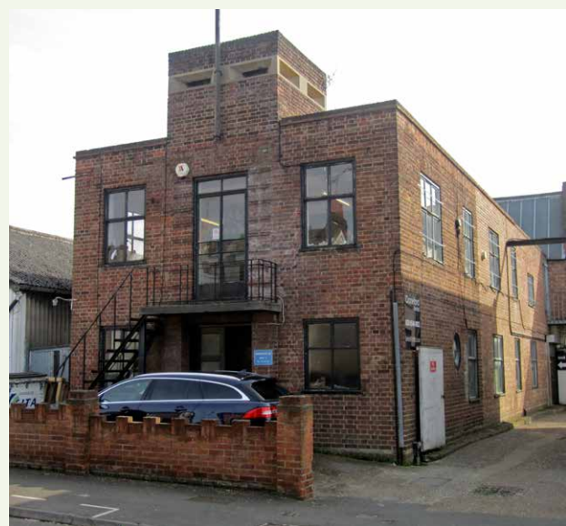
Figure 15: Borough Road, Kingston upon Thames. One of the benefits of the HAA approach is that hitherto unrecognised features of interest may be brought to light. This air raid refuge and canteen block of 1939-40, surmounted by the 1941 addition of a fire watcher's post (1941) was part of a 'key point' factory, essential to war time production. Identified by the Borough Road assessment, it was later listed at Grade II .
