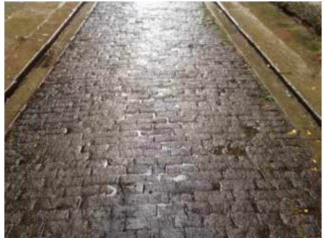
This rare surviving example of timber setting in Rochdale's King Street emphasises the importance of retaining locally distinctive materials or construction techniques.
