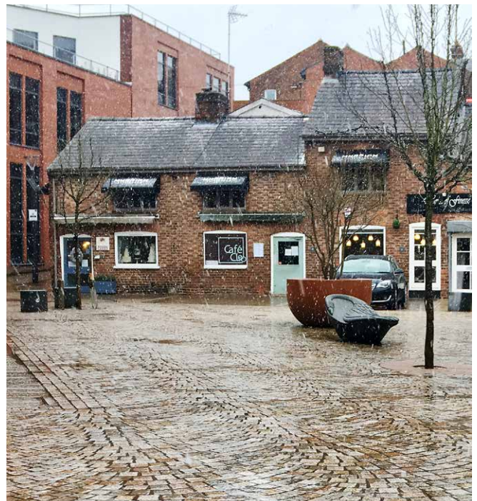
In Goose Green, café tables now spill across the newly laid segmental arch stone paving.
