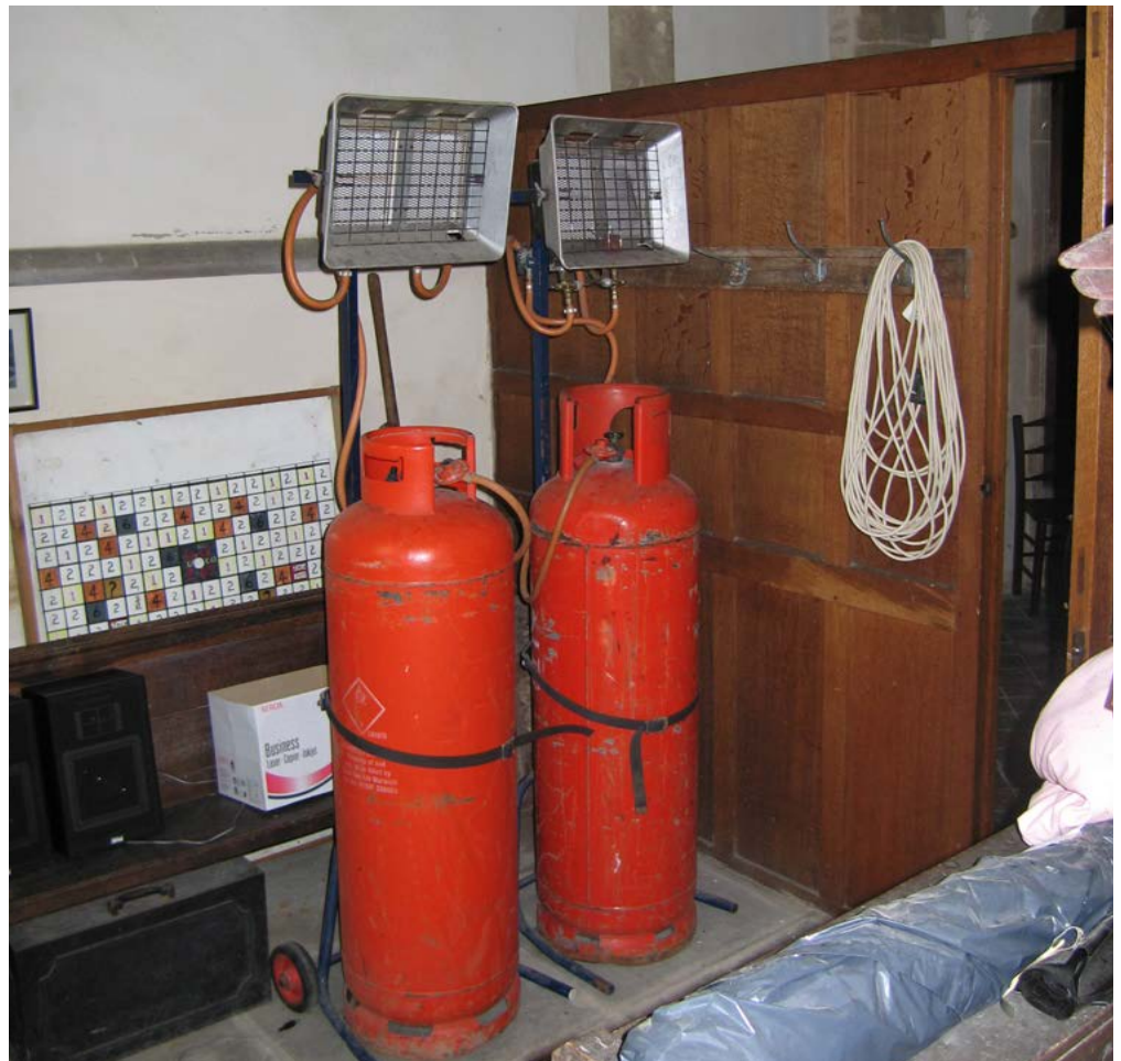
Figure 18 Heaters running on bottled gas are a serious source of indoor moisture, adding to the risk of condensation.
