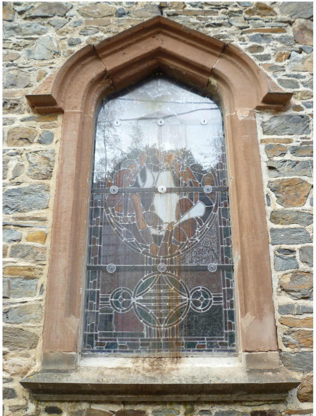
Figure 52 Insects such as wasps and spiders have been observed to nest in unventilated spaces between stained glass and protective sheeting, but there may be some evidence that flying insects are discouraged by the airflow in the EPG interspace. This remains highly uncertain, however.
