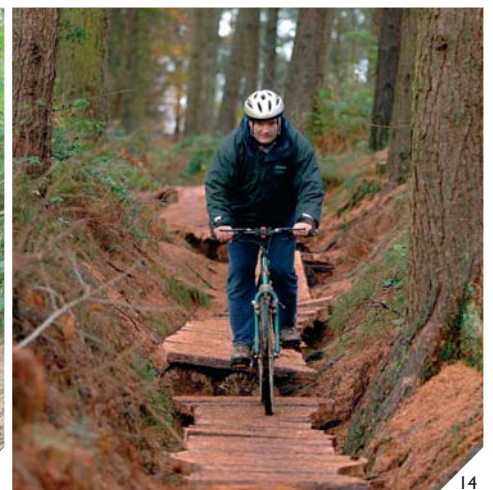
13 & 14 Before and after images of Dargate Dikes, North York Moors National Park: prehistoric linear earthwork in Forestry Commission ownership and suffering from severe erosion caused by mountain bikes. A simple boardwalk trail was constructed as part of an agreed management plan for the site, reducing the impact of the mountain bikes and offering a new non-invasive form of access to the monument.
