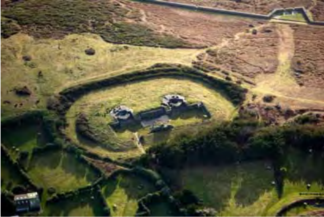
The massive Woolpack Battery of the 1890s, showing the positions for two 6-inch guns and the sunken storage and working areas; also visible are two cruciform structures, modifications made during the Second World War for the erection of radio masts
