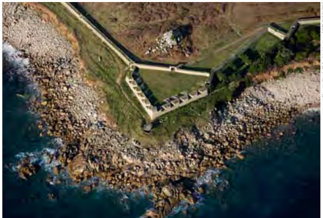
The 1740s battery at Woolpack Point on the southern coast of The Garrison; one of the Defence Electric Lights of the 1890s defensive scheme can be seen in front of the battery; harder to see is the Second World War pillbox inserted into the point of the battery
