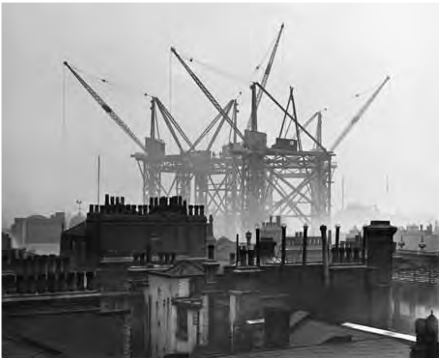
Furness House, Leadenhall Street, City of London, Greater London
