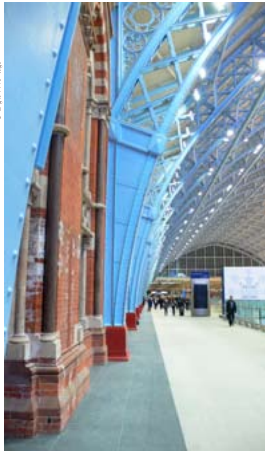
Close-up view of the colour scheme of sky-blue iron trusses and red 'boots'
