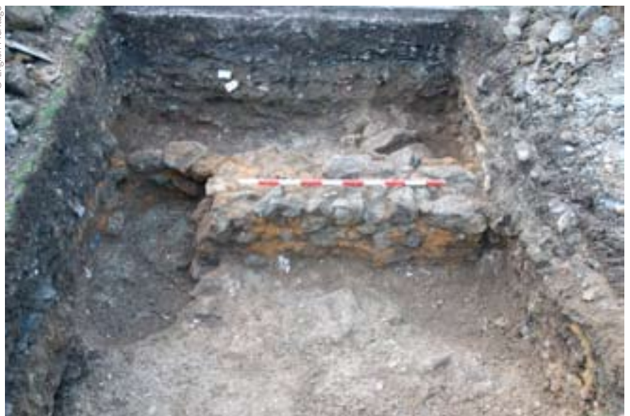
East wall of the south range, looking west. Its southern end is cut by a large pit possibly dug to plant a shrub
