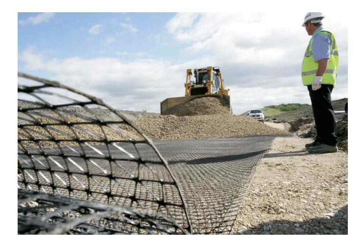
**Figure 9:** Example of a geogrid, used to spread a load. [© Tensar International]
