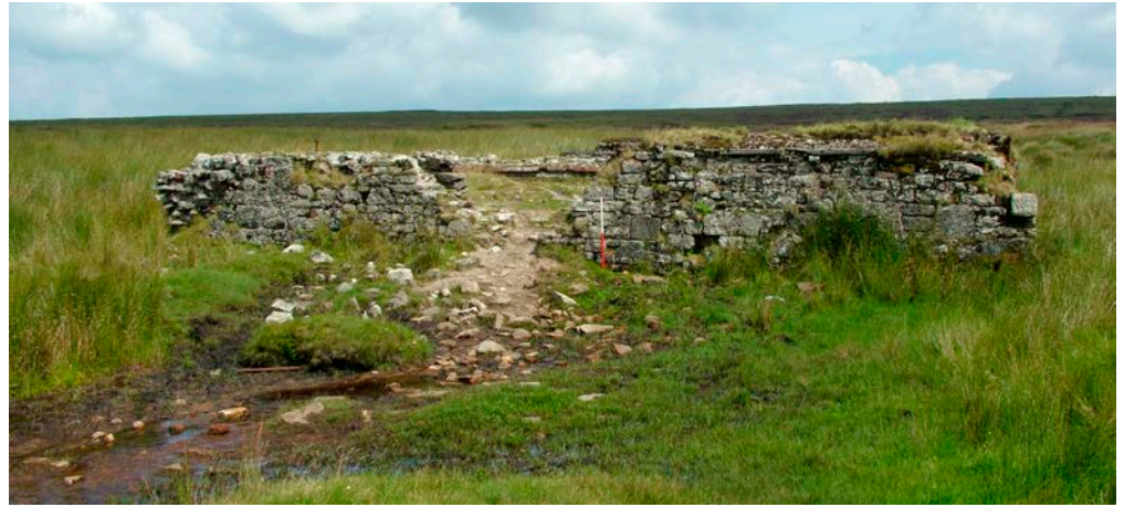
Figure 12: A ruined and part-demolished peat charring oven at Rattlebrook Head Peat Works, Dartmoor, installed in the late 1870s. © Phil Newman.
