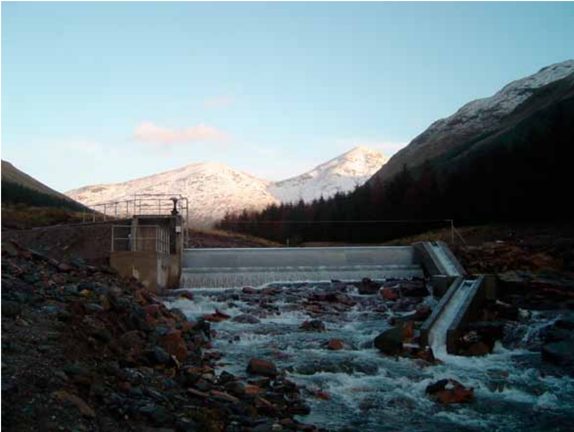
Weir and fish run (Dulas Ltd)
