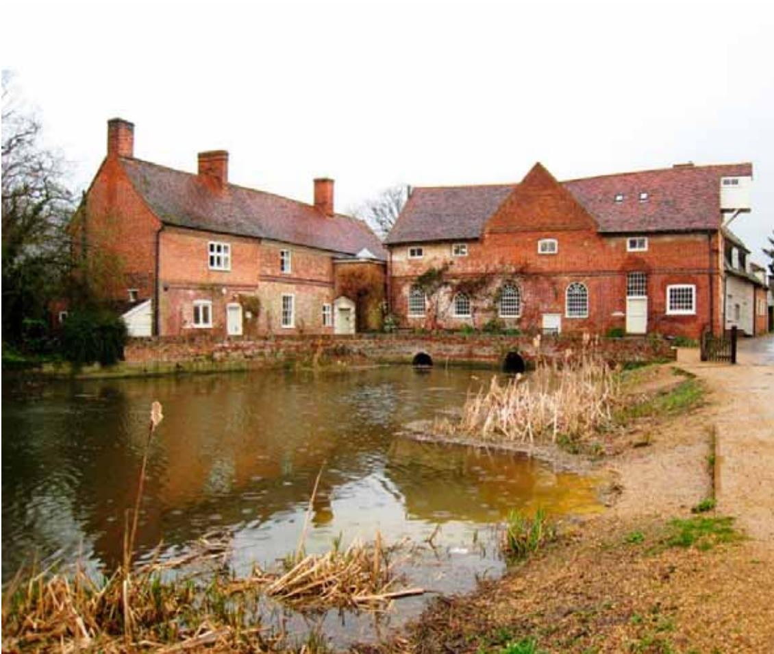
Flatford Mill has recently had an Archimedes screw turbine installed (Photo courtesy of MannPower consulting Ltd)
