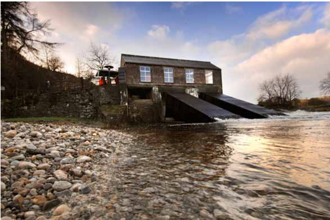
Linton Falls: A community restoration of a hydroelectric scheme (images courtesy of JN Bentley Ltd/Morgan O'Driscoll photography)
