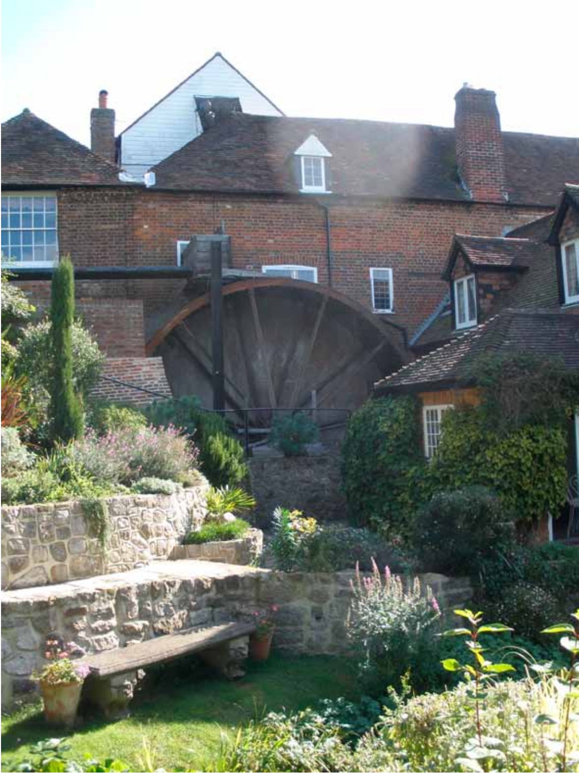
21' x 5' Overshot Wheel at Hythe Mill in Kent (Photo courtesy of Stephen Bartlett)
