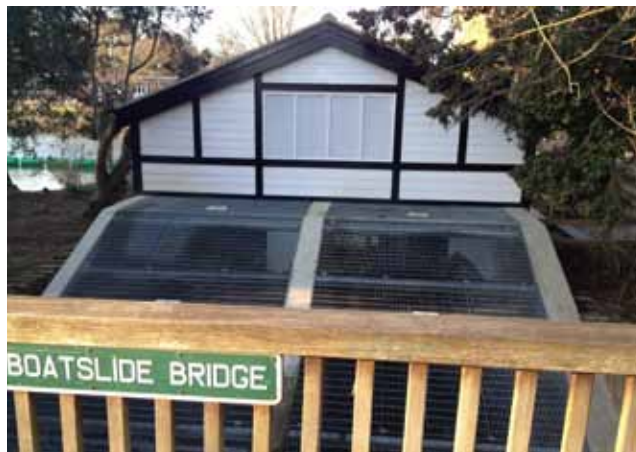
A boat slide on the Great Ouse river. Photos show before the scheme was installed, and after with the turbine building and the two 20kW Archimedes screw turbines underneath a protective grille. (Photo courtesy of Matthew Edgeworth)
