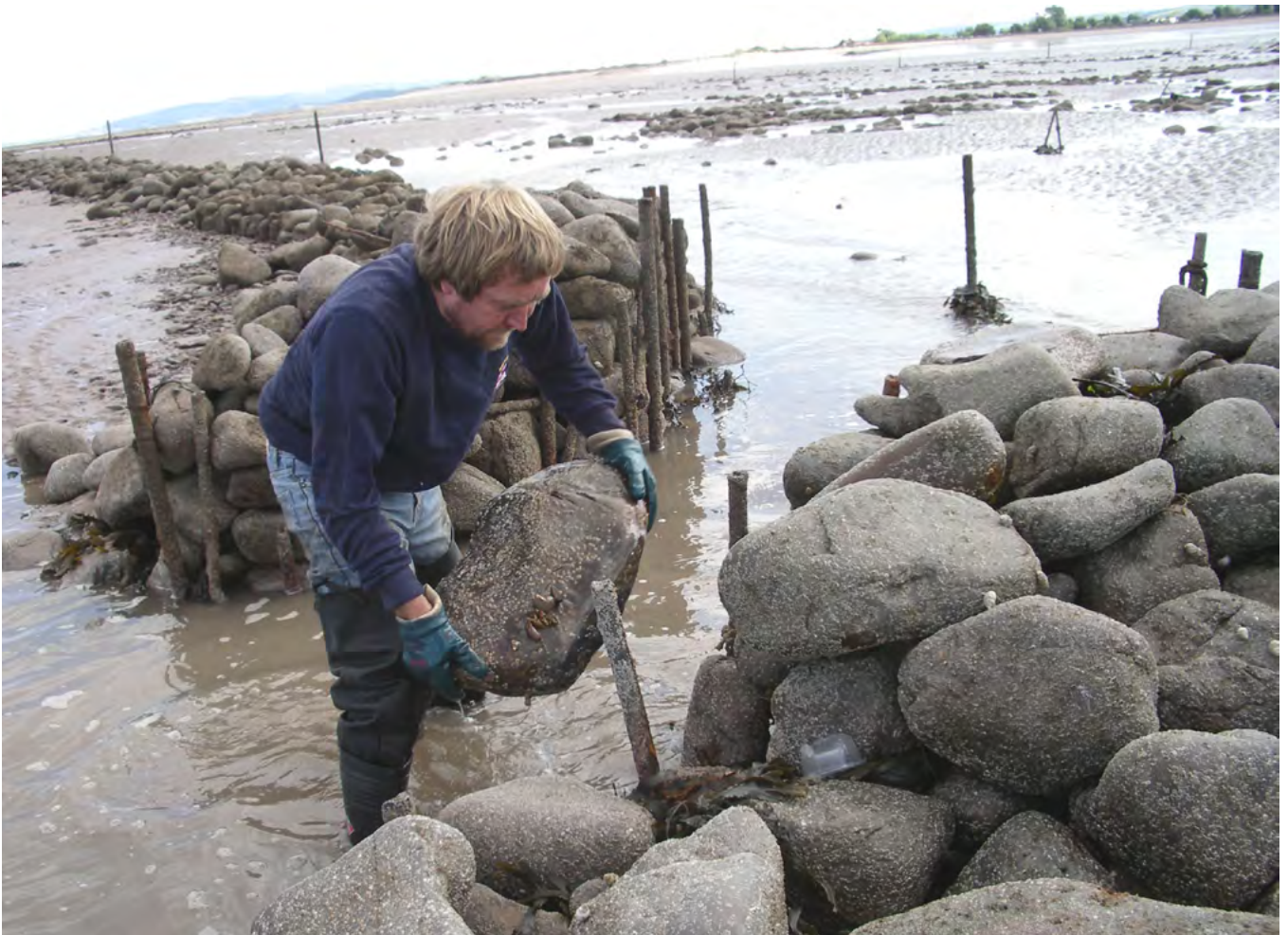
Figure 7 Some of the stone-built weirs in Minehead Bay, Somerset, are still in use and need constant maintenance.
