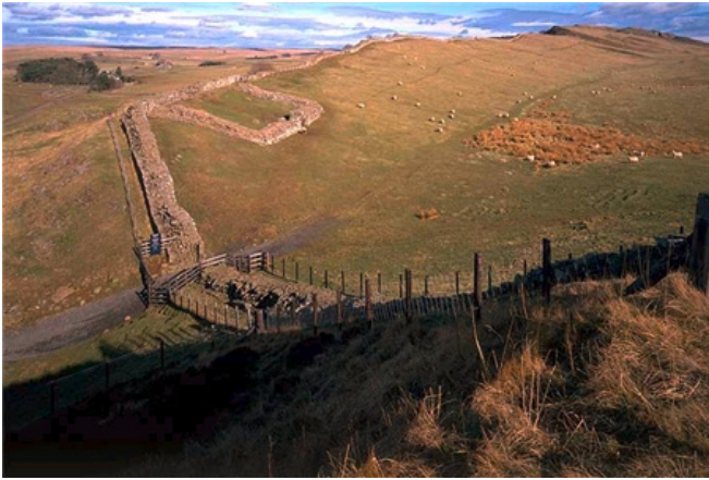
Figure 5 The Stone Wall and milecastle 38 (Cawfields) from the west.
