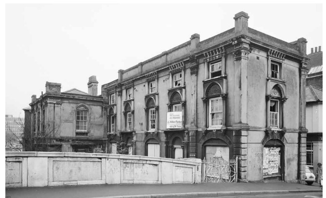
Figure 10 The exterior of the former Coroner's Court. Reading, Berkshire. This coroner's court was adapted from a police court building of 1862, a building built in a 'Venetian Gothic' style mixing gothic and classical forms. Listed Grade II.
