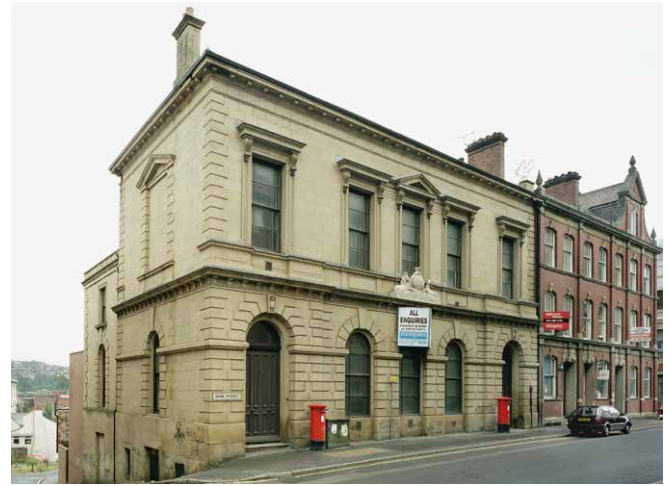
Figure 5 The exterior of the former County Court in Sheffield, South Yorkshire, 1851-4, Charles Reeves. Another of the designs by the prolific Reeves, it was innovative as the courtroom was located on the first floor, allowing the ground floor to be used for office space. Listed Grade II.
