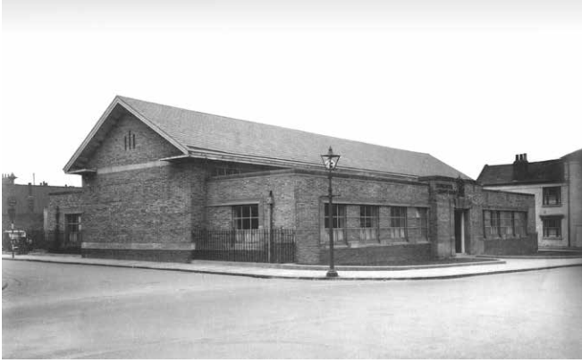
Figure 8 The exterior of Doncaster County Court, 1935-6. From the inter-war years County Court designs followed contemporary architectural tastes and by the late 20th century were often located in modern office buildings.
