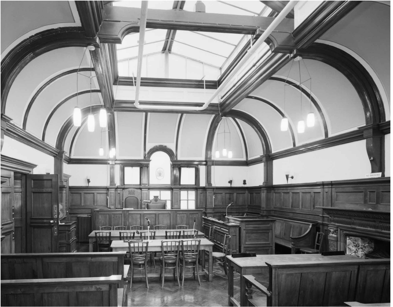
Figure 15 Interior of courtroom, Westminster Coroner's Court, Horseferry Road, Westminster, Greater London, 1893 by G.R.W. Wheeler. This first-floor court is located in the
