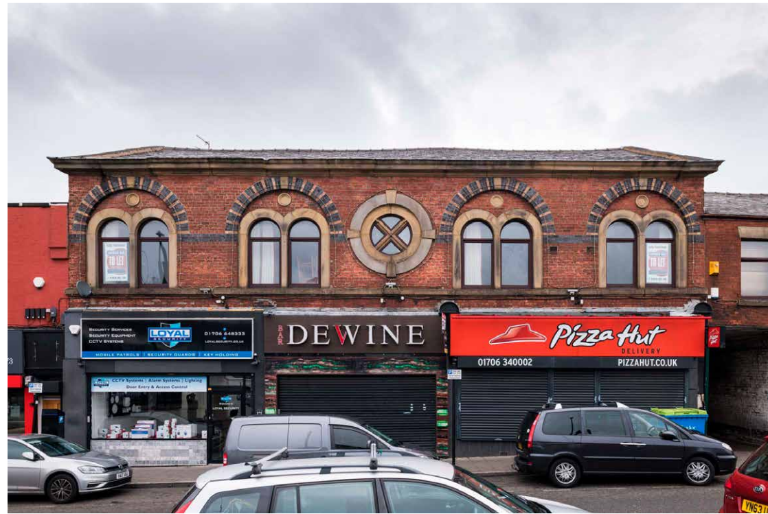
Above right: 7-11 Oldham Road of 1864-5 is the earliest surviving purpose-built co-operative branch store in Rochdale. © Historic England Archive, Steven Baker, DP235562
