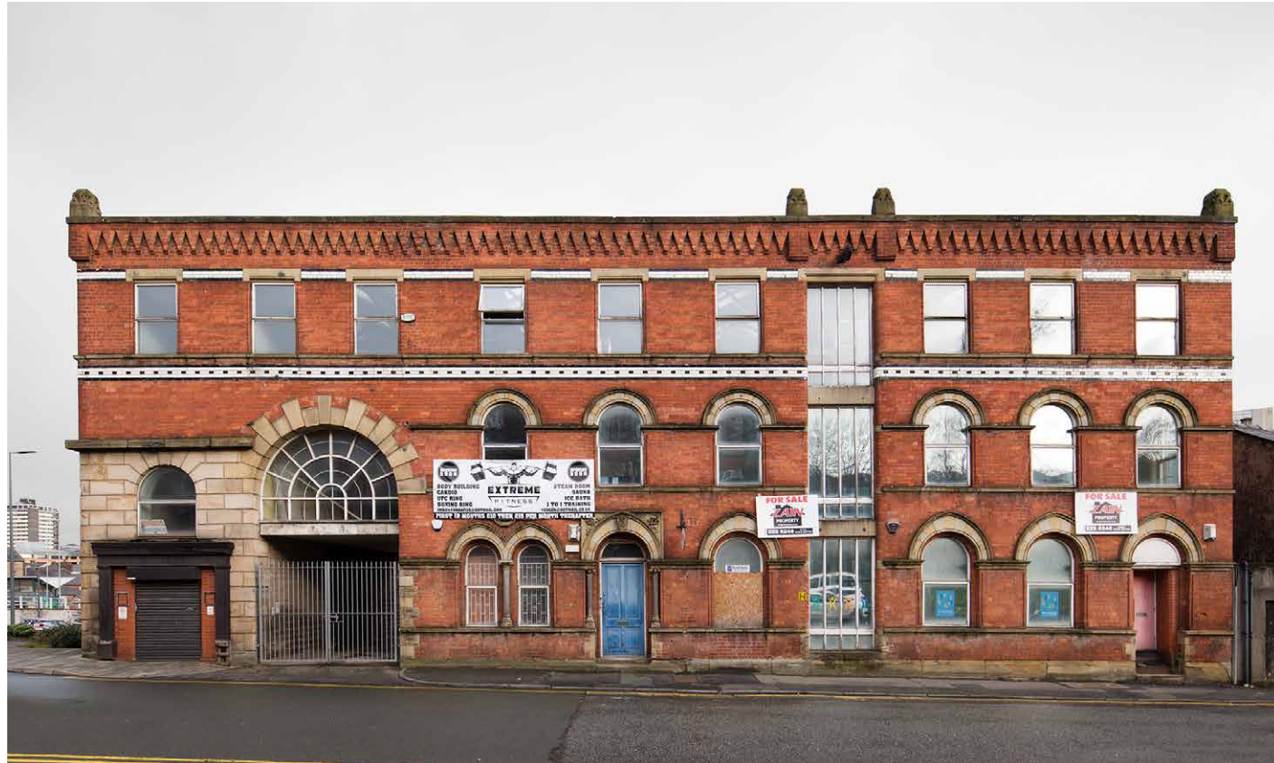
Above: The remains of Water Street Mill, an early steam-powered woollen mill, include an engine house of the 1820s (far left). © Historic England Archive, James O. Davies, DP221867
