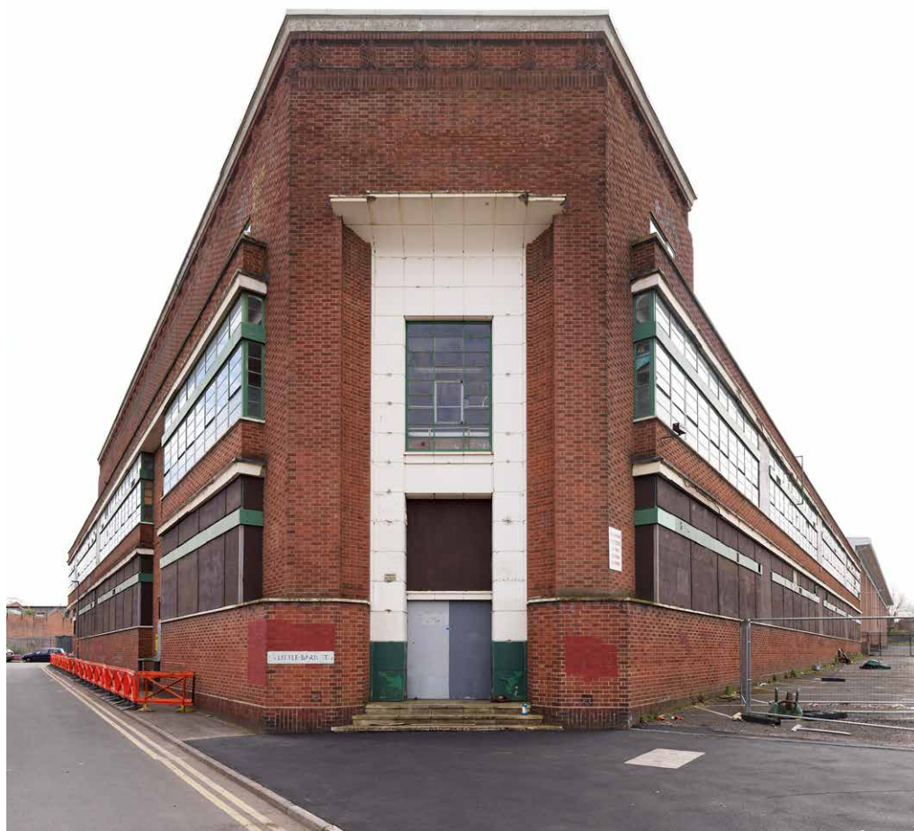
Above: The former Argyle Works in Great Barr Street, an unlisted factory built between 1937 and 1952, has been used as a performance venue by Birmingham Opera. © Historic England, James O Davies, DP196448
