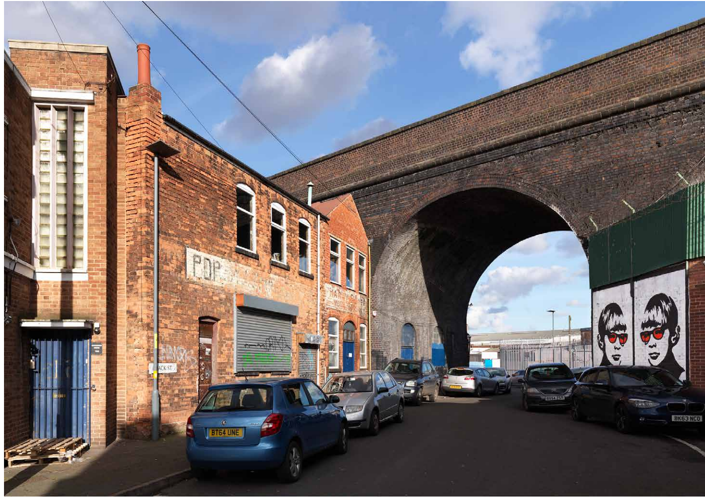
Above: Duddeston Viaduct seen from Hack Street. © Historic England, James O Davies, DP195887
