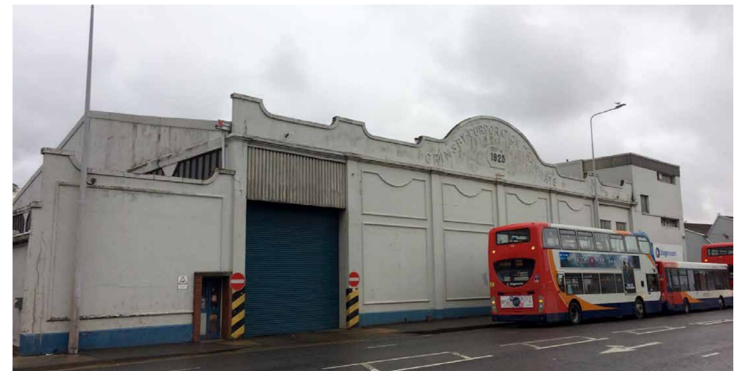
Above right: Grimsby Bus Depot, built out of former RNAS side-opening hangers from the nearby RNAS Killingholme. © Dr Antony Firth
