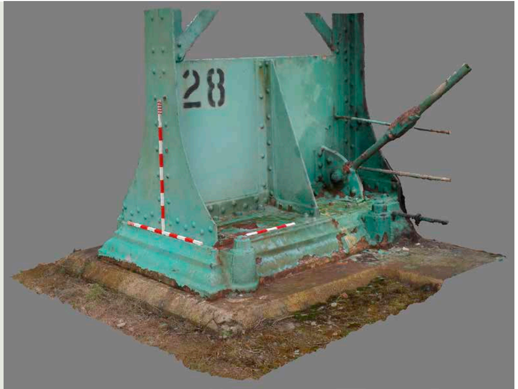
Figure 12: Structure-from-Motion photogrammetry has proved to be a highly effective way of recording in detail structural elements of redundant gasholders. This wrought iron standard base was recorded at the Washwood Heath works, Birmingham. © Museum of London Archaeology.
