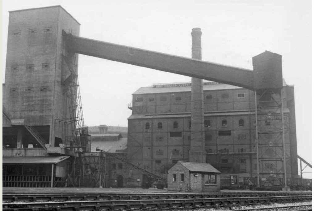
Figure 2: No. 1 retort house at Basford gasworks in 1950. Built between 1854 and 1857 by the Nottingham Gas Light and Coke Co., the works were extended after they were acquired by the municipality in 1874. In 1883, a large horizontal retort house was constructed on the work's southern extension which was later reconfigured to accommodate Woodhall-Duckham vertical retort ovens. The photograph shows the vertical retort house (right) and the earlier horizontal retort house (left, background). The conveyor provided the retorts with a continuous feed of fossil fuel. No vertical retort houses are believed to be extant in England. © National Gas Archive, National Grid.
