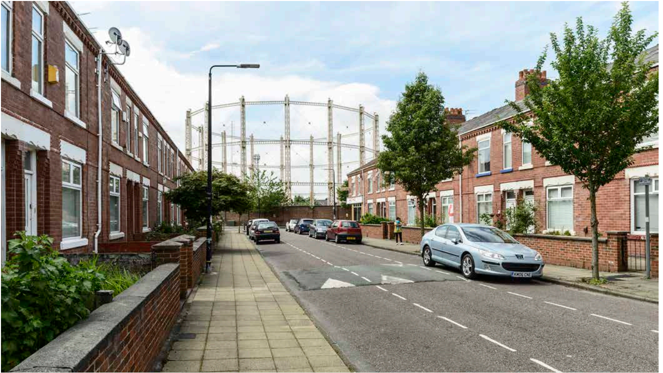
Figure 9: Attention should also be paid to recording the setting and context of the gas works and in particular the gasholders and their dominant position within the skyline and townscape. This view, looking north along Norway Street in Manchester past rows of terraced houses, records the Thomas Street gasholder's place within its wider landscape context. [DP186271]
