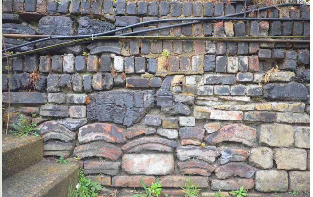
Figure 7: Ex Situ remnants of an early retort house reused in a boundary wall at the Imperial Gas Light and Coke Company works, Fulham. © Matthew Bristow.
