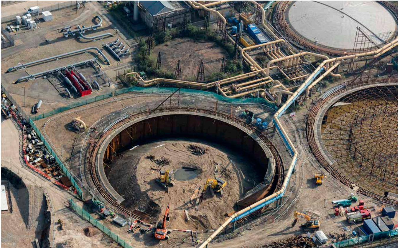
Figure 1: The former Imperial Gas Light and Coke Company gasworks, Sands End, Fulham, during the demolition and remediation of the gasholder station in 2017. The gas holder to the right has had its crown removed, revealing the radial trusses which supported the crown when the holder was in an unpressurised state. The gas holder in the centre of the view has had its trusses removed, exposing the ‘dumpling’ (the cone of earth in the centre of an in-ground gasholder tank) which is in the process of being excavated to remove the source of contamination. The small gasholder at the top of the image was constructed in 1829-30 and is Grade II* listed. [33093_012]
