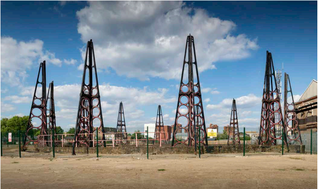
Figure 3: Gasholder number 2 at the Imperial Gas Light and Coke Company gasworks, Sands End, Fulham. Constructed in 1829-30, it was, at that time the largest gasholder in the world. A Type 20 holder according to Malcolm Tucker's typology, it is now the only known example of that type in the world. [DP262679]
