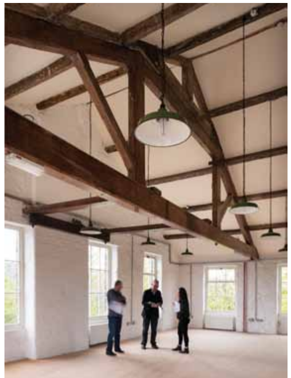
Lomeshaye Bridge Mill is an example of community involvement and third sector occupancy of commercial floor space
