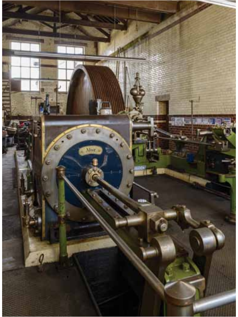
Above: The original Edwardian steam power plant is a rare feature of great interest
