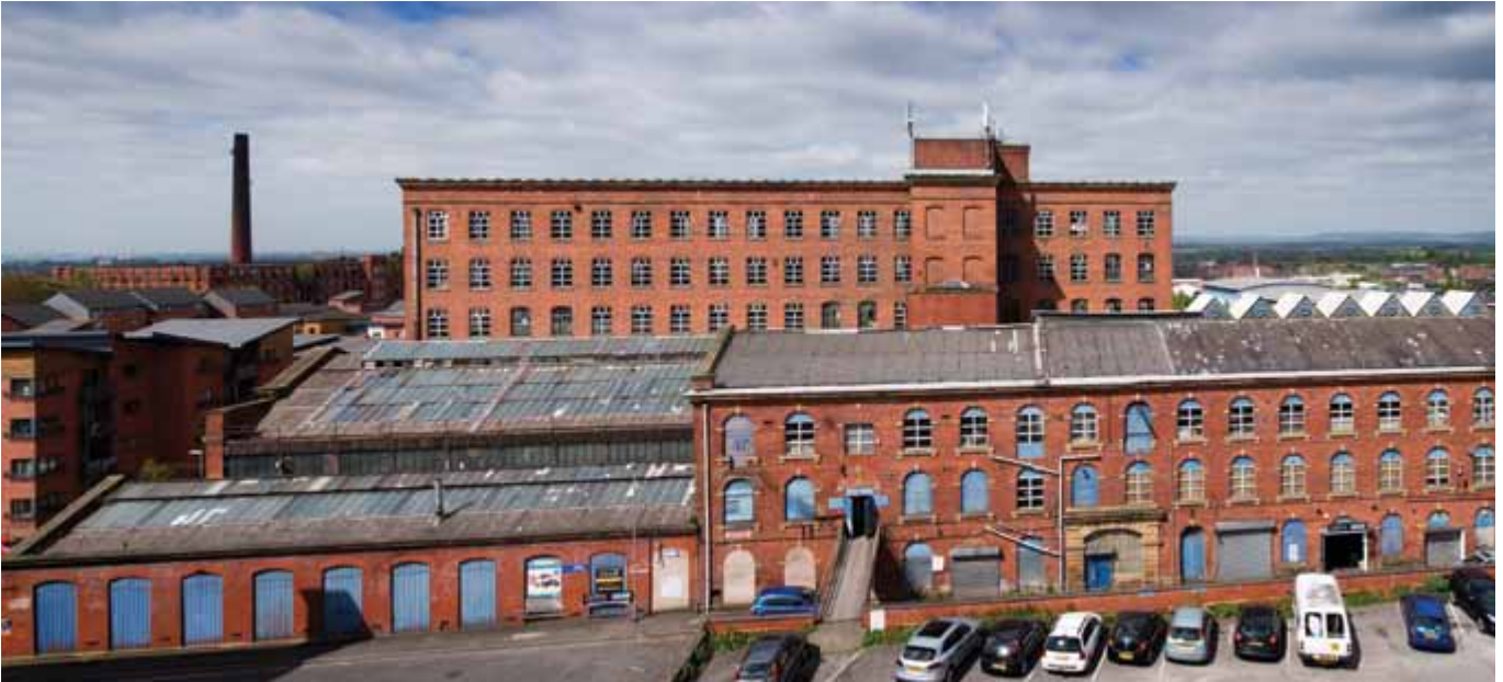
Hartford Works cotton mill dates to 1850, with workshops and offices built in c.1870 and 1883
