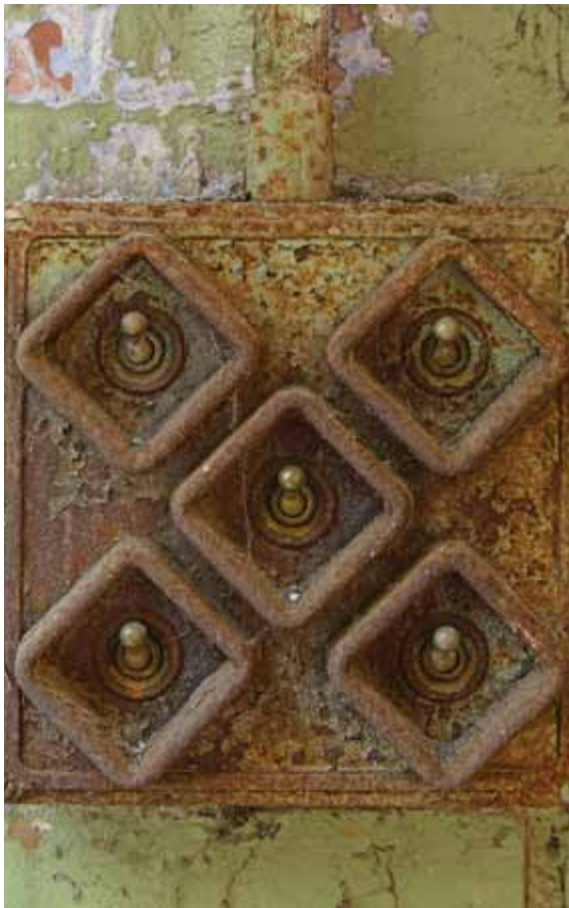
Left and right: Typical detailing within historic mill buildings
