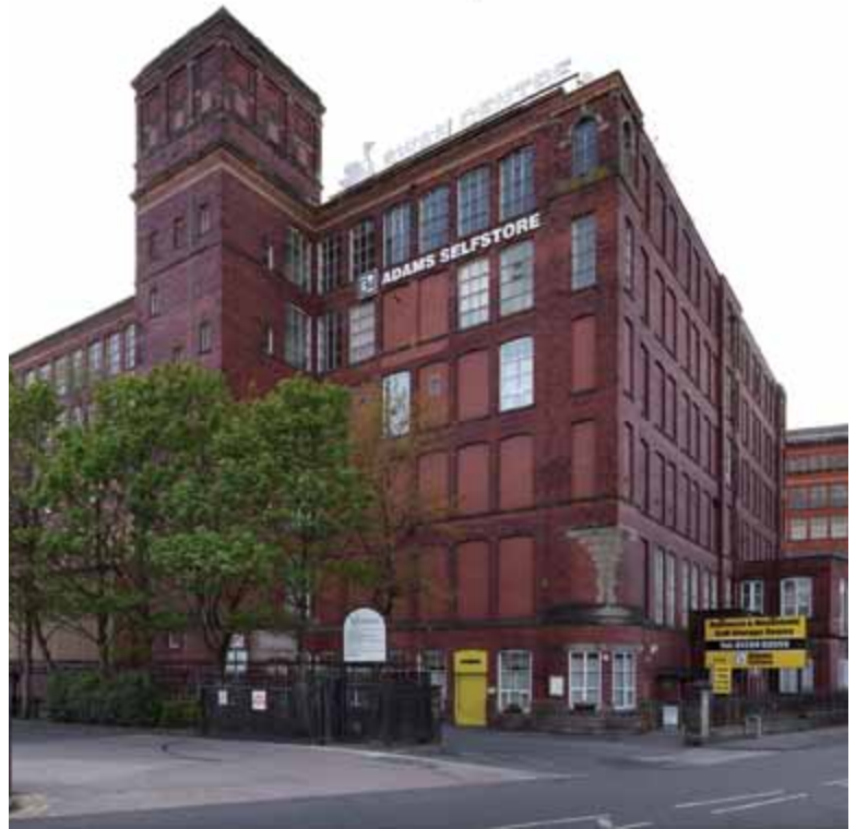
The Swan Lane Mill complex includes a range of commercial uses from storage space to liquorice manufacture
