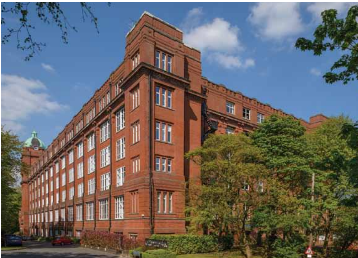
The Cotton Works, Bolton illustrates how former textile mills can be adapted for residential use
