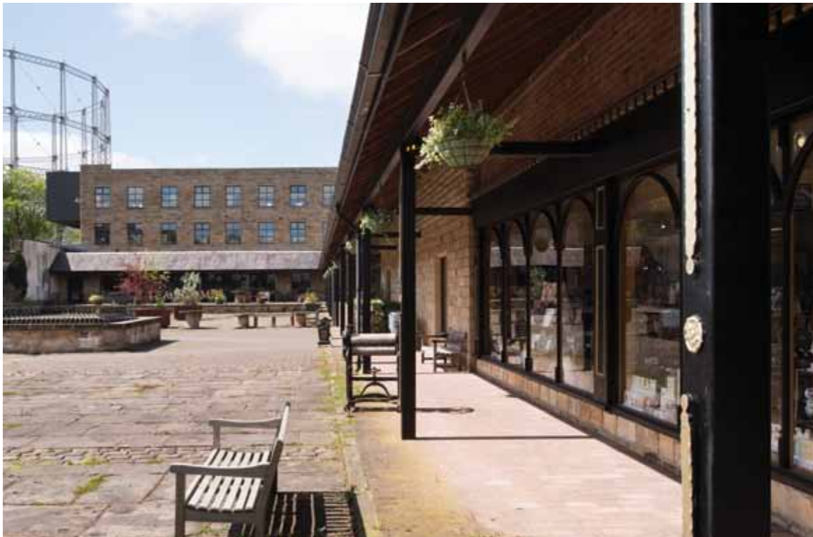
Pendle Village Mill has been refurbished into a successful retail destination
