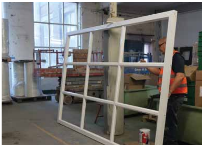
Each window at Tower Works is carefully restored
