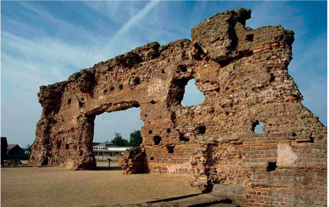
Figure 1 The 'Old Work', Wroxeter, Shropshire. This Roman wall formed part of the entrance from the exercise hall
