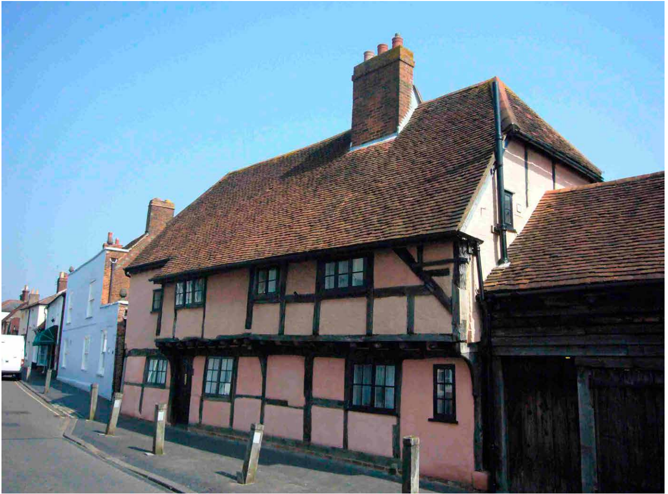
Figure 11 28-30 South Street, Titchfield, Hampshire (listed Grade II*), a jettied urban house set parallel to the
