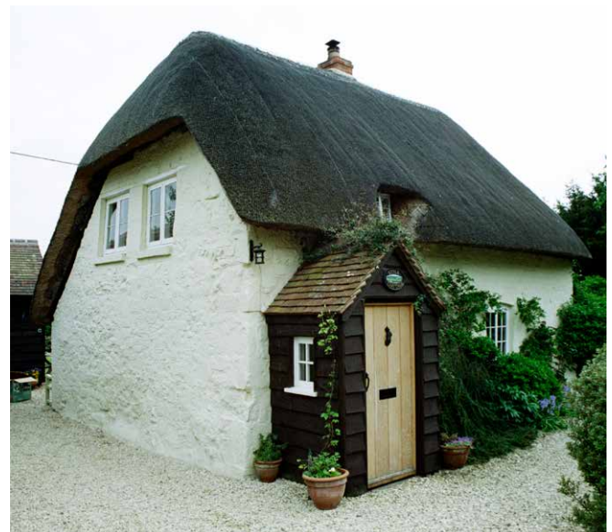
Figure 2 Style Cottage, Uffington, Oxfordshire (listed Grade II), one of the oldest labourer's cottages in Oxfordshire. The left side of this chalk-block cottage was built as a one-up one-down dwelling before 1699; a second one-up one-down was built against it between 1705 and 1766. About 1900 the two were knocked together.
