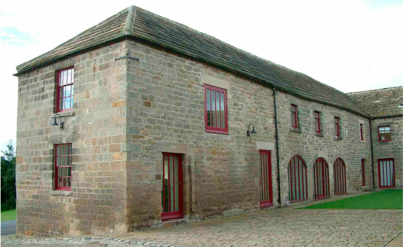
Figure 16 Stocksfield Farm, Hexham, Tynedale. A nineteenth-century planned farmstead successfully converted to multiple business uses. Listed Grade II.
