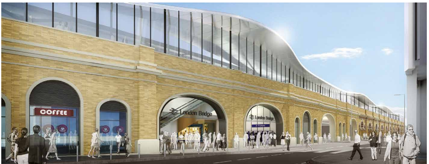
London Bridge station is currently undergoing massive reconfiguration at the historic heart of the city and Borough integrating a Victorian main station into a 21st Century transport hub whilst enlivening the surrounding area.
