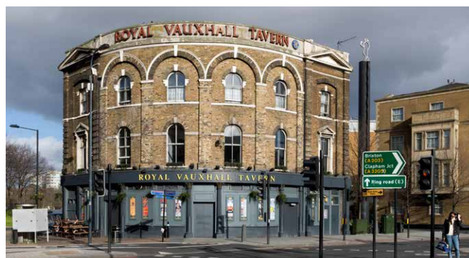
Royal Vauxhall Tavern, London. The Royal Vauxhall Tavern was listed at Grade II in 2015 as part of Historic England's ongoing research into LGBT heritage © Historic England
