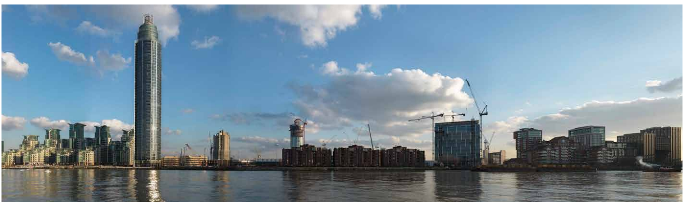
New residential development under construction at Vauxhall and Nine Elms, one of London's Opportunity Areas. © Historic England
