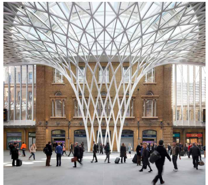
King's Cross Western Concourse has opened up the front of the station, as the original architect intended in 1852, and created a major new public area. © Hufton and Crow
