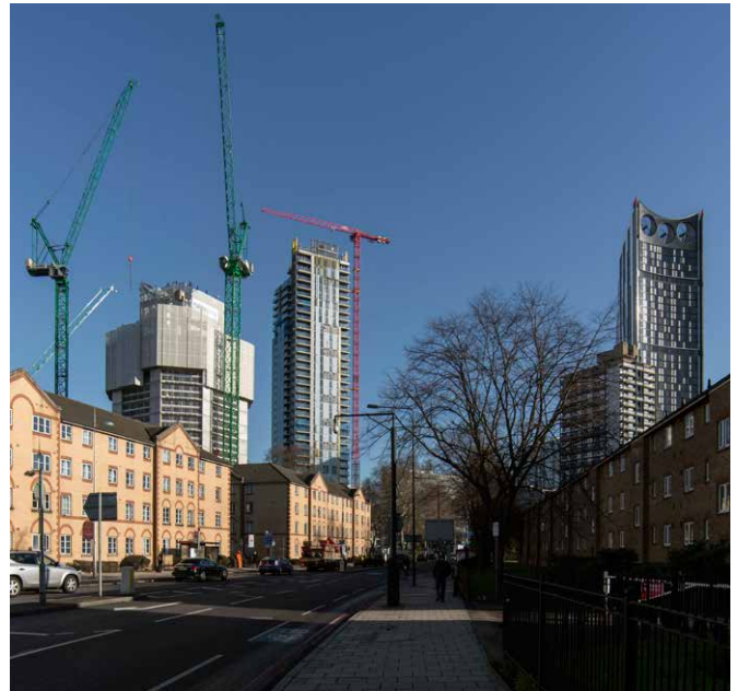
New tall buildings under construction at Elephant & Castle. © Historic England
