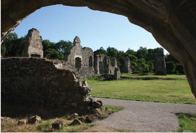
Theft of supporting arches caused considerable damage to the masonry at Grace Dieu Priory, near Loughborough.
