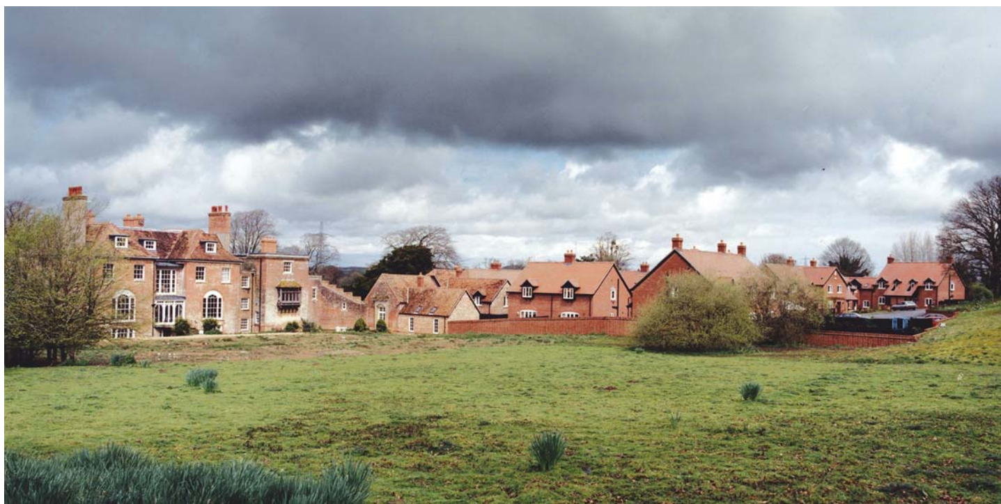
Henbury House, Dorset. In 1995 'enabling development' permission was given for the construction of 29 new homes to offset the cost of major structural repairs to this important Grade II* country house. With hindsight, the application of Conservation Principles could have helped identify a solution less damaging to the heritage values of the original building and its setting. © English Heritage
