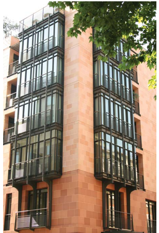
15–25 Davies Street, Mayfair, London: a fine new modern building in terracotta and bronze by KPF.
