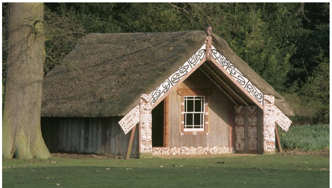
Understanding significance: Hinemihi is a Maori meeting house now located within the grounds of Clandon Park, near Guildford, Surrey. The National Trust has been working with the Maori community on plans for the future care of Hinemihi. © NTPL/Nick Meers
