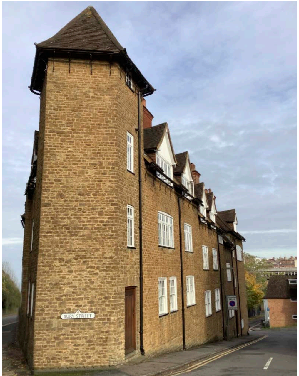
Figure 29: Wycliffe Buildings, Portsmouth Road, Guildford. Bargate Stone.
