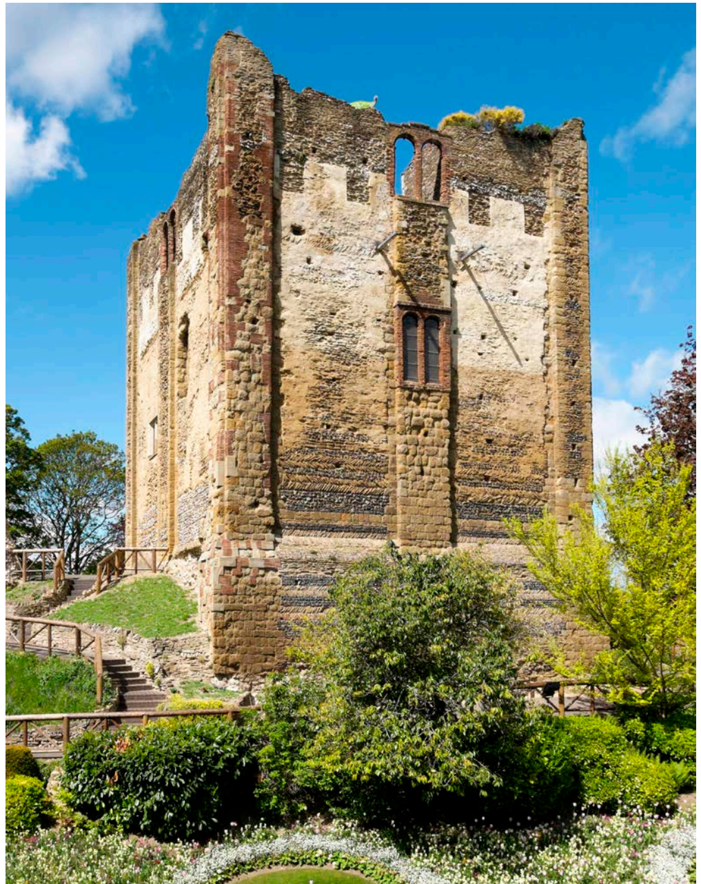
Figure 2: Guildford Castle tower keep. Bargate Stone and Quarry Flint, with chalk and Upper Greensand Sandstone quoins and a chalk plinth. Repairs include Bargate Stone, flint and carstone.
