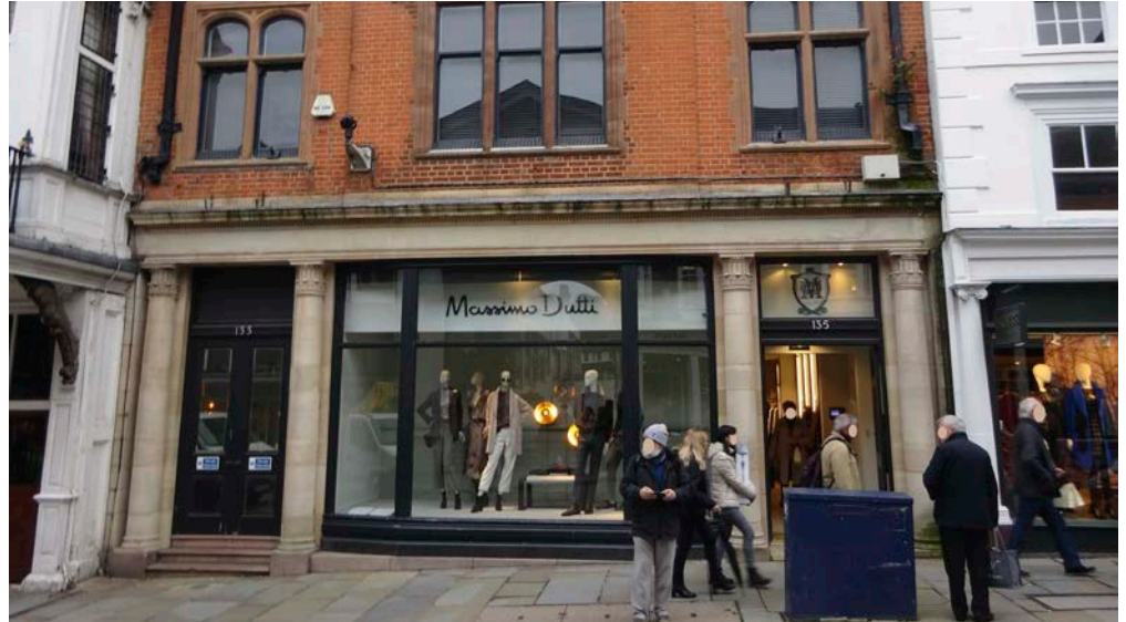
Figure 66: Pillars and surrounds, 133–135 High Street, Guildford. Ancaster Stone. First and second floor window dressings are Permo-Triassic red sandstones, including Hollington Stone.
