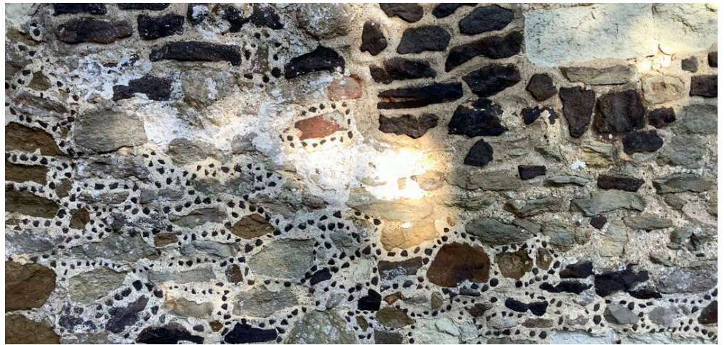
Figure 36: Church of St James, Shere. Ironstone and Upper Greensand Sandstone with ironstone galleting.
