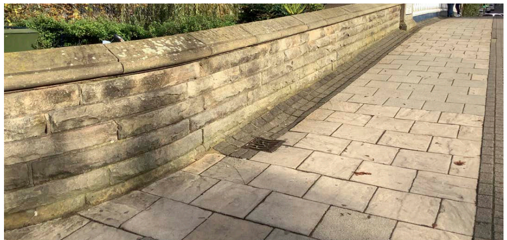
Figure 60: Town Bridge, Guildford. Millstone Grit.
