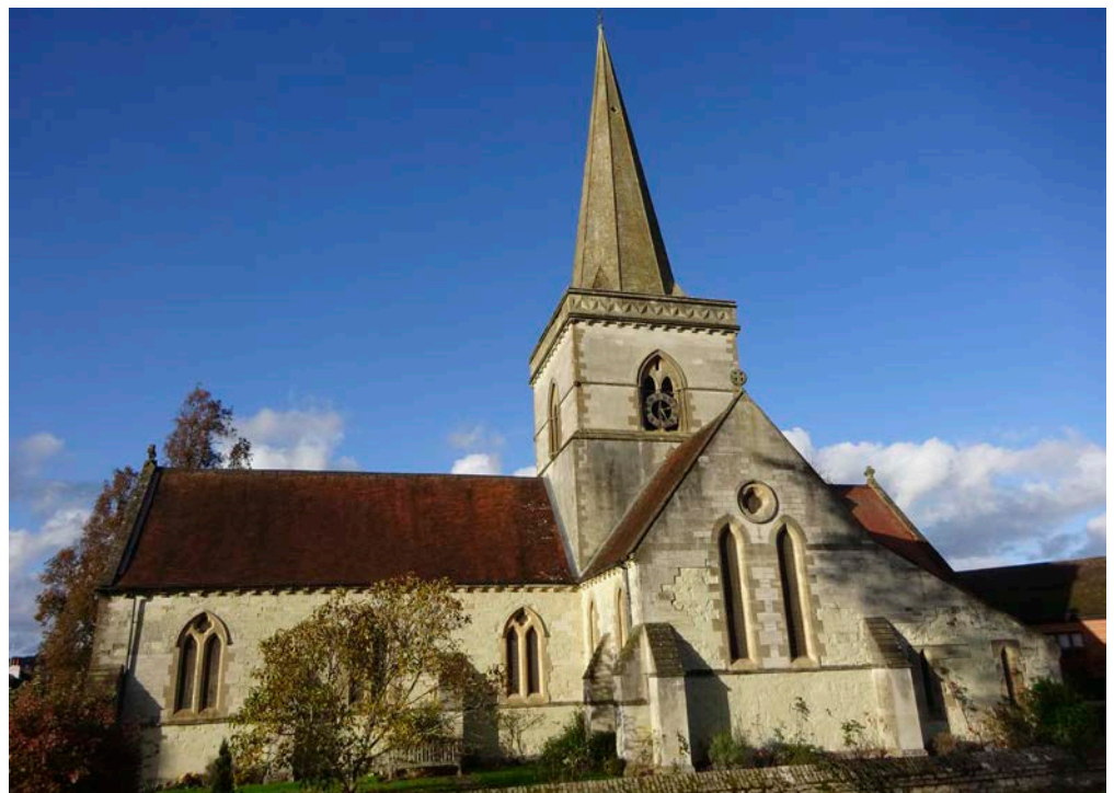
Figure 14: Christ Church, Brockham. Reigate Stone with chalk dressings, much replaced with Bath Stone.
