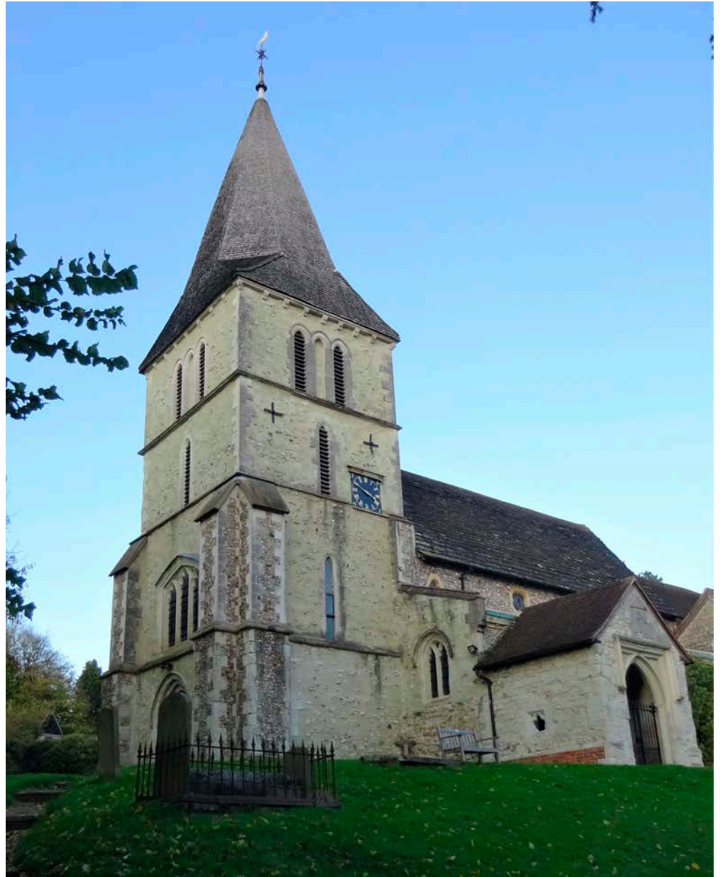
Figure 39: Church of St Katharine, Merstham. Reigate Stone and flint rubble. Horsham Stone slate roof on the nave.
