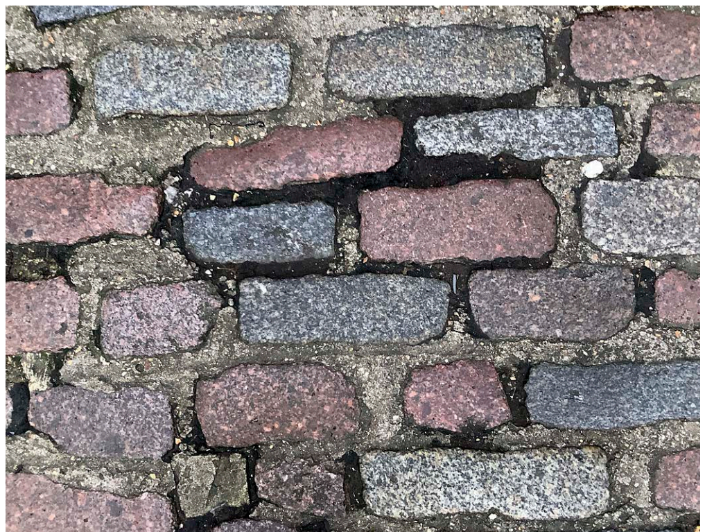
Figure 76: Paving setts outside the Angel Hotel, High Street, Guildford. Granodiorite.
