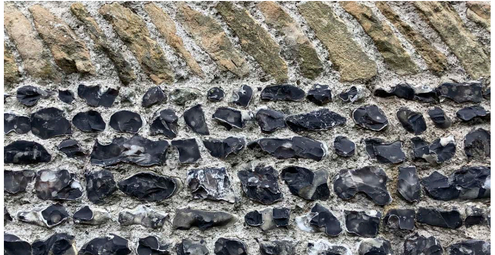
Figure 44: Castle keep walls, Guildford Castle. Quarry Flint and Bargate Stone.
