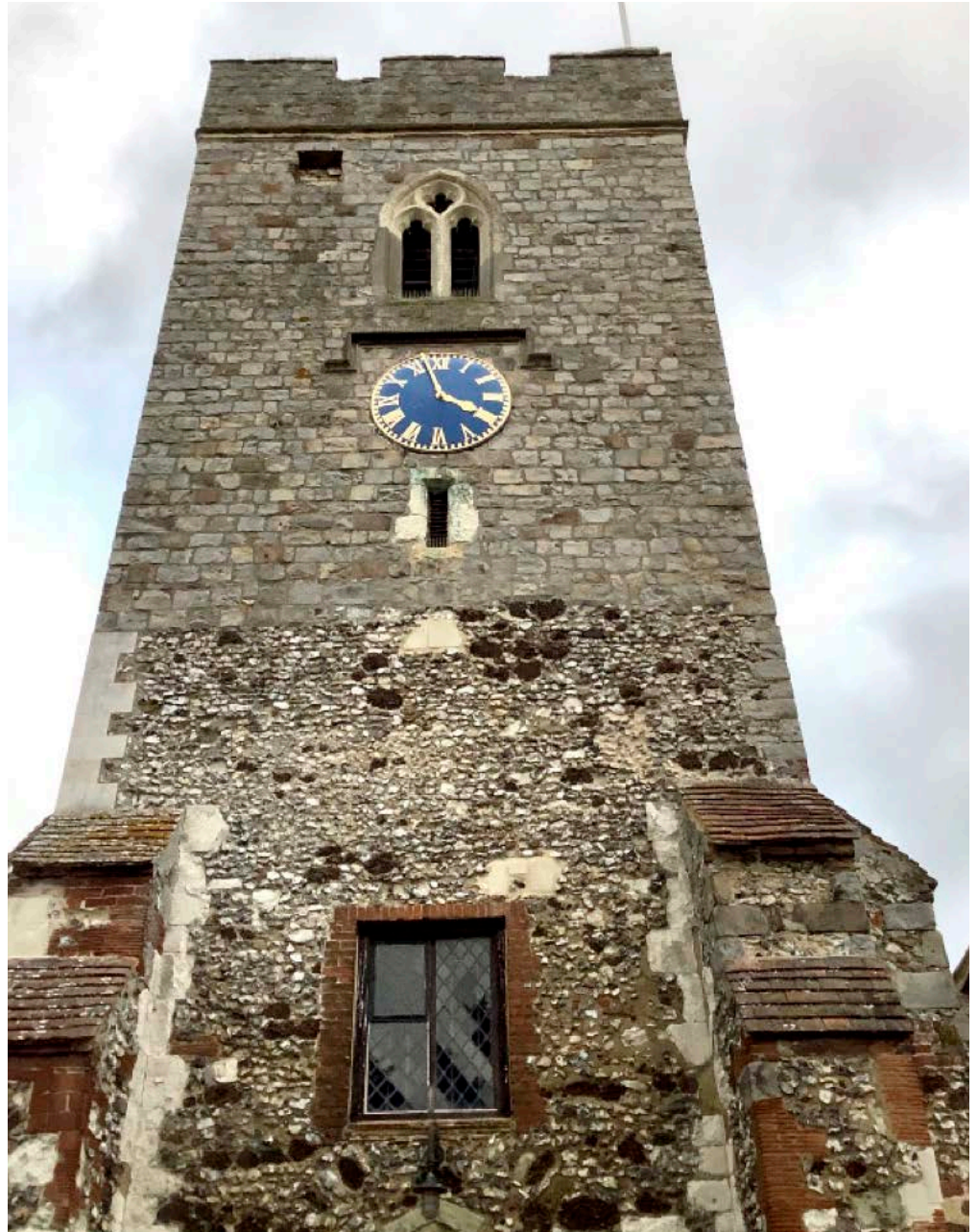
Figure 49: Church of St Peter, Old Woking. Quaternary Flint and ironpan conglomerate. Upper part of the tower is Sarsen stone.
