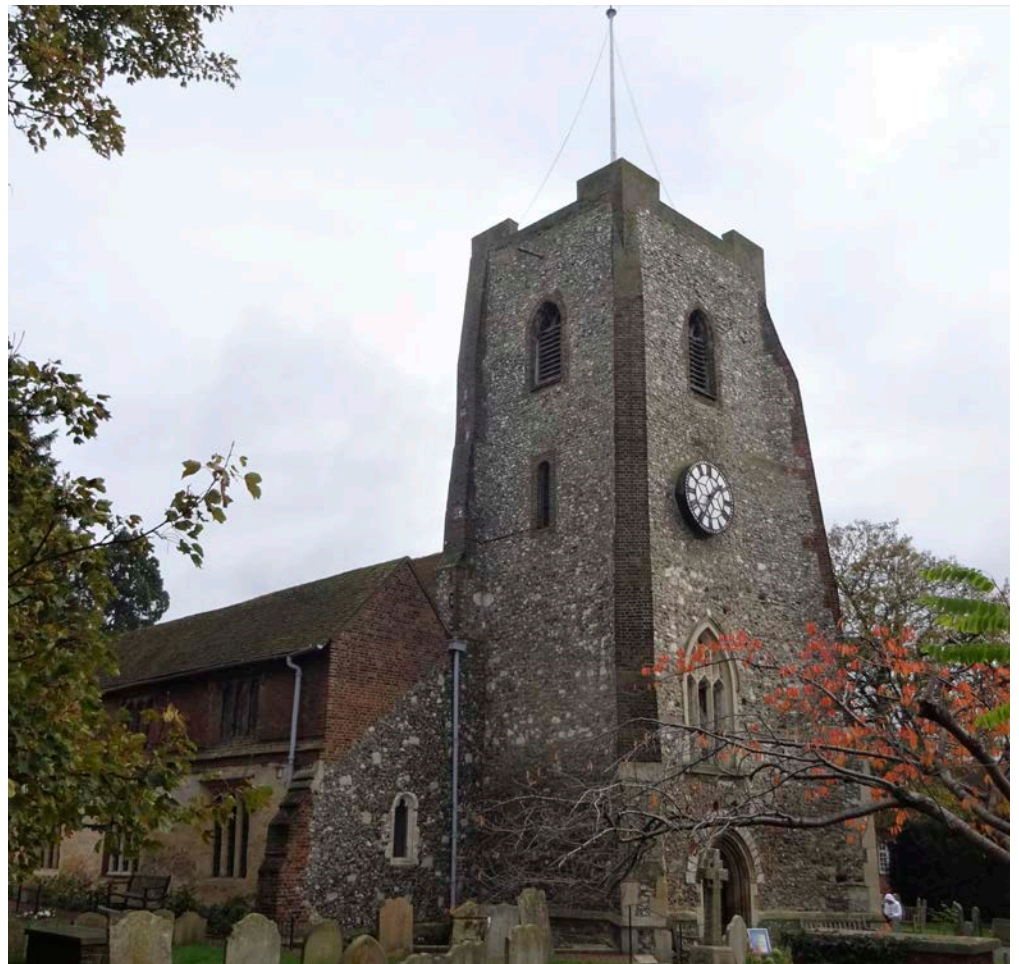
Figure 9: St Mary's Church, Walton-on-Thames. Flint with stone dressings, and a brick clerestory.
