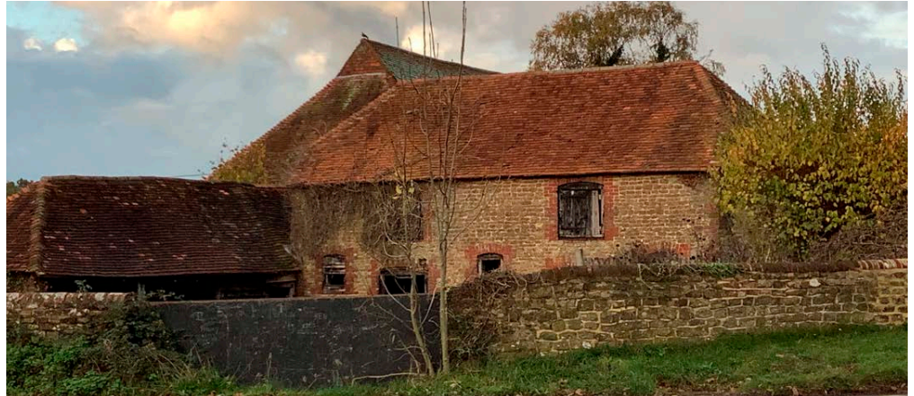
Figure 4: Barns, Hydestile Farm, Hambledon. Bargate Stone with brick dressings.
