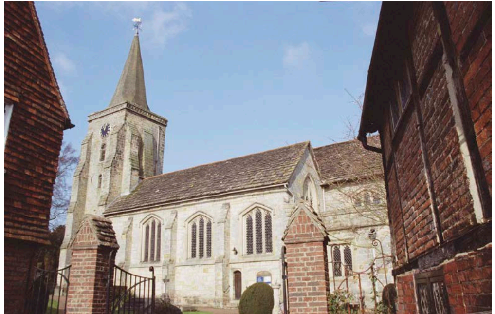
Figure 22: Church of SS Peter and Paul, Lingfield. Tunbridge Wells Sandstone with a Horsham Stone slate roof.
