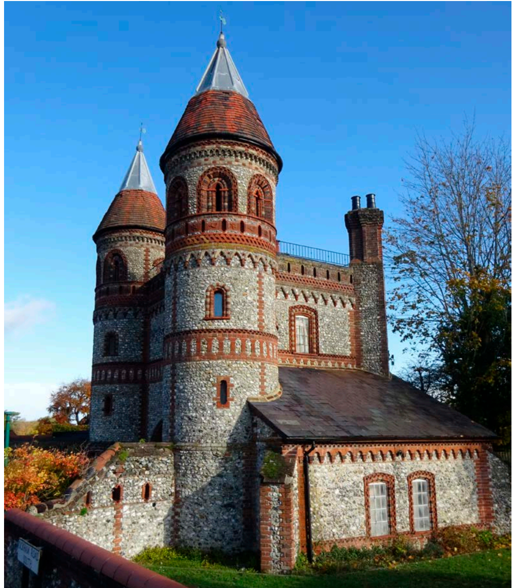
Figure 57: Guildford Lodge and Gate, East Horsley. Quaternary Flint rubble with brick and terracotta dressings.
