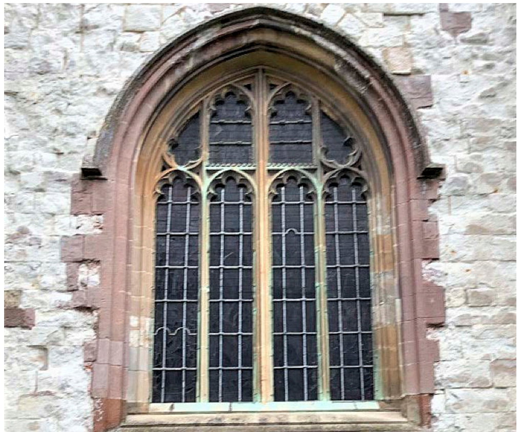
Figure 63: St Andrew's Church, Farnham. Window dressings of Hollington Stone and Bath Stone.
