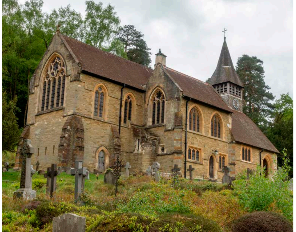
Figure 27: St Mary the Virgin Church, Holmbury St Mary. Holmbury Hill Sandstone with Bath Stone dressings.
