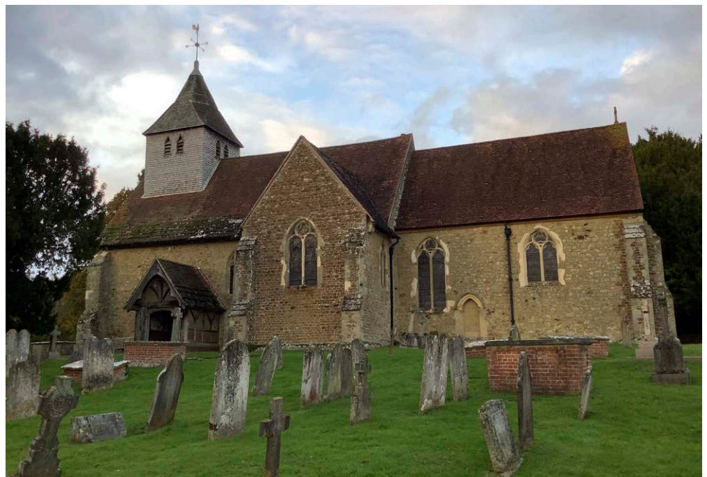
Figure 16: Church of St Mary and All Saints, Dunsfold. Bargate Stone with some ironpan conglomerate and Upper Greensand Sandstone and ironstone galleting.
