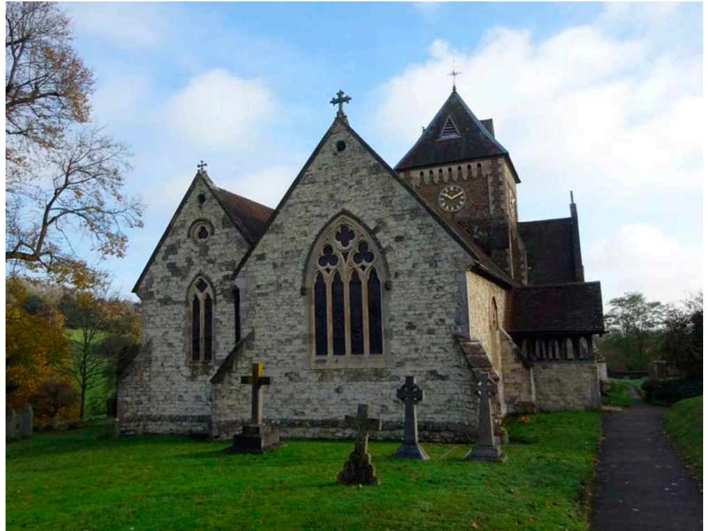
Figure 43: Church of St Laurence, Seale. Upper Greensand Sandstone and chalk; the tower is mainly Bargate Stone with Bath Stone dressings.
