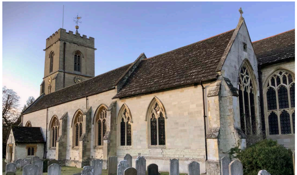
Figure 67: St Mary’s Church, Reigate. Restored using Bath Stone.
