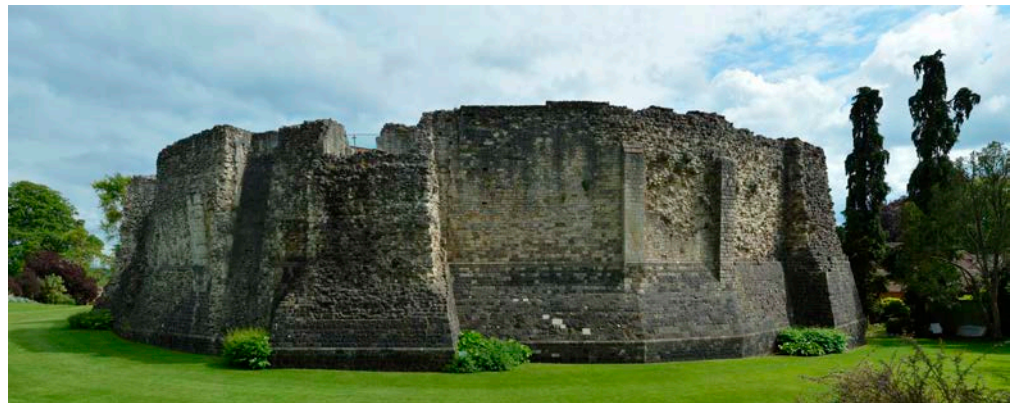
Figure 21: Curtain wall and keep, Farnham Castle. Chalk and Upper Greensand Sandstone.
