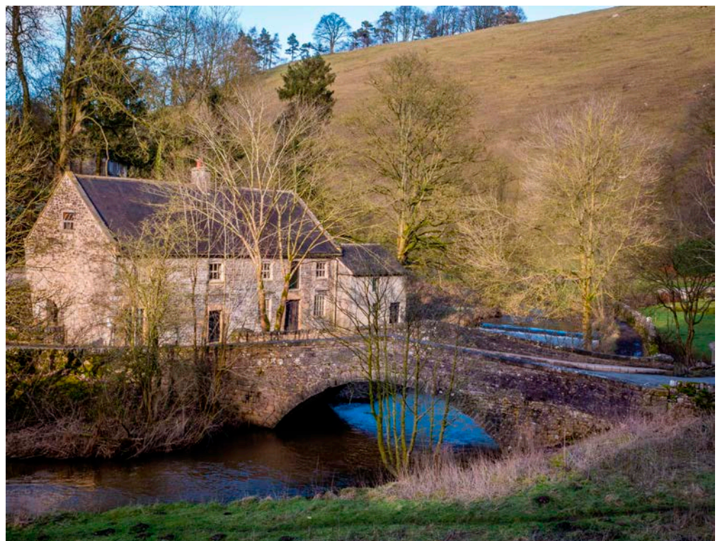
Figure 5: Lode Mill Bridge, Alstonefield. Limestone rubble.
