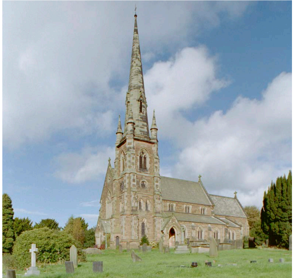
Figure 13: The Church of St John the Baptist, Keele. Butterton and Springpool sandstones.
