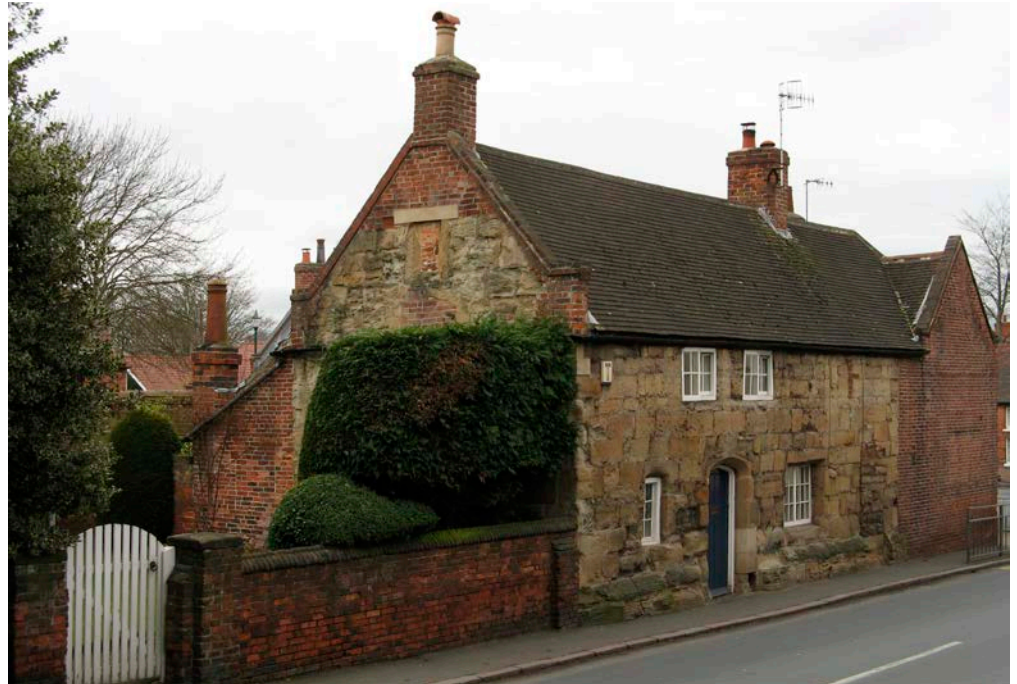
Figure 3: The Chantry, Wollaton. Coal Measures Sandstone.
