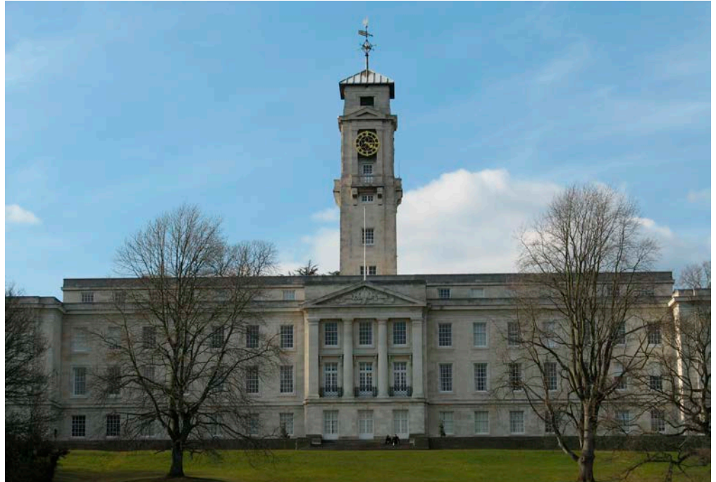
Figure 21: Trent Building, University of Nottingham. Portland Limestone facade.
