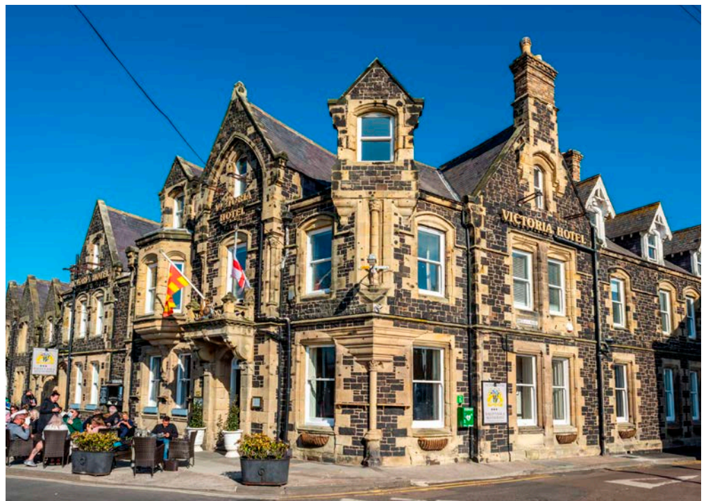
Figure 22: The Victoria Hotel, Bamburgh. Whinstone with Stainmore Formation sandstone dressings and quoins.
