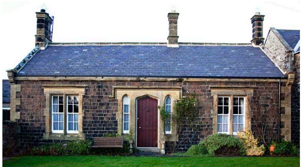
Figure 23: Cottage, Embleton. Whinstone with Stainmore Formation sandstone dressings and quoins.
