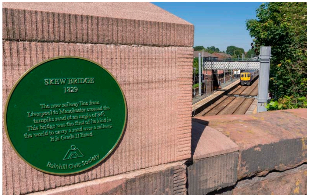
Figure 9: Skew Bridge, Rainhill Station. Rainhill Stone.
