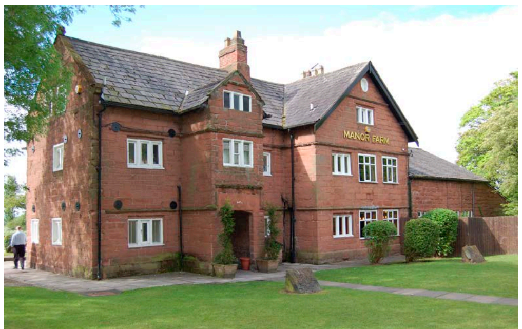
Figure 7: Manor Farm pub, Rainhill. Rainhill Stone.
