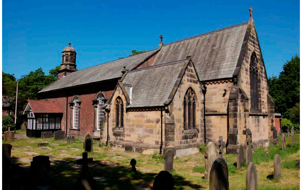
Figure 29: Church of St Peter Apostle and Martyr, Formby. Westmoreland Slate roof.
