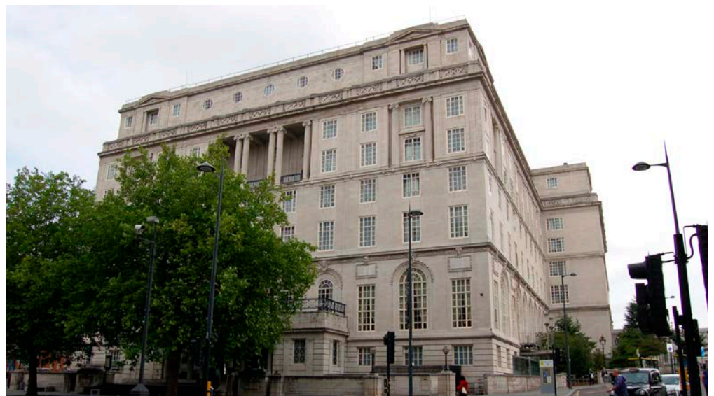
Figure 25: Adelphi Hotel, Liverpool. Portland Stone cladding.
