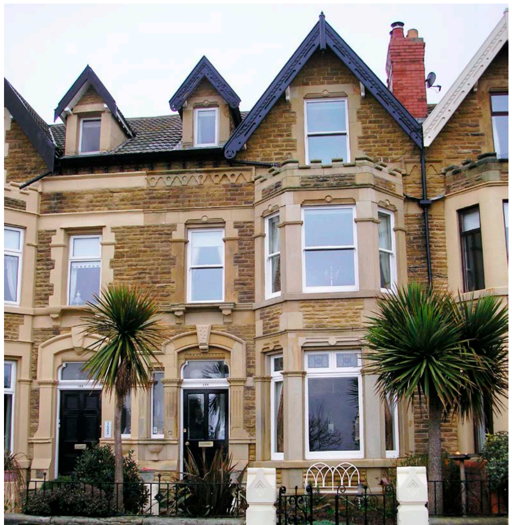
Figure 4: Villa, West Kirby. Milnrow Sandstone.
