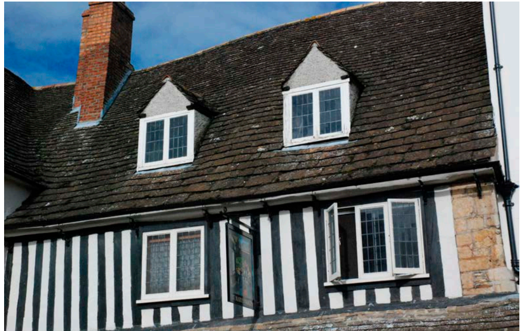
Figure 22: 19 St Mary's Street, Stamford. Collyweston Stone slate roof.
