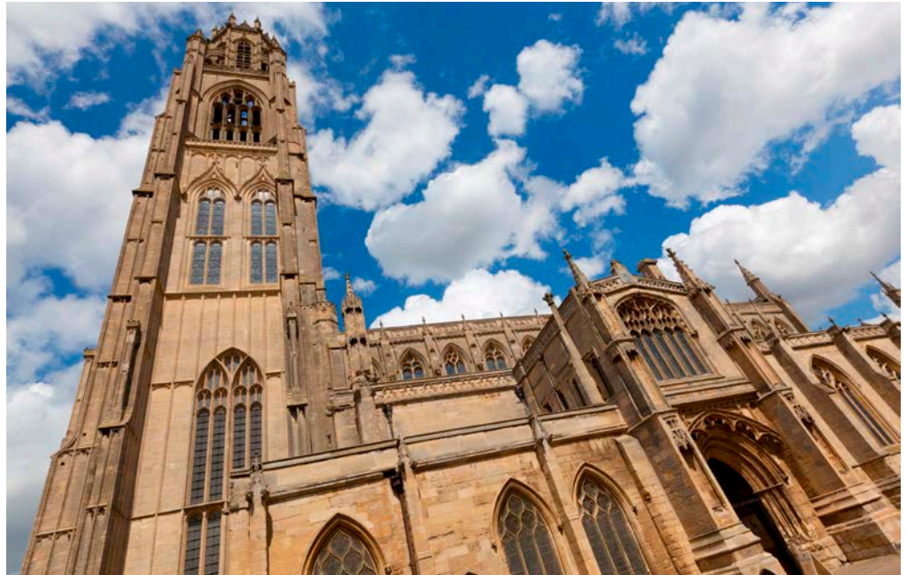
Figure 12: St Botolph's Church, Boston. Lincolnshire Limestone.
