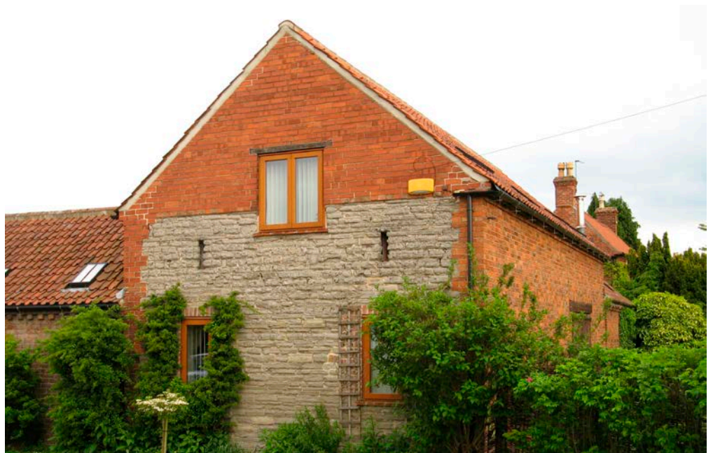
Figure 3: Houses, Main Road, Long Bennington. Blue Lias.
