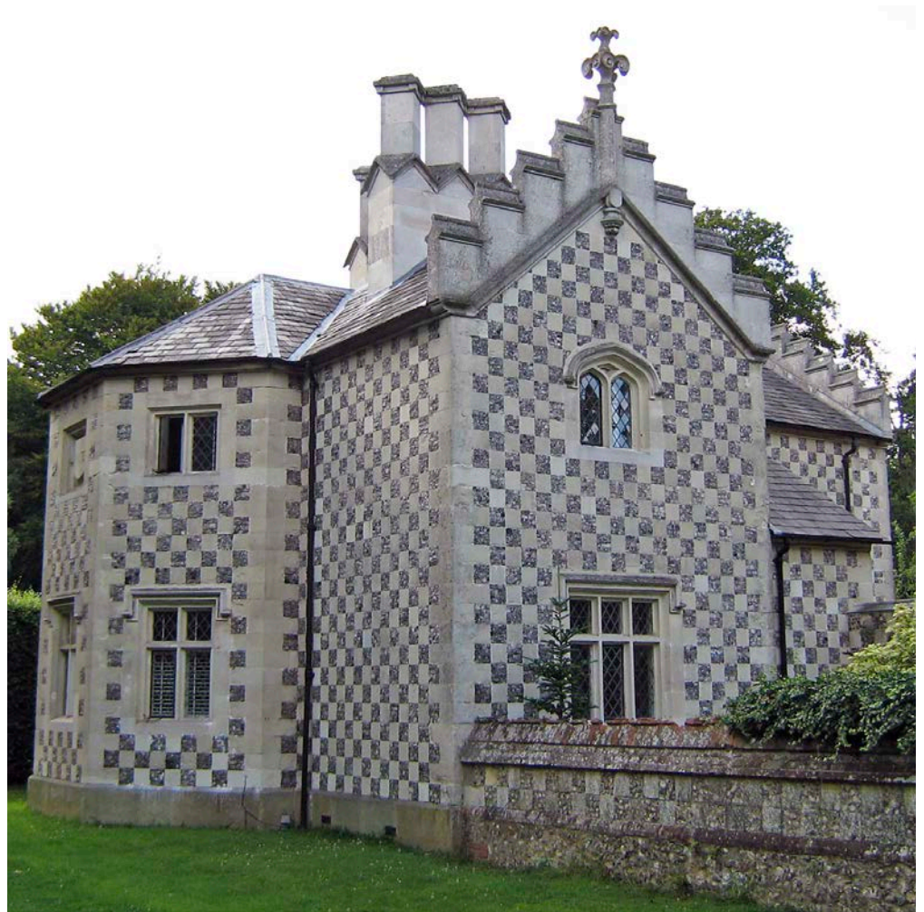
Figure 13: Thunderdell Lodge, Ringshall, near Berkhamsted. Knapped flint and Totternhoe Stone chequerwork.
