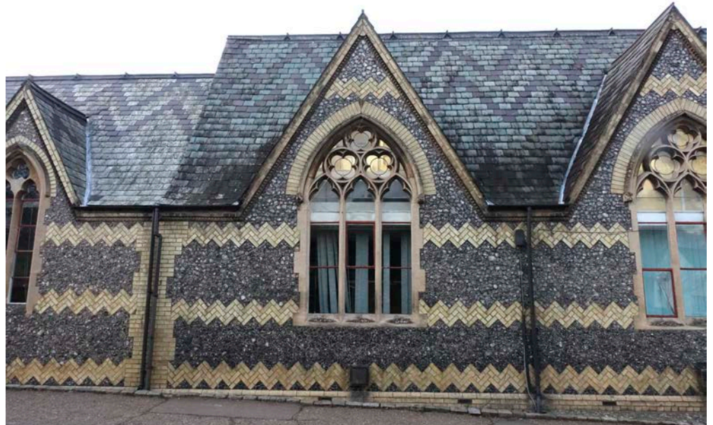
Figure 59: Old School, Church Street, Wheathampstead. Knapped flint with gault brick and Westmorland Slate and Welsh Slate roof.
