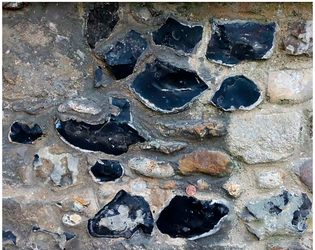
Figure 20: St Mary's Church, Hitchin. Quarry Flint nodules.
