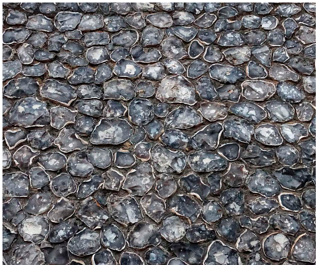
Figure 18: Old School House, Wheathampstead. Knapped flint nodules.
