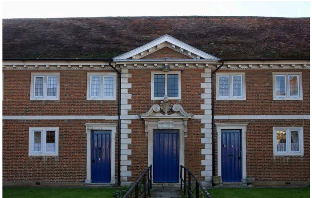
Figure 53: Almshouses, Ward's Hospital, Buntingford. Brick with Portland Stone dressings.
