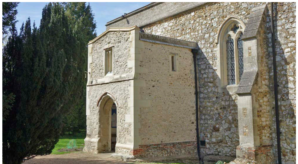
Figure 55: St Mary's Church, Pirton. Flint, with chalk clunch and various limestone and sandstone rubble, including Bedfordshire Greensand.
