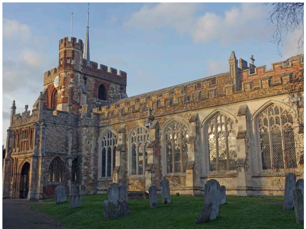
Figure 11: Church of St Mary, Hitchin. Chalk block, Totternhoe Stone, Quarry Flint, Quaternary Flint, glacial pebbles and cobbles and Hitchin Carstone, with Ancaster Stone, Bath Stone and Permo-Triassic sandstone.
