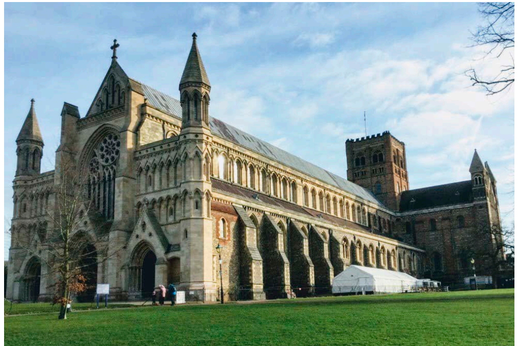
Figure 1: Cathedral and Abbey Church of St Alban, St Albans. Originally flint and Roman brick, rebuilt in Ancaster Stone.
