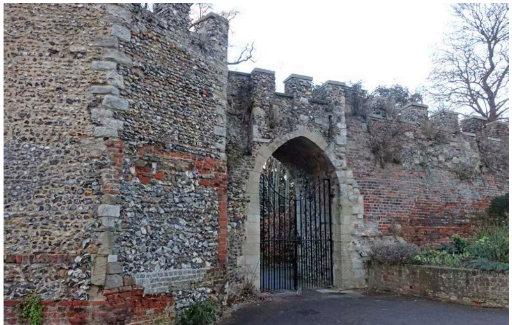
Figure 33: Hertford Castle curtain wall, Hertford. Quaternary Flint and chalk block, with glacial pebbles and cobbles and Quarry Flint nodules. Portland Stone and brick repair work.
