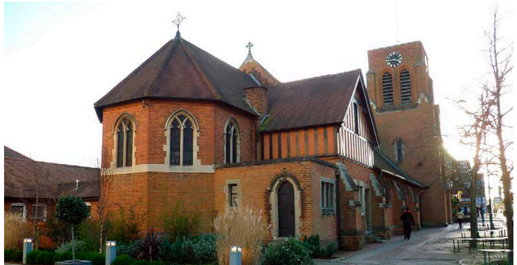
Figure 47: Church of All Saints, Borehamwood. Red brick with Doultong Stone dressings.
