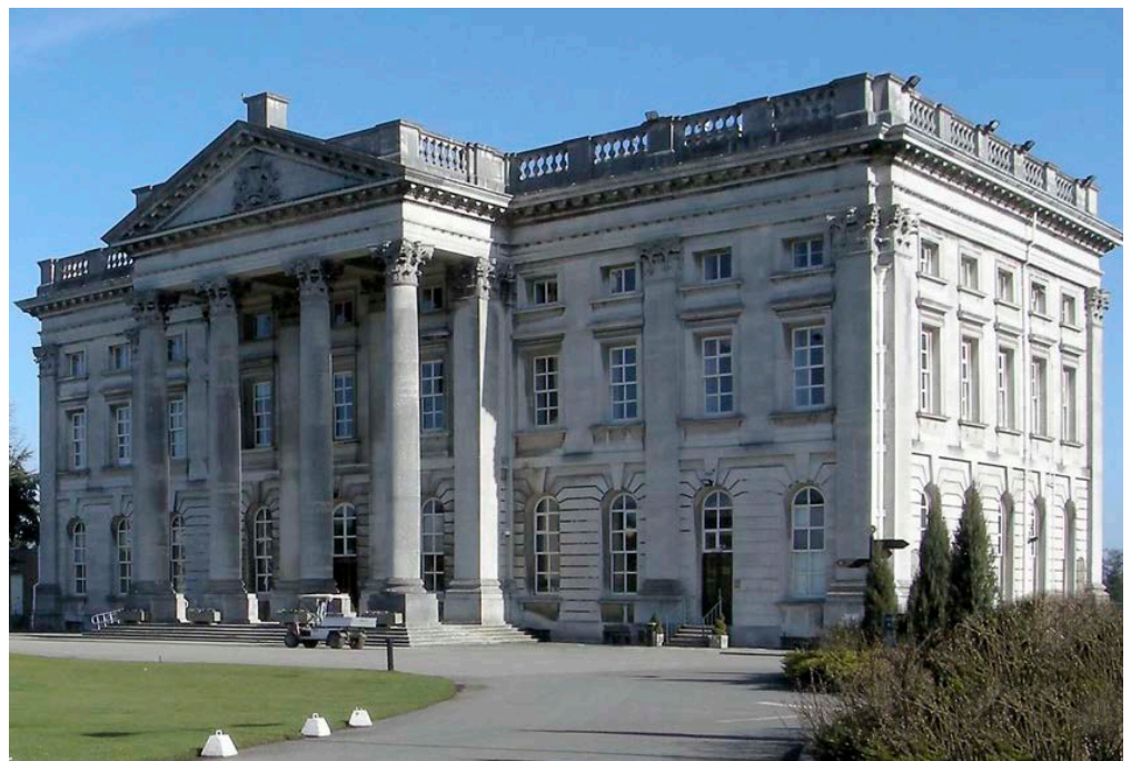
Figure 3: Moor Park, near Rickmansworth. Brick encased in Portland Stone.
