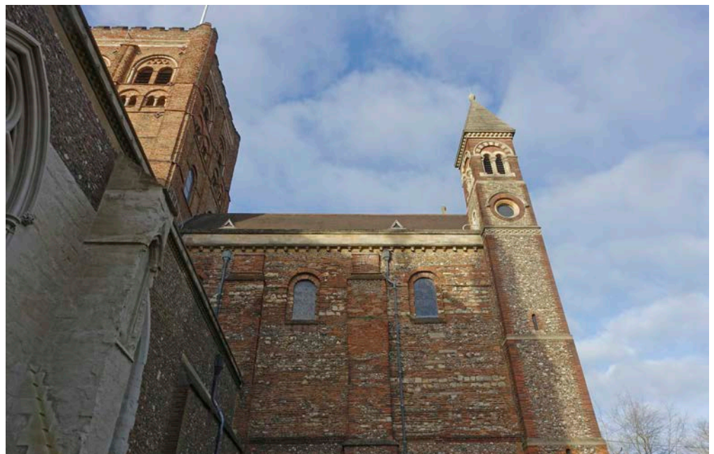
Figure 50: Cathedral north transept and nave, St Albans. Clipsham Stone.
