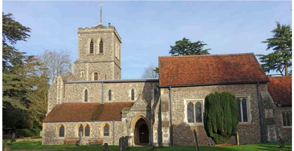
Figure 10: Church of St Michael, St Albans. Flint and Roman tiles with Totternhoe Stone, Hertfordshire Puddingstone, Bath Stone and possibly Ham Hill Stone.
