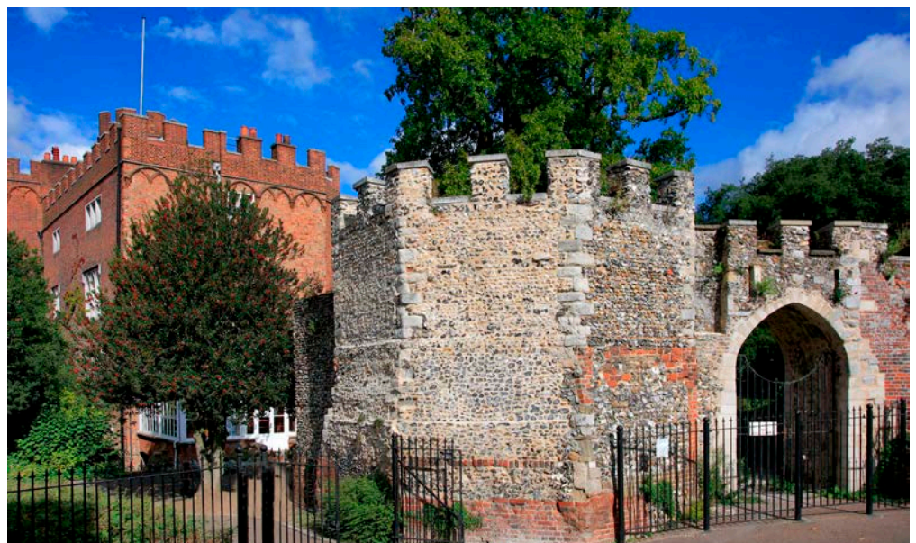
Figure 2: Hertford Castle curtain wall, Hertford. Quaternary Flint and chalk block, with glacial pebbles and cobbles and Quarry Flint nodules.
