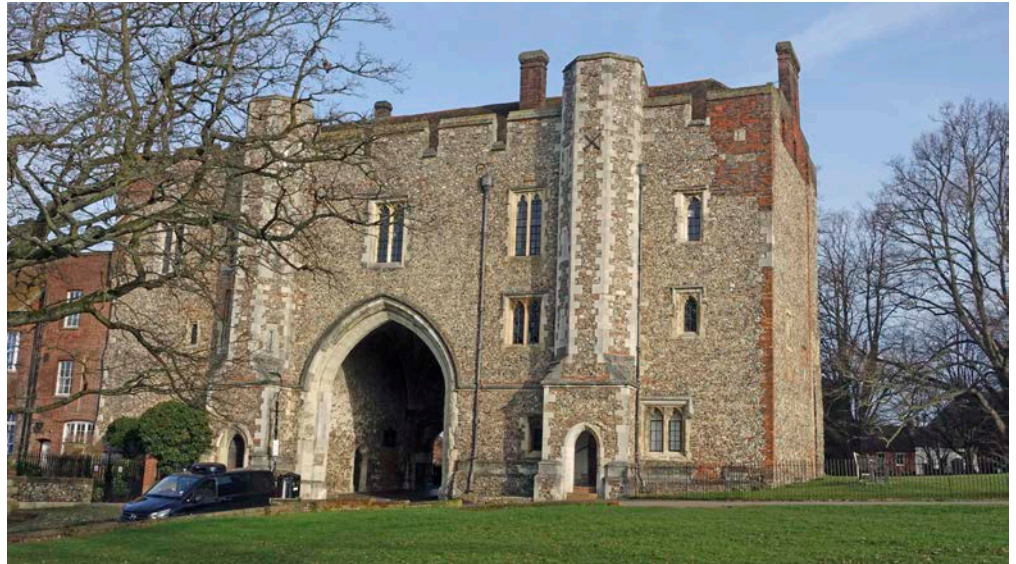
Figure 19: Abbey gate, St Albans. Quarry Flint with chalk block dressings.
