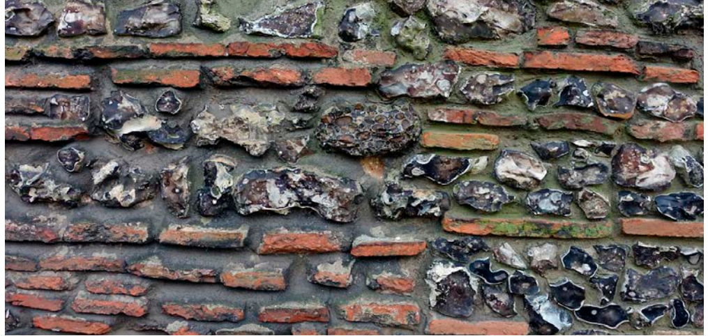
Figure 32: Cathedral nave wall, St Albans. Quaternary Flint pebbles, knapped Quarry Flint, Hertfordshire Puddingstone and Roman tiles.
