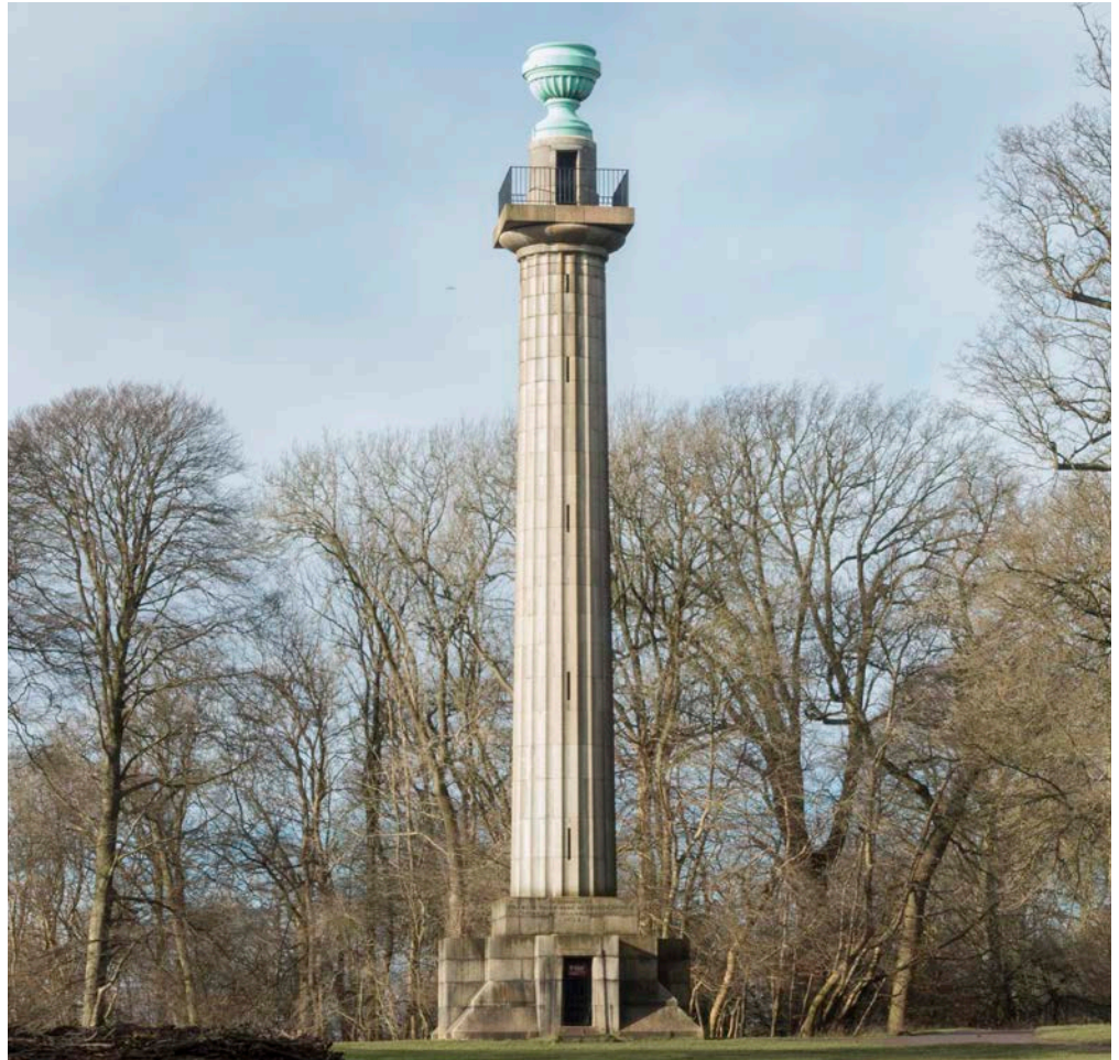
Figure 57: Bridgewater monument, Ashridge Estate, near Berkhamsted. Granite, possibly from Devon or Cornwall.
