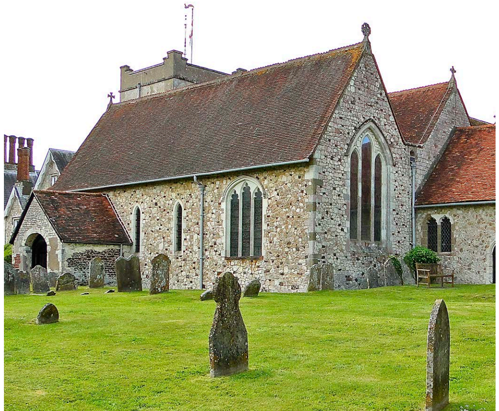
Figure 23: St Mary's Church, Selbourne. Chilmark Stone window repairs.
