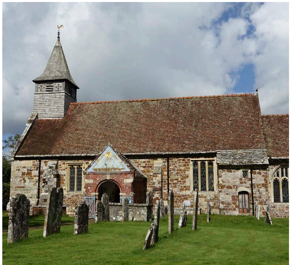
Figure 17: Church of St Mary, Ellingham. Ferricrete, Reading Beds Sandstone and Purbeck Stone with Chilmark Stone dressings.
