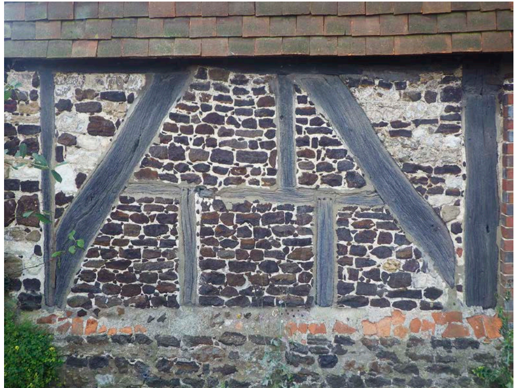
Figure 4: Farmhouse wall, West Liss. Carstone (laid to course) and Malmstone blocks.
