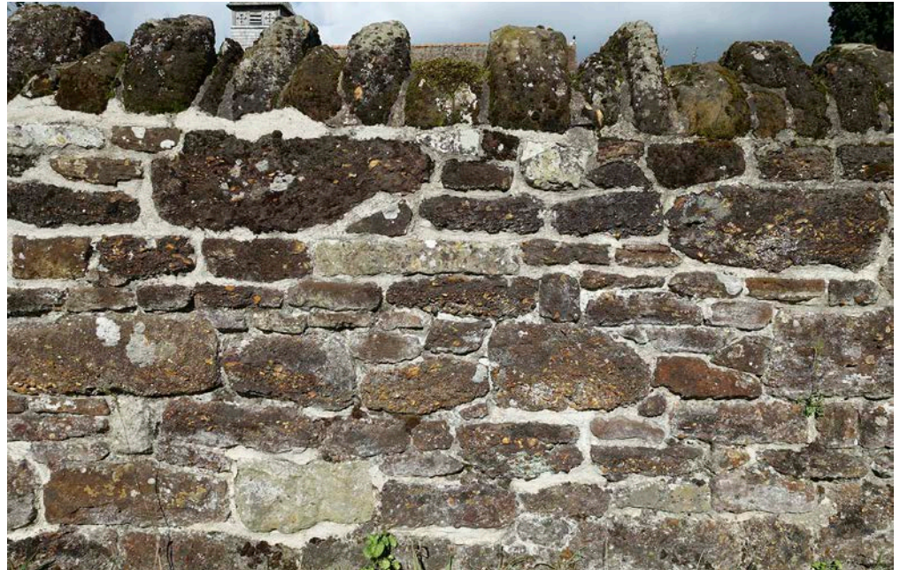
Figure 7: Churchyard wall, Ellingham. Burley Rock, Reading Beds Sandstone and ferricrete.
