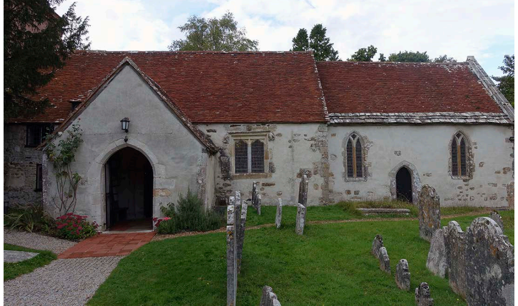
Figure 27: Church of St Nicholas, Brockenhurst. Purbeck Stone slate eaves.
