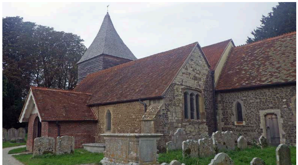
Figure 9: Church of St Peter, West Liss. Bargate Stone, carstone, Malmstone and ferricrete.
