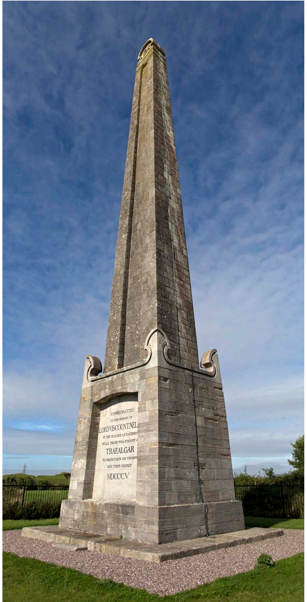
Figure 24: Nelson Monument, Boarhunt. Portland Stone ashlar on a granite base.
