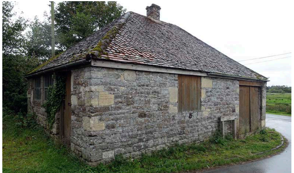
Figure 34: Former blacksmith's shop, London Lane, near Sopley. Reused stone, including Bembridge Limestone.
