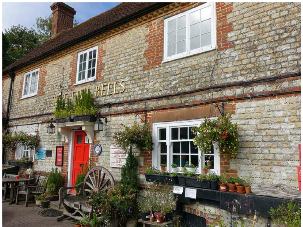
Figure 11: Public house, Buriton. Squared and coursed Malmstone blocks with carstone galleting.
