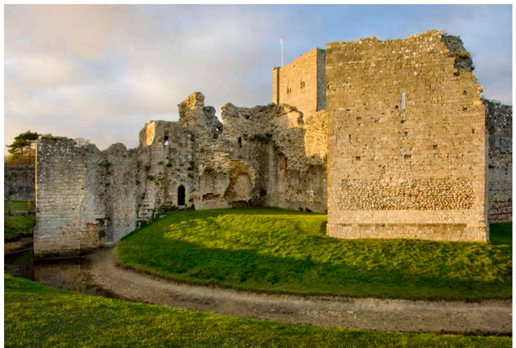
Figure 2: Portchester Castle, near Fareham. Flint walls with Quarr Stone and Nettlestone Sandstone stringers.
