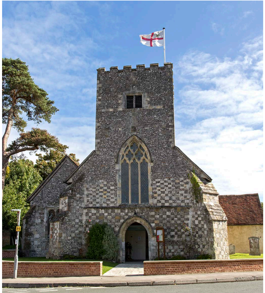
Figure 19: Church of St James, Southwick. Flint chequerwork with Malmstone, Caen Stone and Hambledon Chalk.
