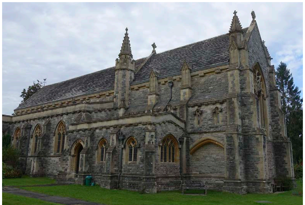
Figure 22: Church of St Saviour, Brockenhurst. Purbeck Stone with Bath Stone dressings and tracery.
