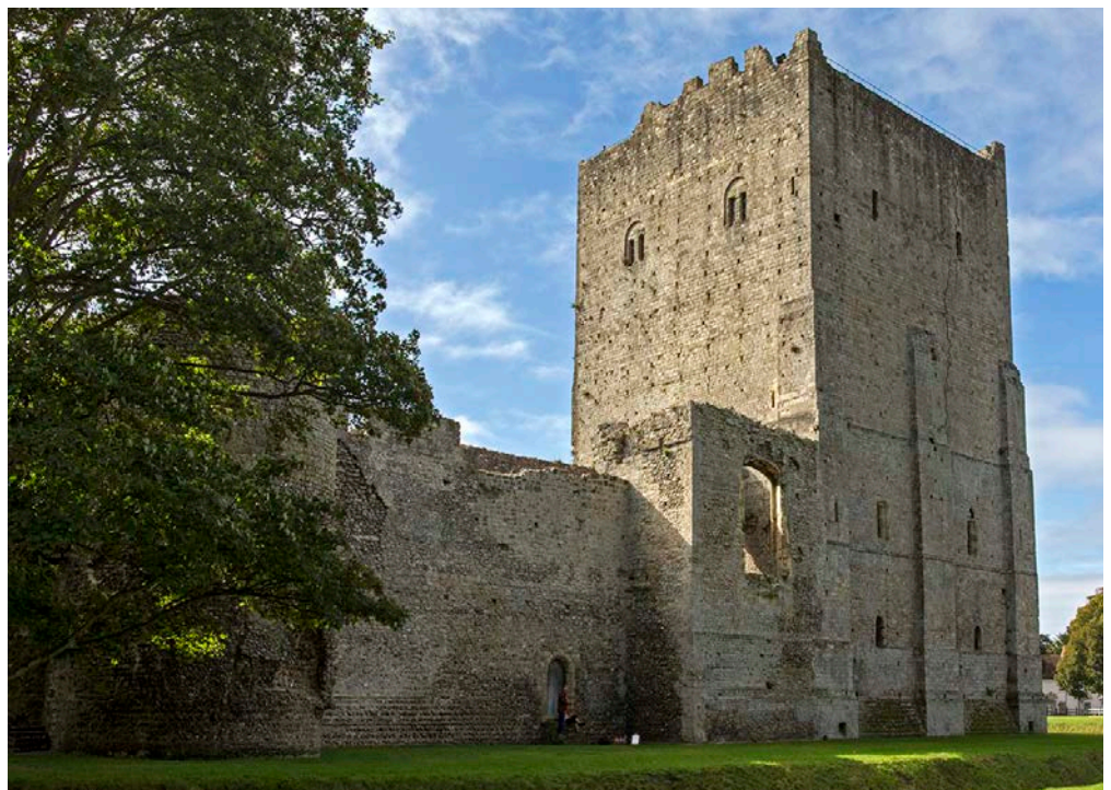
Figure 32: Keep, Portchester Castle, near Fareham. Nettlestone Sandstone and Quarr Stone.
