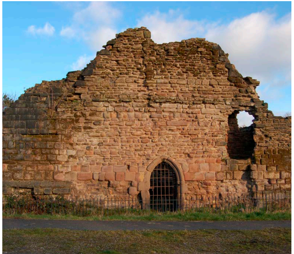
Figure 11: Radcliffe Tower, Radcliffe. Nob End Rock.
