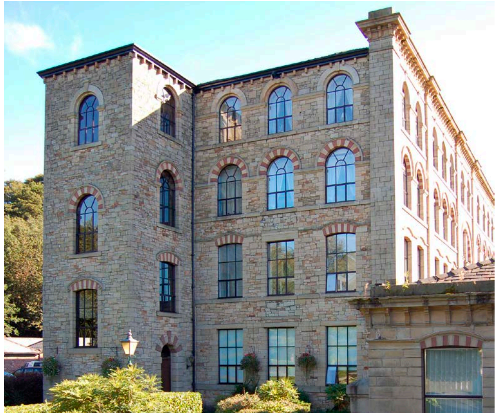
Figure 2: Brooksbottom Mill, Summerseat. Fletcher Bank Grit used for quoins and window surrounds.
