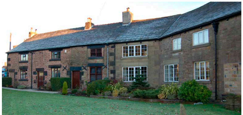
Figure 5: Houses at Blackrod, Bolton. Cannel Rock with Ousel Nest Grit dressings.
