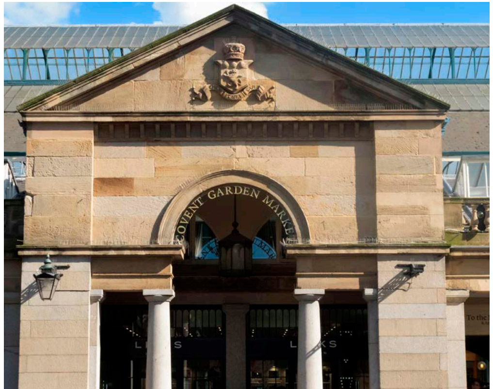
Figure 36: Market building, Covent Garden. Aislaby Stone and Aberdeenshire Dancing Cairns Granite columns.
