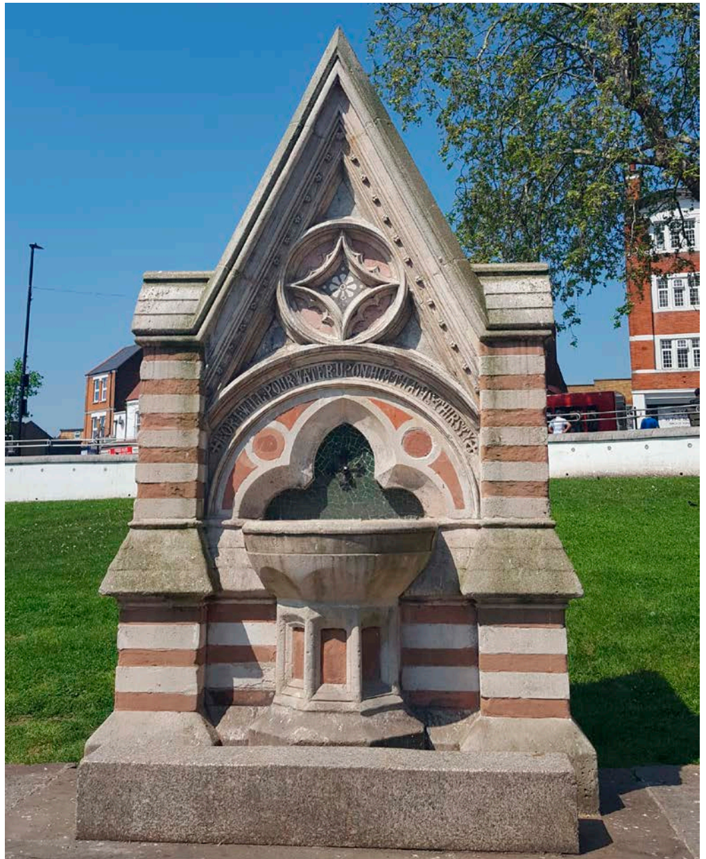
Figure 35: Dyce Drinking Fountain, Streatham Green. Portland Stone and possibly Mansfield Red Sandstone on a Cornish or Devon granite base.
