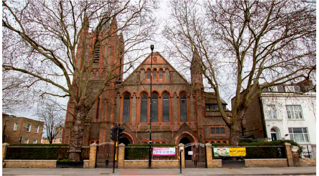
Figure 34: Former Congregational Church, Forest Gate. Knapped flint with Permo-Triassic sandstone and brick dressings.
