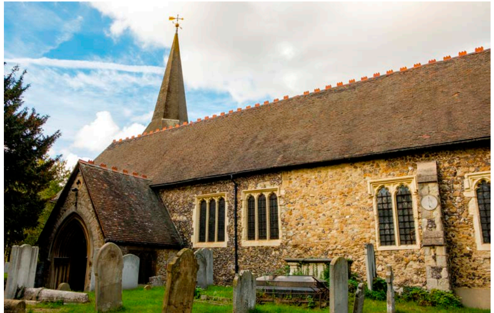
Figure 9: Church of St John the Baptist, Erith. Quaternary Flint, with chalk and stone reused from Lesnes Abbey, Bexley.
