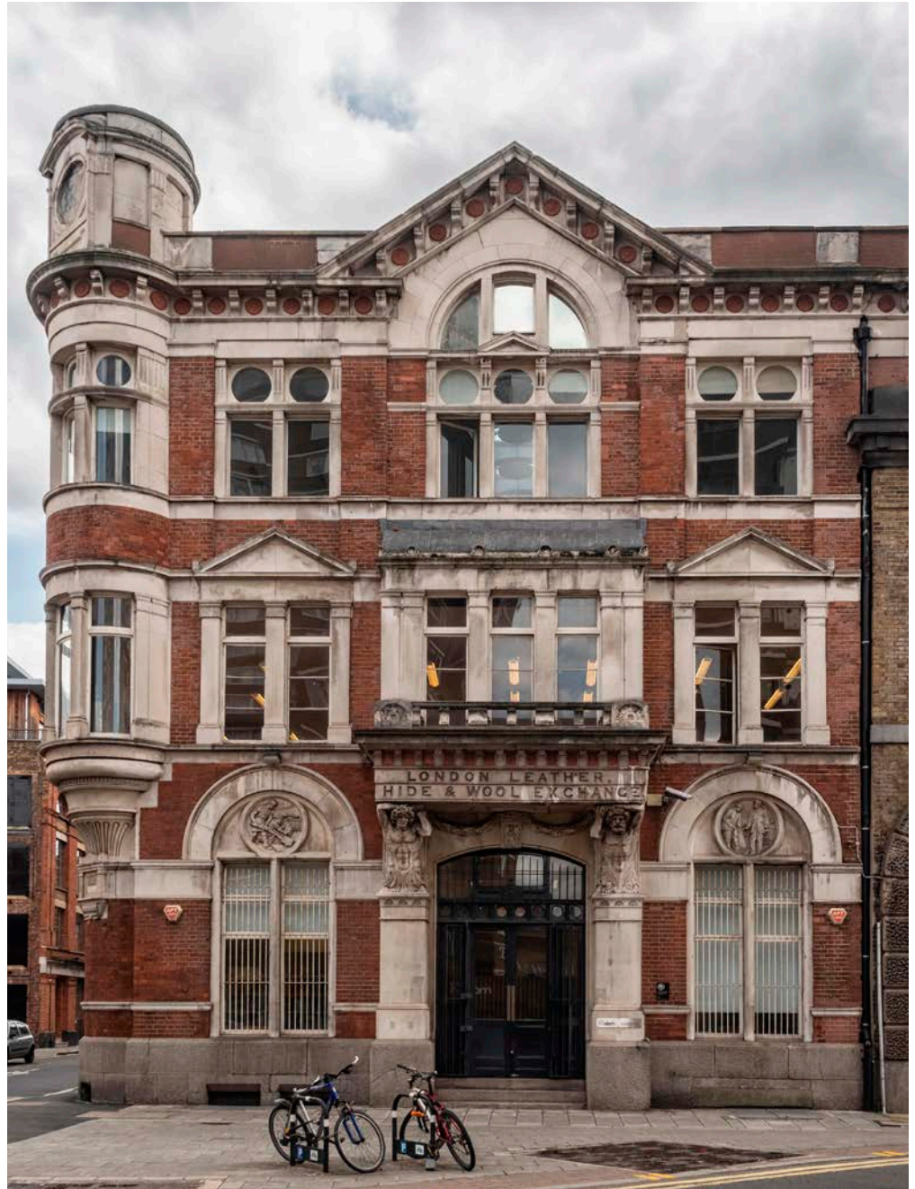
Figure 12: London Leather Hide and Wool Exchange, Southwark. Brick and Portland Stone dressings.
