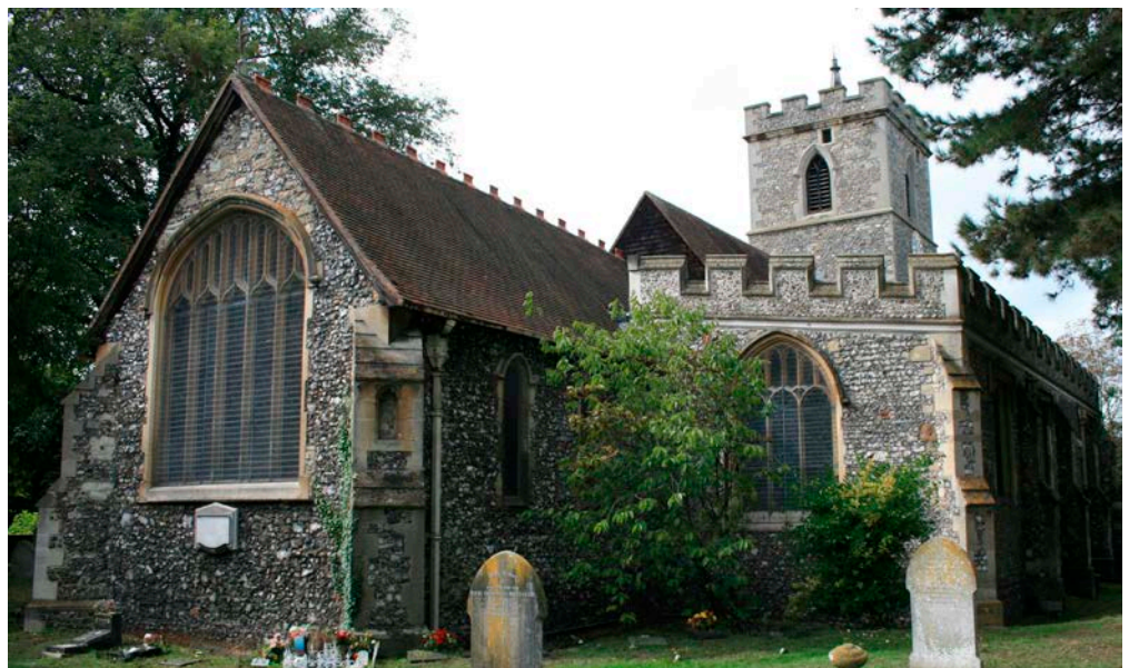
Figure 44: Church of St Mary the Virgin, Hayes. Quaternary Flint with Reigate Stone dressings.
