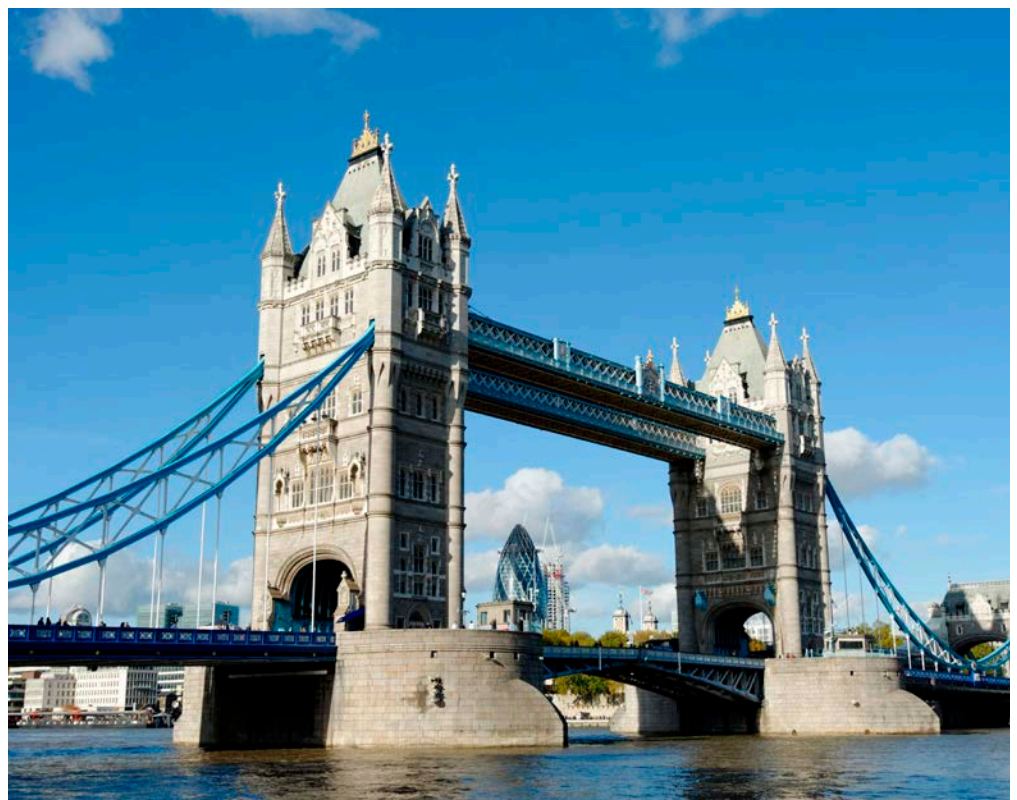
Figure 32: Tower Bridge, River Thames. Cornish Granite foundations, Kentish Ragstone and Portland Stone towers.
