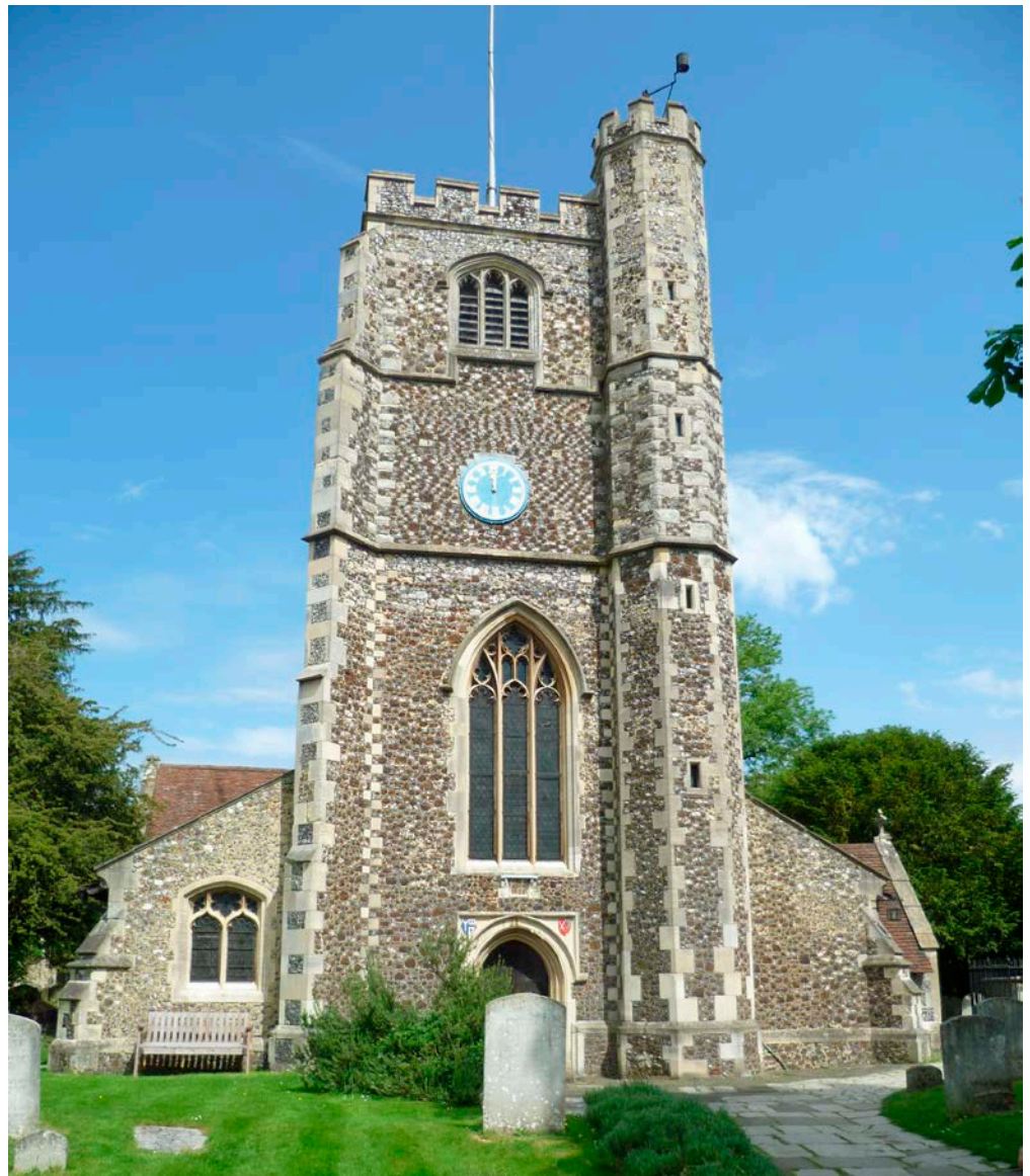
Figure 23: Church of St Mary the Virgin, Monken Hadley. Septaria and Quaternary Flint nodules, with Bath Stone dressings.
