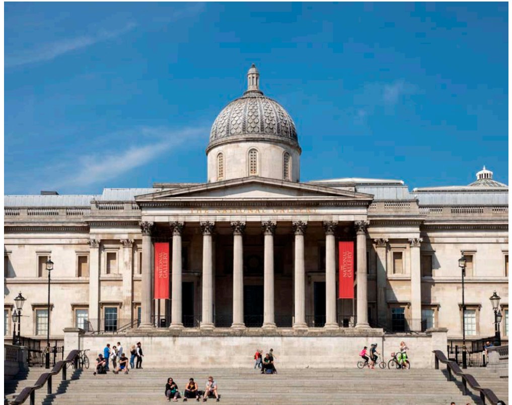
Figure 31: National Gallery, Trafalgar Square. Portland Stone and Libishaw Sandstone.
