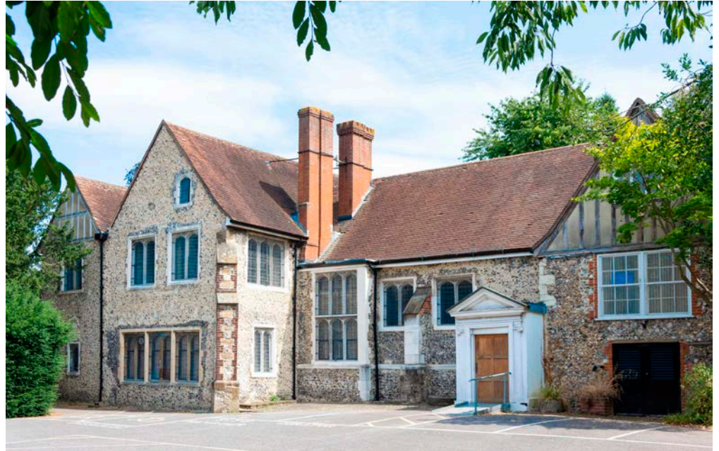
Figure 17: The Priory, Orpington. Quaternary Flint and chalk with Portland Stone dressings.
