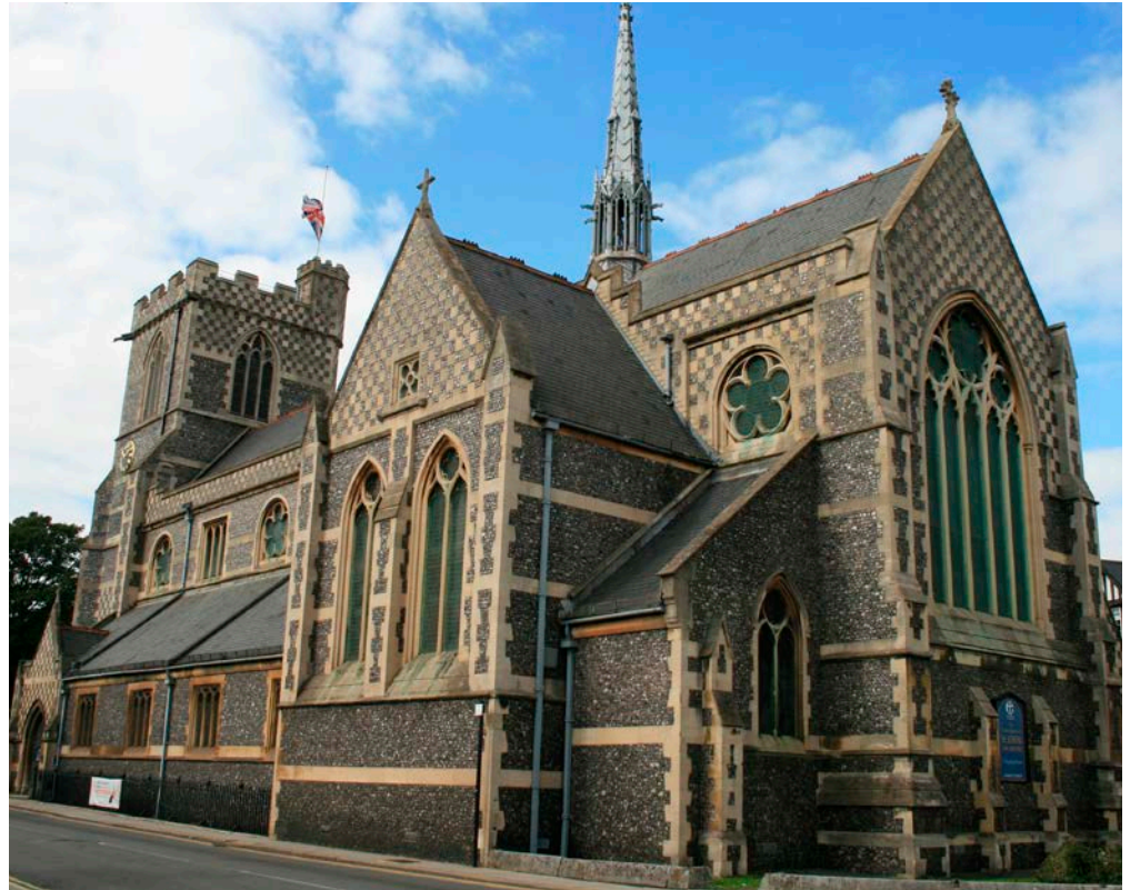
Figure 20: Church of St John the Baptist, Chipping Barnet. Quarry Flint, Quaternary Flint, Bath Stone and Ancaster Stone.
