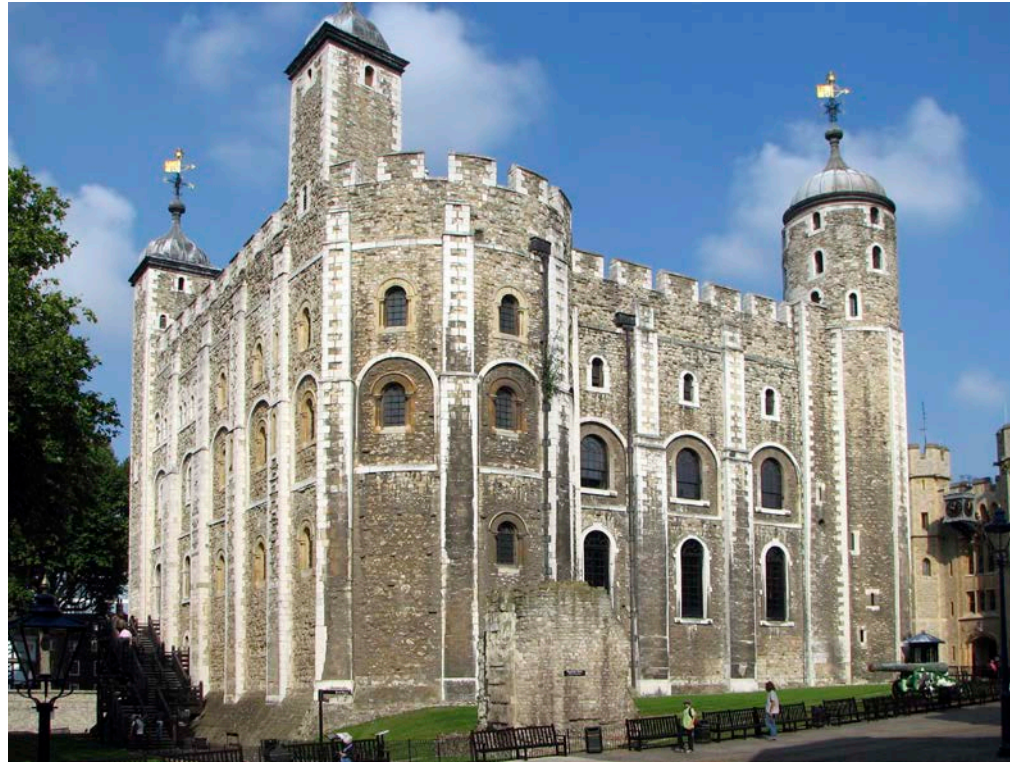
Figure 42: White Tower, Tower of London. Kentish Ragstone, with some Portland Stone, Quarr Stone, Binstead Stone and Reigate Stone.
