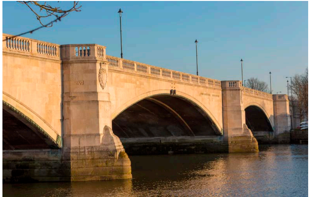
Figure 16: Chiswick Bridge. Portland Stone facing on reinforced concrete.
