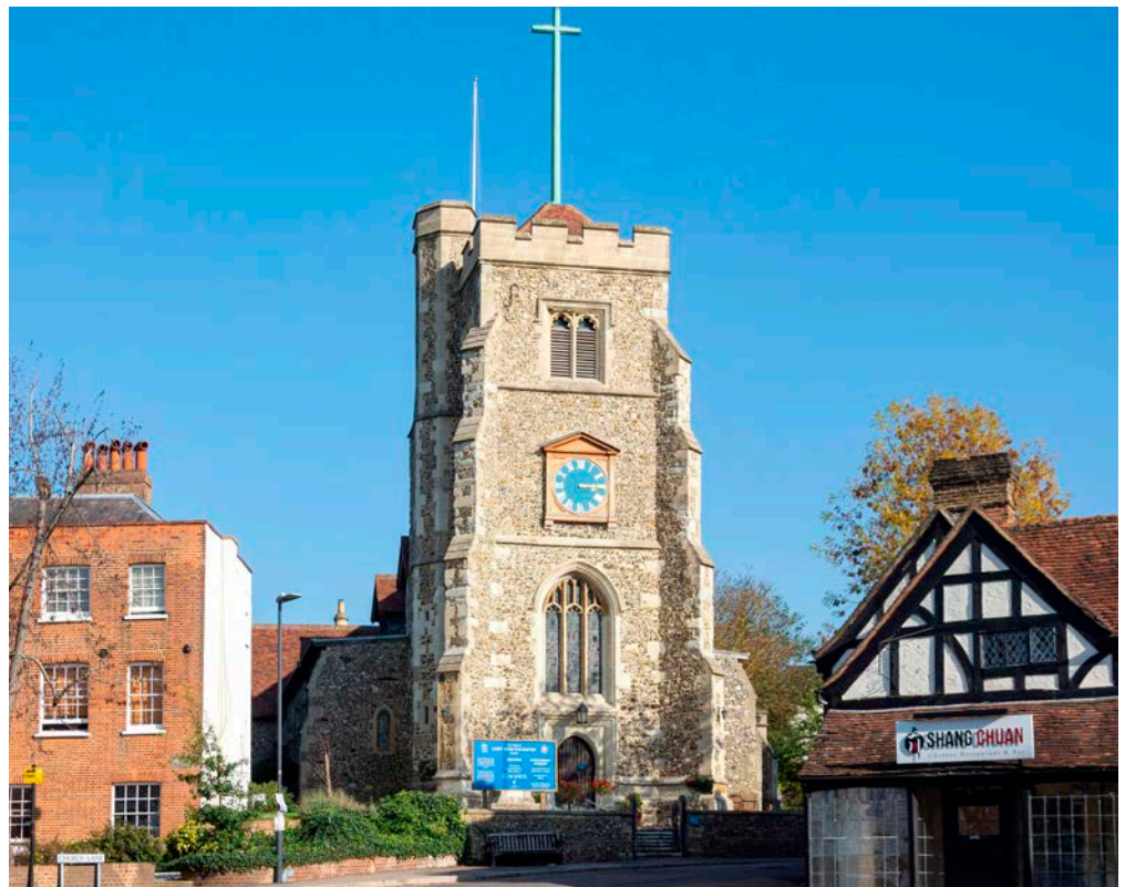
Figure 10: St John the Baptist Church, Pinner. Hertfordshire Puddingstone with flint and ironstone quoins.
