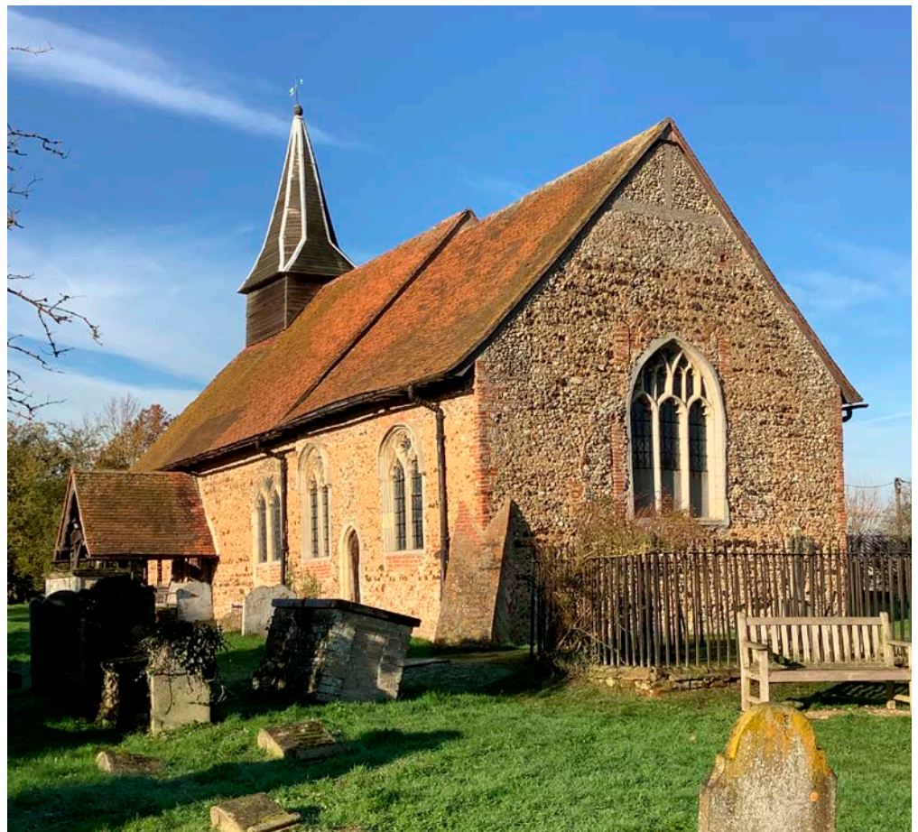
Figure 6: Holy Trinity Church, Bradwell. Flint, pebble and cobble rubble, ferricrete and Roman tile.
