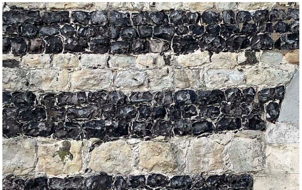
Figure 13: Church of St Clements, West Thurrock. Quarry Flint and Kentish Ragstone banding.
