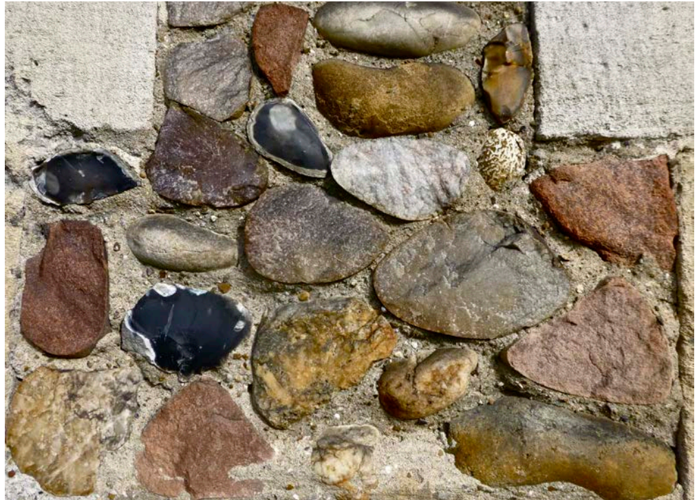
Figure 51: Cathedral wall, Chelmsford. Split quartzite pebbles.
