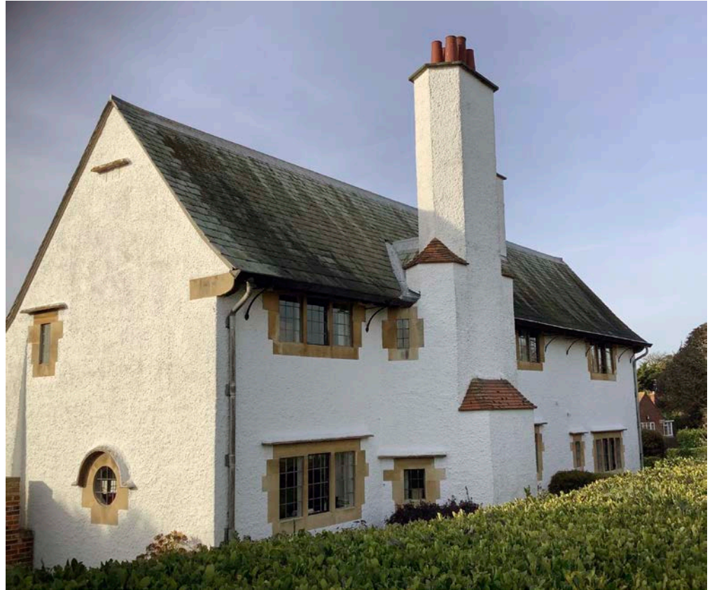
Figure 73: The Homestead, Frinton-on Sea. Bath Stone dressings and a Westmorland Slate roof.
