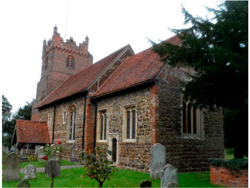
Figure 38: Church of St Mary the Virgin, Fryerning. Conglomeratic Ironstone, Roman brick and flint rubble, with limestone, chalk and Roman brick dressings.
