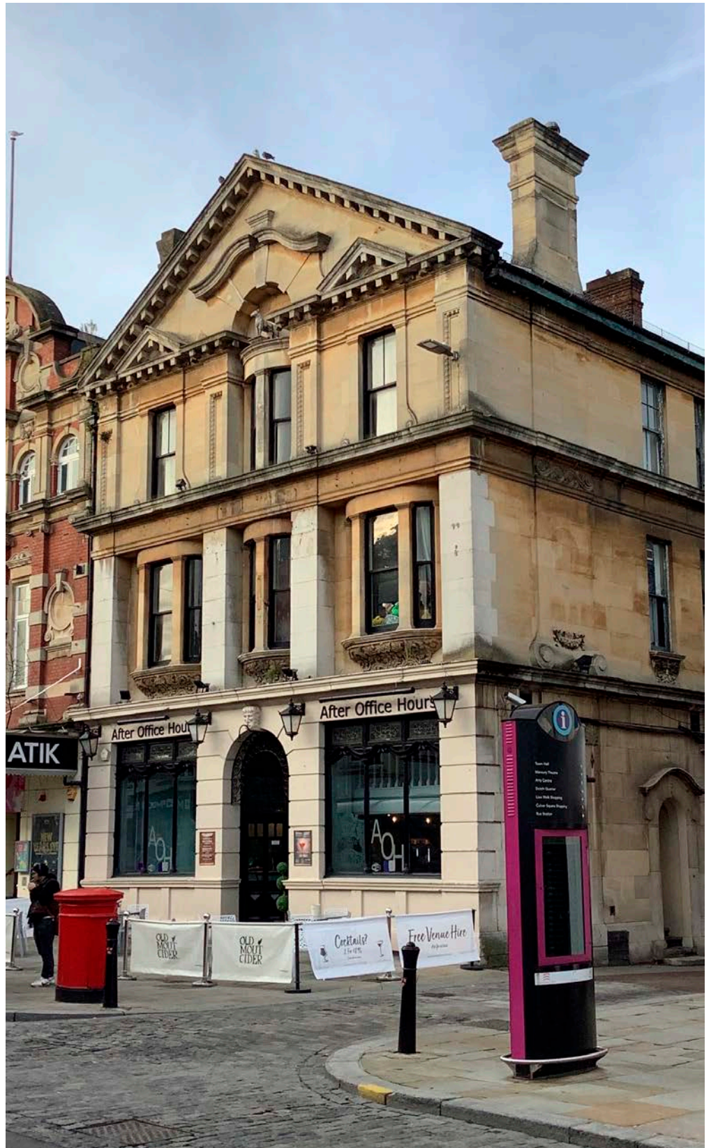
Figure 11: 128 High Street, Colchester. Portland Stone with Bath Stone facade.
