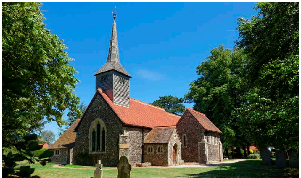
Figure 63: Church of St Mary, Stapleford Tawney. Quaternary Flint and Purbeck Limestone.
