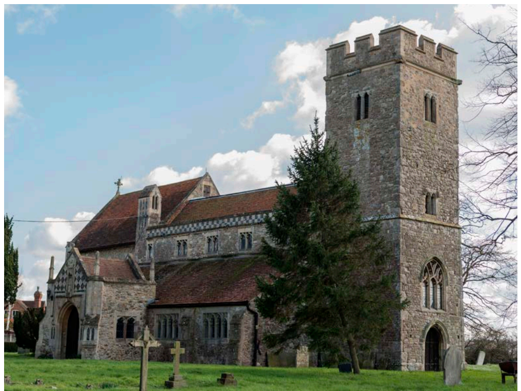
Figure 10: St Nicholas' Church, Rawreth. Kentish Ragstone with flint flushwork and Bath Stone dressings.
