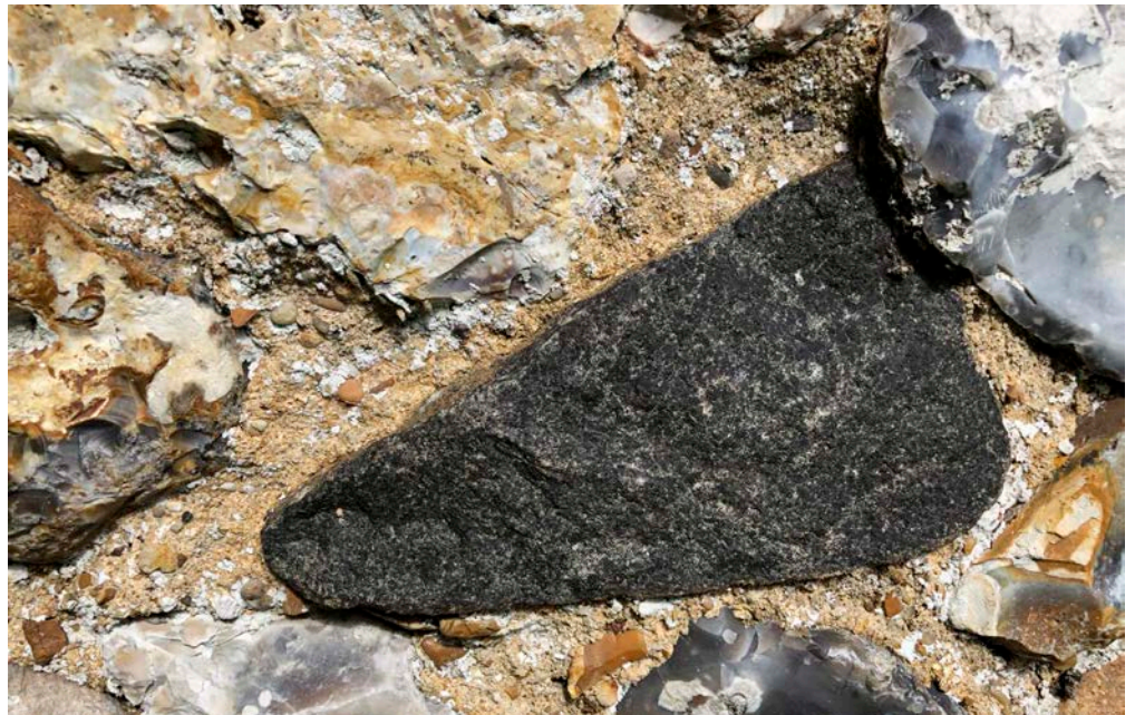
Figure 71: Church of St Katharine, Little Bardfield. Dolerite pebble.
