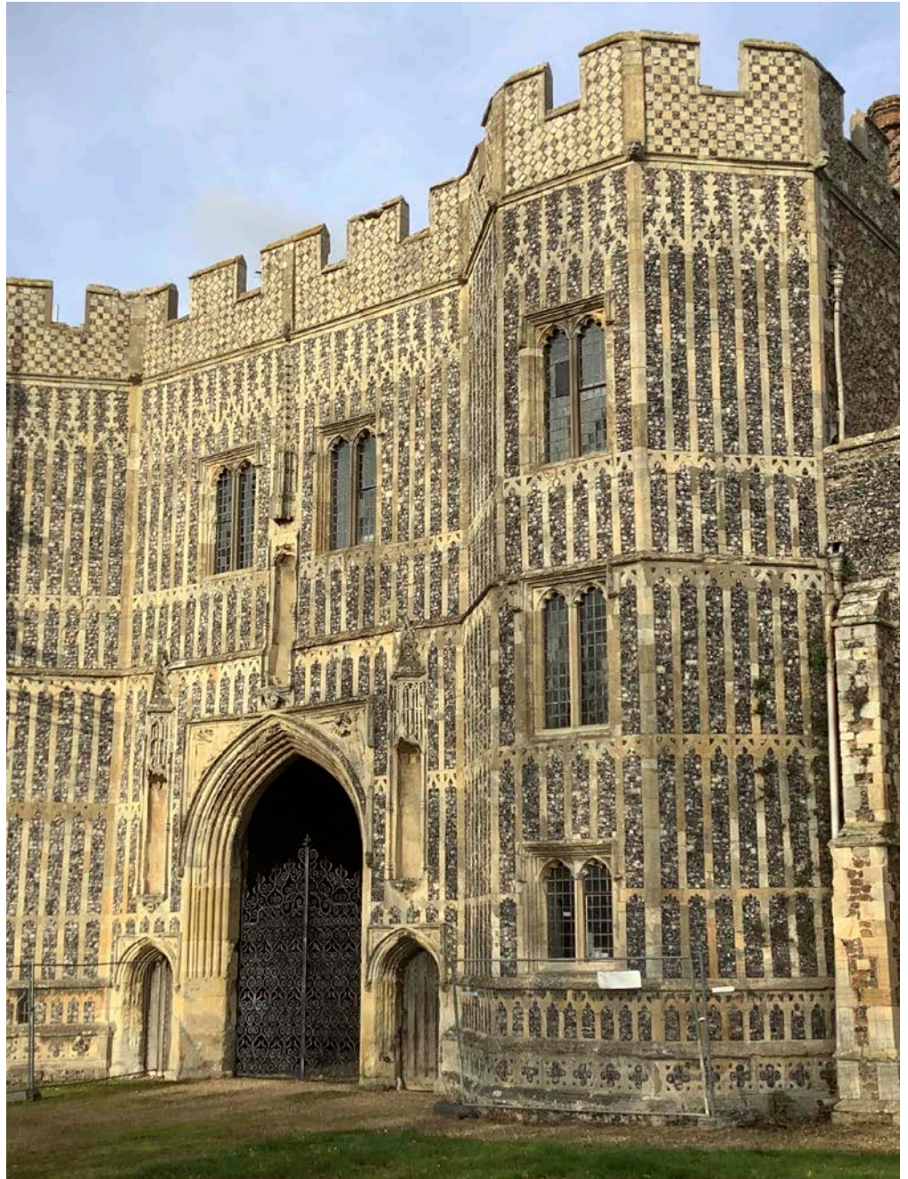
Figure 14: Priory of St Osyth, near Clacton-on-Sea. Flint flushwork.
