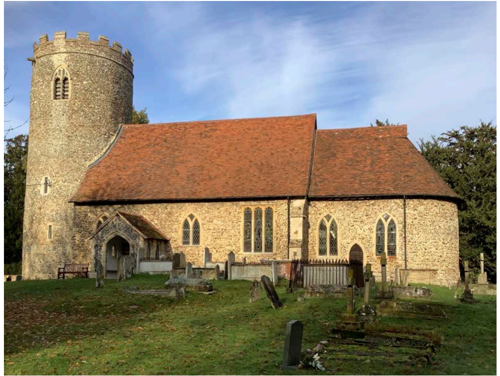
Figure 5: Church of St Gregory and St George, Pentlow. Whole flints, pebbles and cobbles with large flint quoins.
