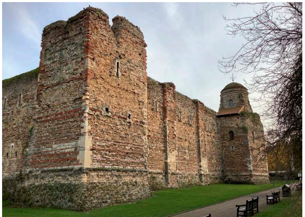
Figure 25: Castle Keep, Colchester. Cementstone, Barnack Stone and Caen Stone.
