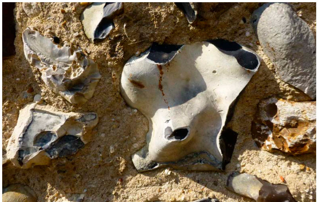
Figure 15: Mashbury Church wall, near Chelmsford. Quarry Flint nodule.
