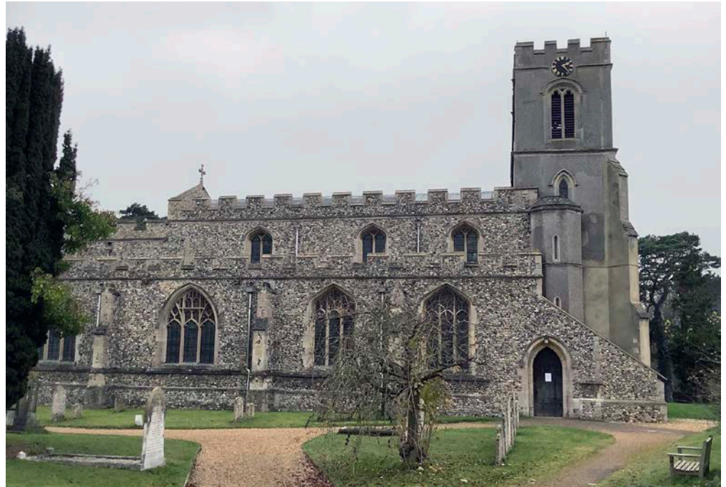
Figure 20: All Saints' Church, Great Chesterford. Flint, pebbles and cobbles, chalk and limestone, with a plinth course in ashlar.
