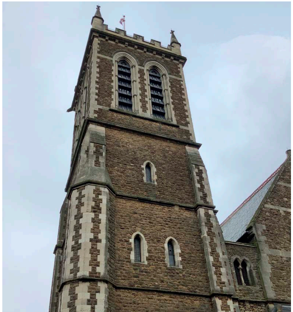
Figure 65: Church of All Saints, Chigwell Row. Bargate Stone with Bath Stone dressings.
