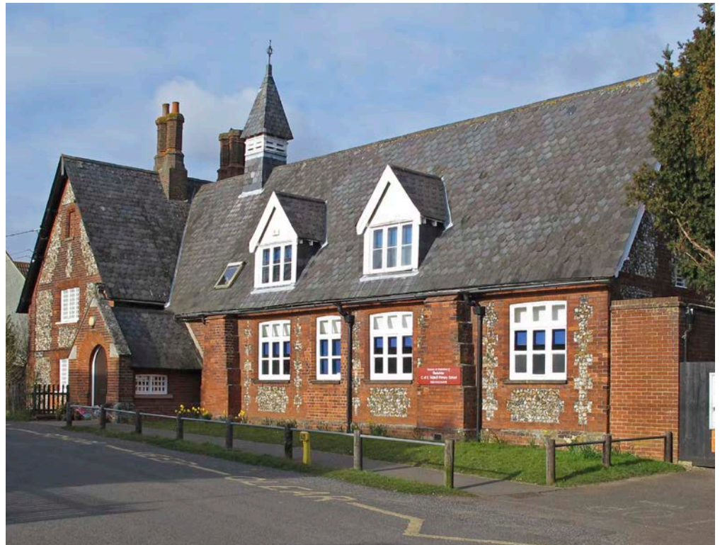
Figure 8: Radwinter School, Radwinter. Flint rubble and brick.
