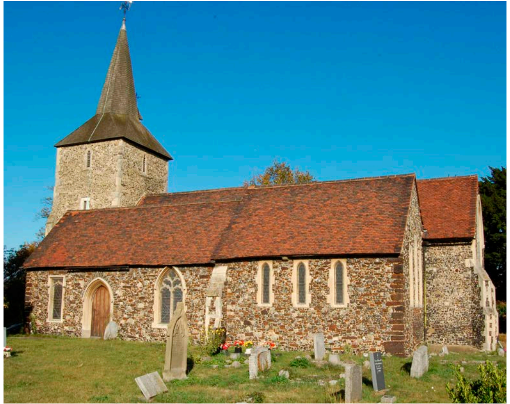
Figure 26: Church of St Mary, North Stifford. Ferricrete and Quaternary Flint with Bath Stone and Reigate Stone dressings.
