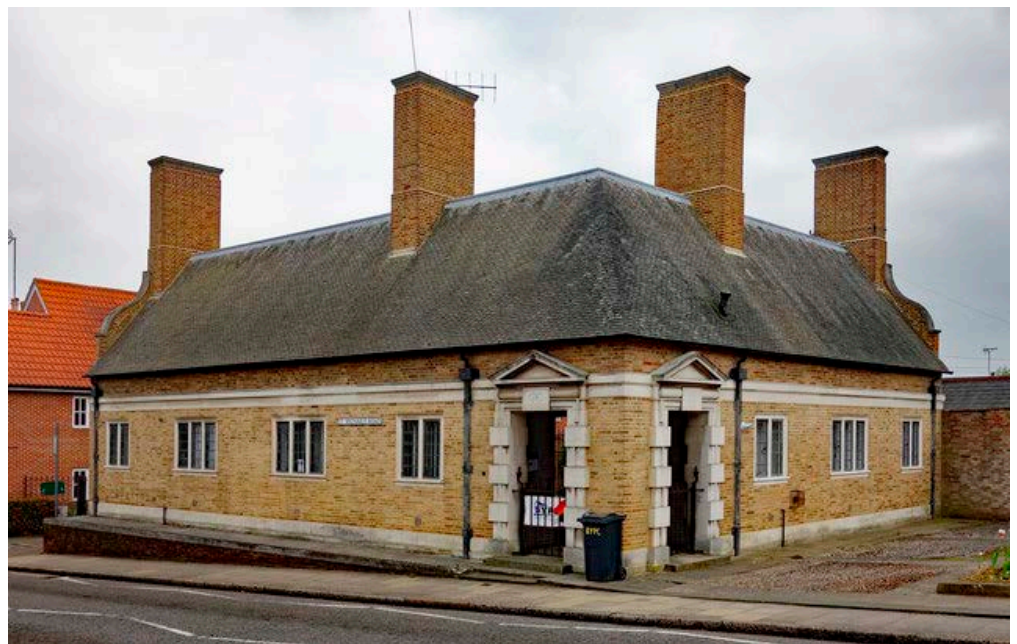
Figure 74: Former almshouses, St Michael's Road, Braintree. Northwick brick with Portland Stone string courses and dressings, and a Delabole Slate roof.
