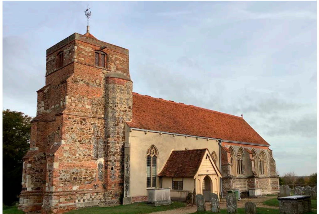
Figure 22: Church of St Mary the Virgin, Lawford. Quaternary flint, Cementstone, Conglomeratic Ironstone and Roman tiles, with limestone dressings.
