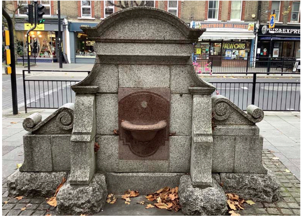
Figure 67: Larkin's horse trough, High Street, Shenfield Common. Cornish Granite with a Peterhead Granite bowl.
