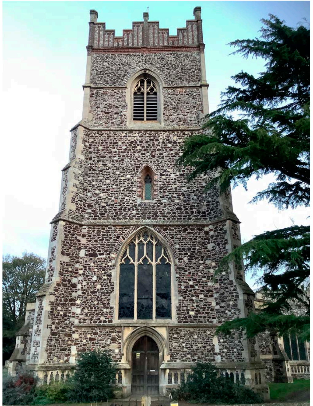
Figure 29: Church of St Mary, Ardleigh. Ferricrete, Quaternary Flint, pebbles and cobbles, cement stone and Roman brick, with limestone and brick dressings.
