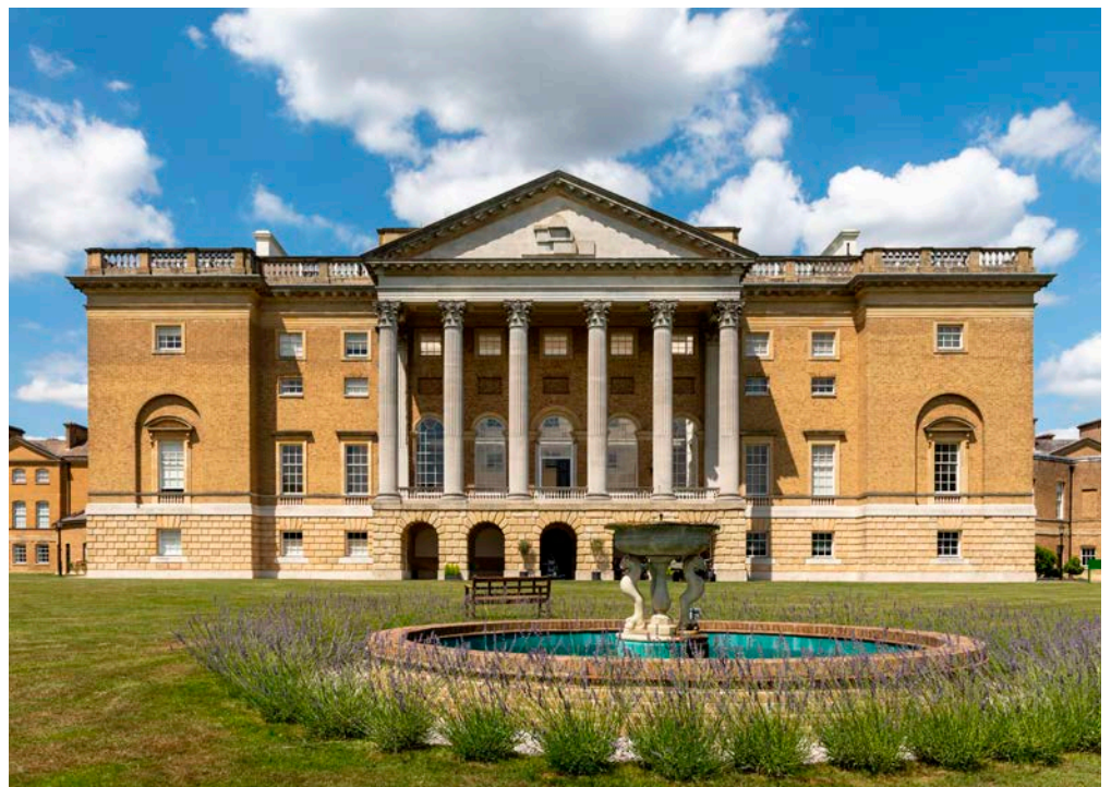
Figure 9: Thorndon Hall, Ingrave. Limestone rustication and columns.
