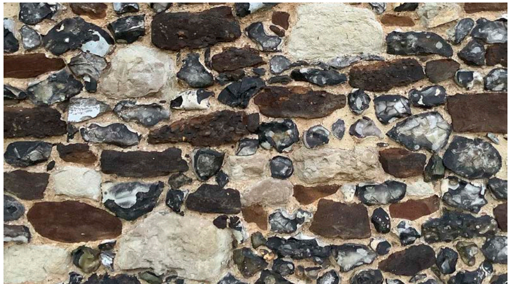
Figure 27: Church of St Mary, North Stifford. Ferricrete and knapped flint with Reigate Stone blocks.
