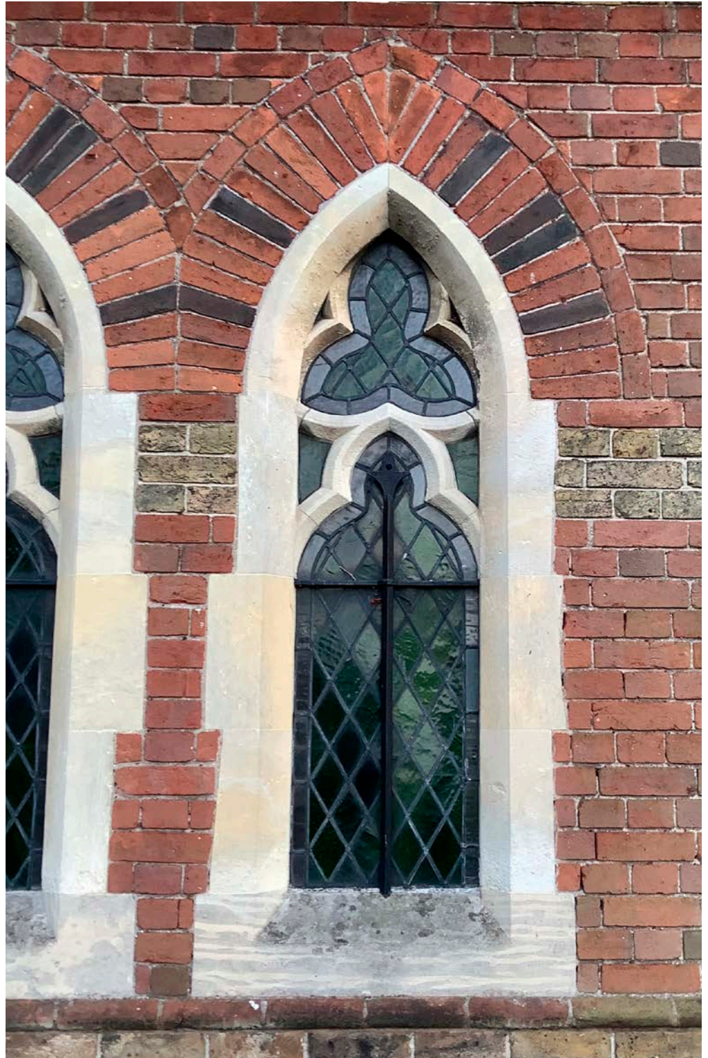
Figure 56: Church of St John, Highwoods, Colchester. Red and gault brick with limestone dressings, including Ancaster Stone.
