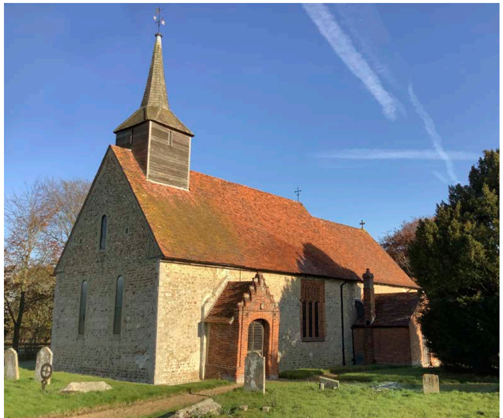
Figure 46: Church of St Germanus, Faulkbourne. Tufa, Kentish Ragstone, Quaternary Flint and vein quartz pebbles and cobbles, with Barnack stone dressings.
