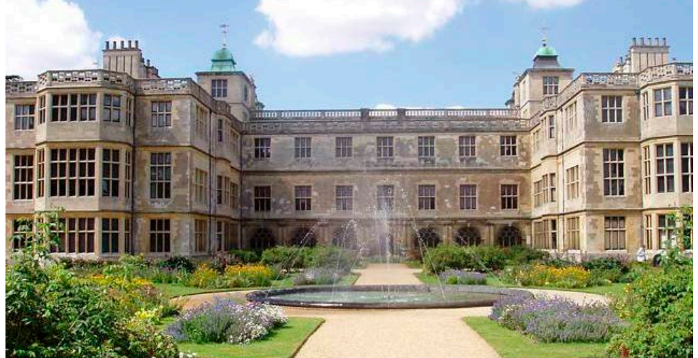
Figure 62: Audley End House, near Saffron Walden. Chilmark Stone ashlar.
