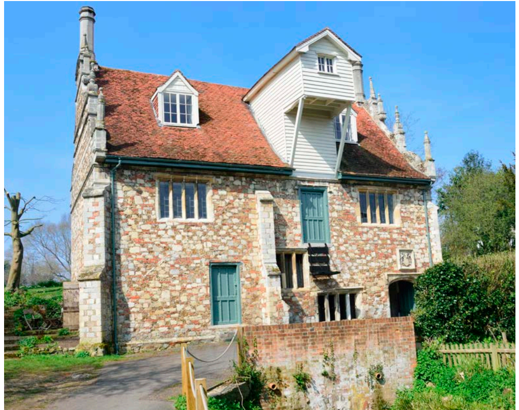
Figure 57: Bourne Mill, Colchester. Barnack Stone.
