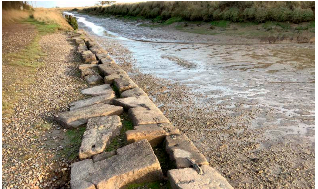
Figure 44: Beaumont Quay, Hamford Water. Reigate Stone and Sarsen stone.
