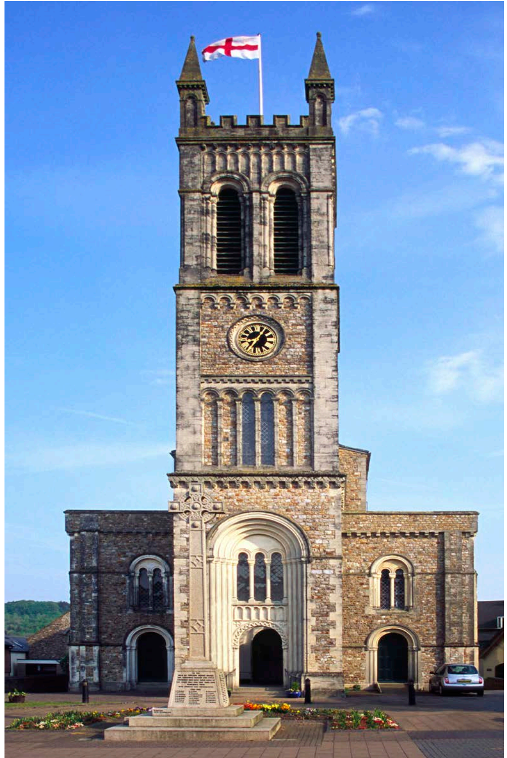
Figure 21: Church of St Paul, Honiton. Green Glauconite Sandstone and Beer Stone tracery.
