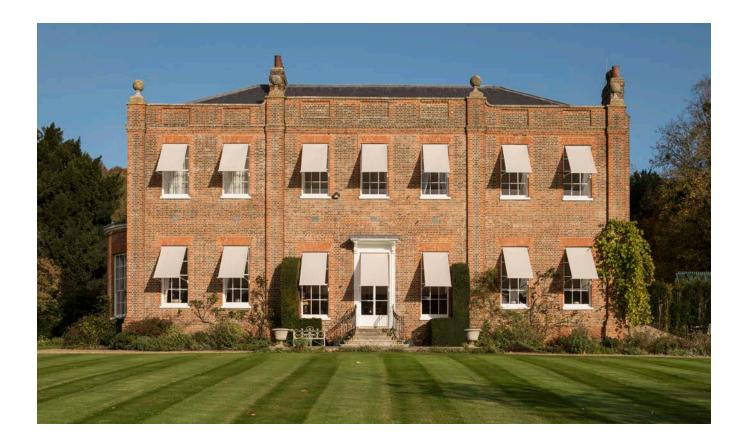
Figure 14: Rooms on the southwest elevation of this Grade II\* house increasingly suffered from overheating in summer. Historic fixings for external awnings were identified in the window reveals and replacement blinds were fitted. © Historic England
