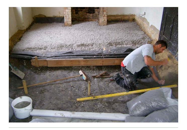
Figure 6: An insulated hydraulic lime floor being laid. © Matthew Clements/Mike Wye Ltd
