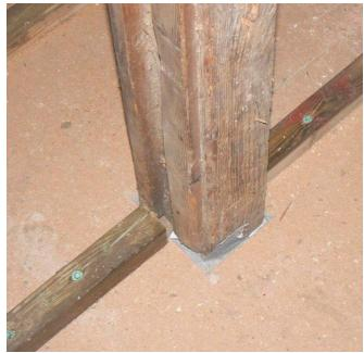
**Figure 7:** Battens have been added at the sides of the joists to support boarding to carry compressible sheep's wool insulation. © Oxley Conservation
