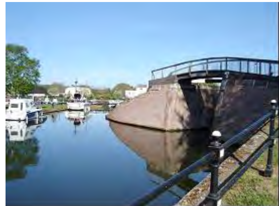
Barge Lock after
