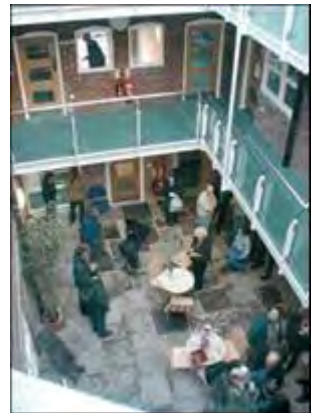
Scotia Works after
