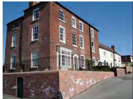
House in Severnside after
