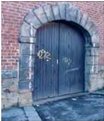
Scotia Works before
