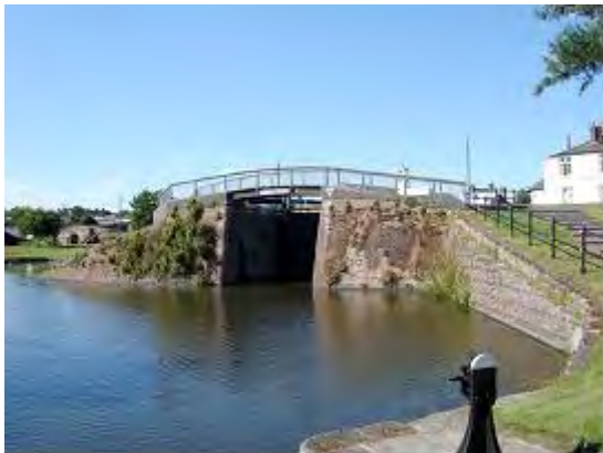
Barge Lock before
