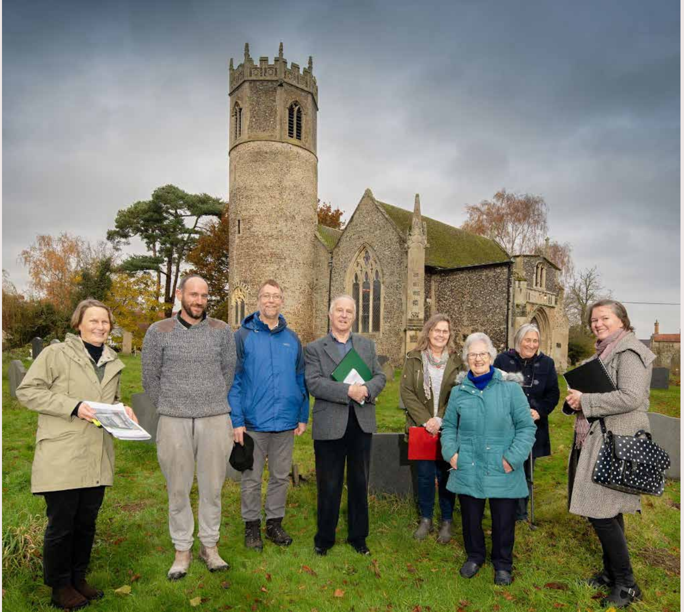
St Mary Rickinghall Inferior, Suffolk, a round tower church. A Taylor Pilot grant of £7,500 helped with repointing, replacement of roof tiles and new guttering. A community meeting encouraged local residents to offer funding, time and skills, including new volunteers to take care of maintenance in the future. The church team commented that they “now feel they have a clear way forward” to develop their plans and are sharing lessons learned to help support other churches in the area. © Historic England Archive
