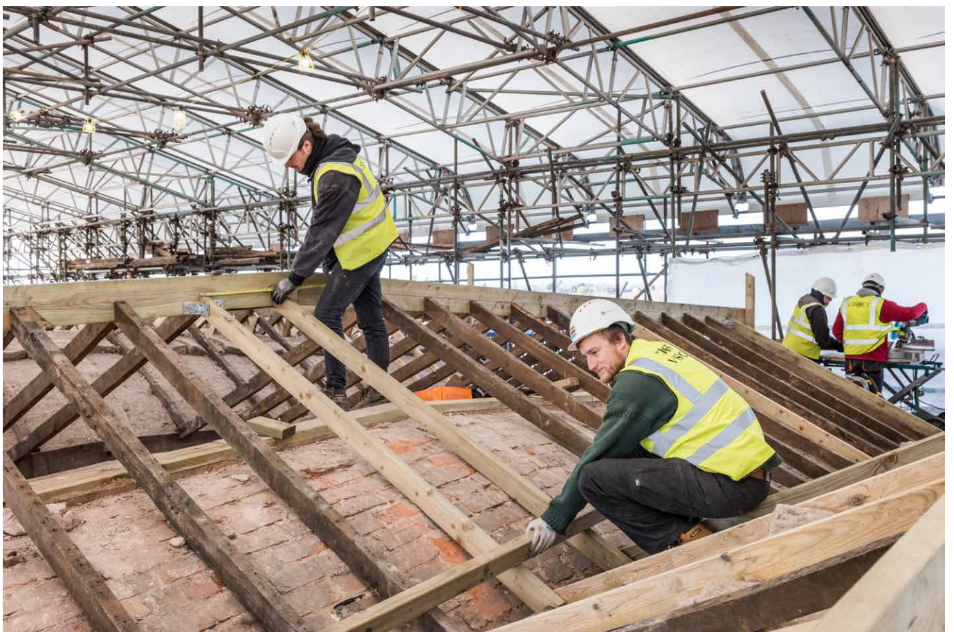
Construction work at Shrewsbury Flaxmill Maltings, Shropshire. © Historic England Archive
