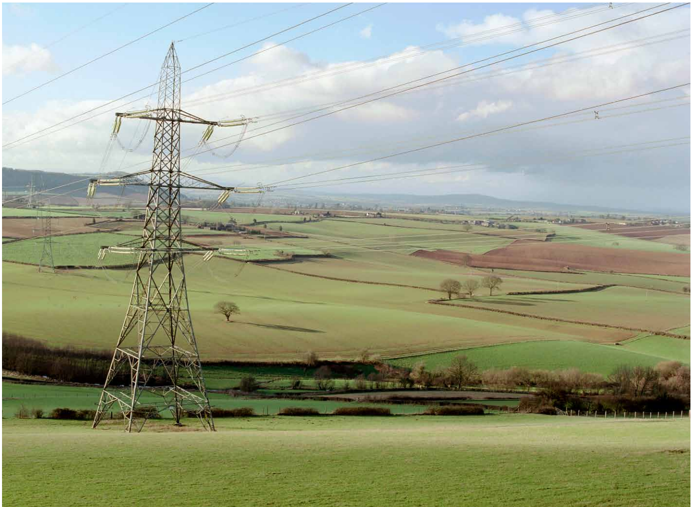
Visual Impact Provision (VIP), project to remove overhead electricity cables and pylons. © Historic England Archive
