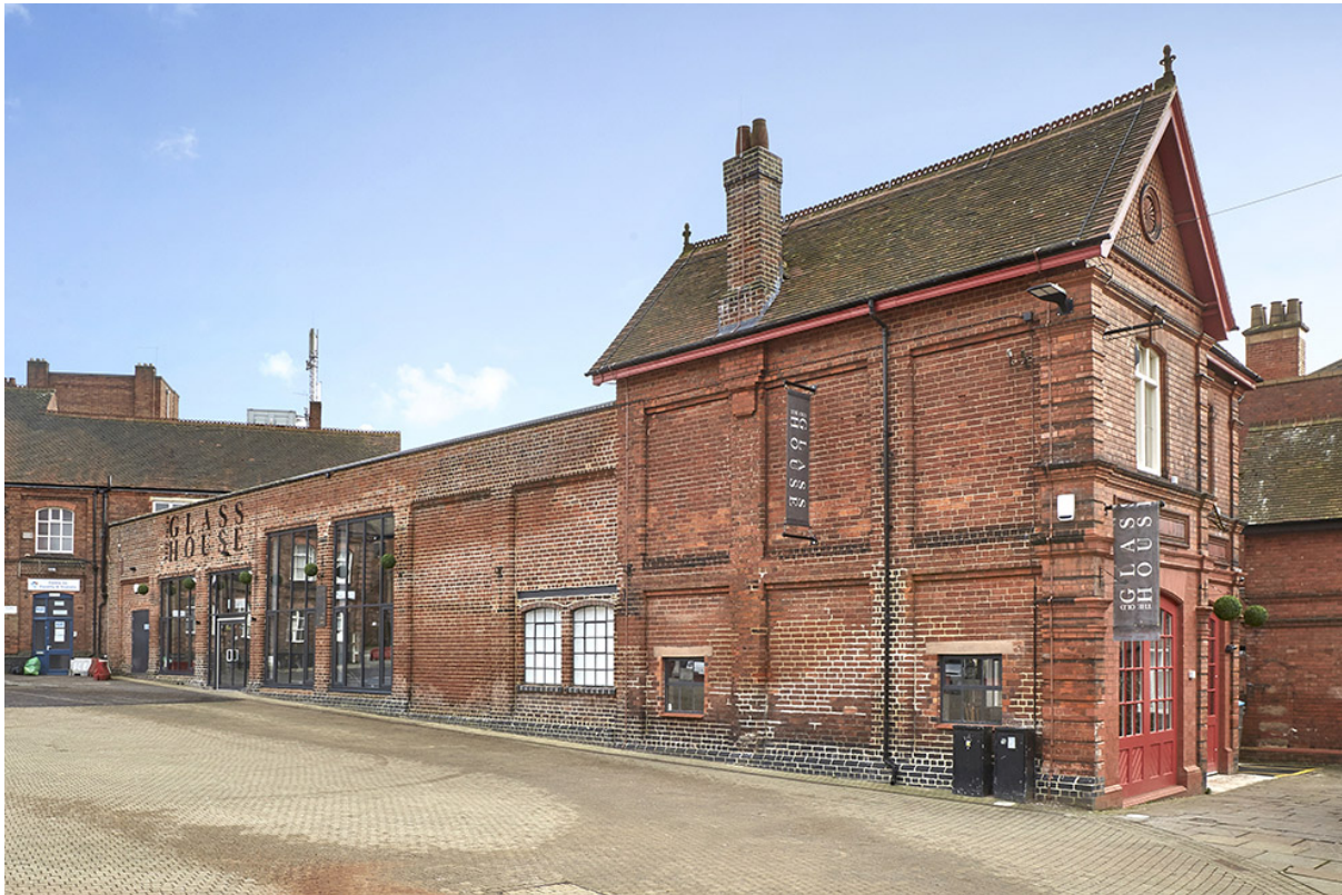
The Old Glasshouse refurbishment which won the 2017 West Midlands RTPI Award for Excellence was part funded through a HE Partnership Scheme. © Brown Haywood Brown Architects
