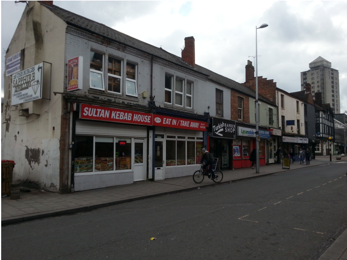
Conservation issues on Hales Street. © Coventry City Council
