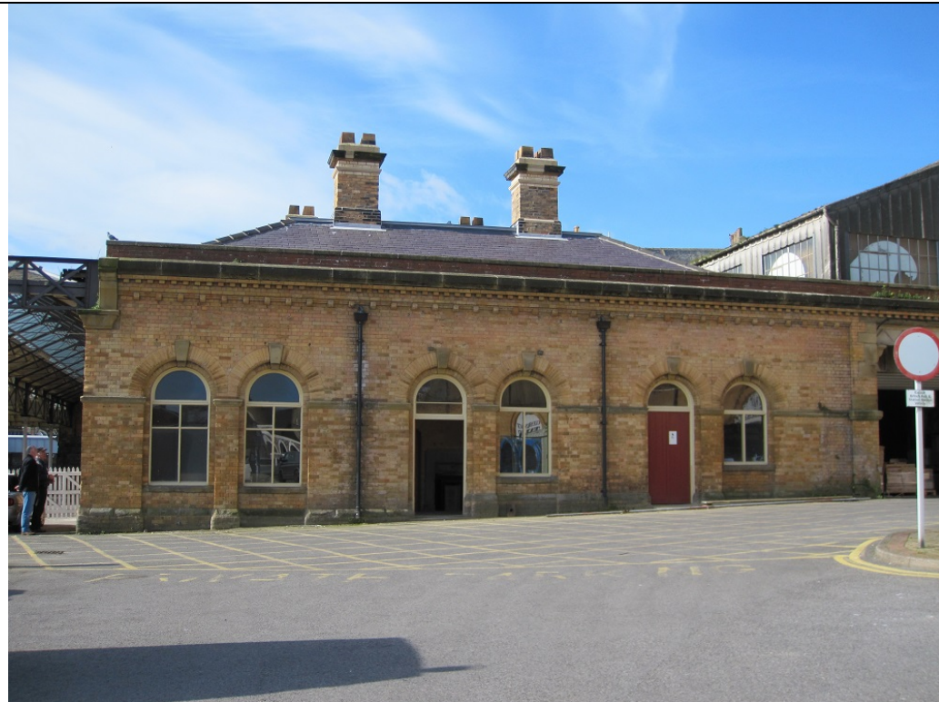
The car park elevation of the repaired building (Photo: © Scarborough Studios Ltd).
