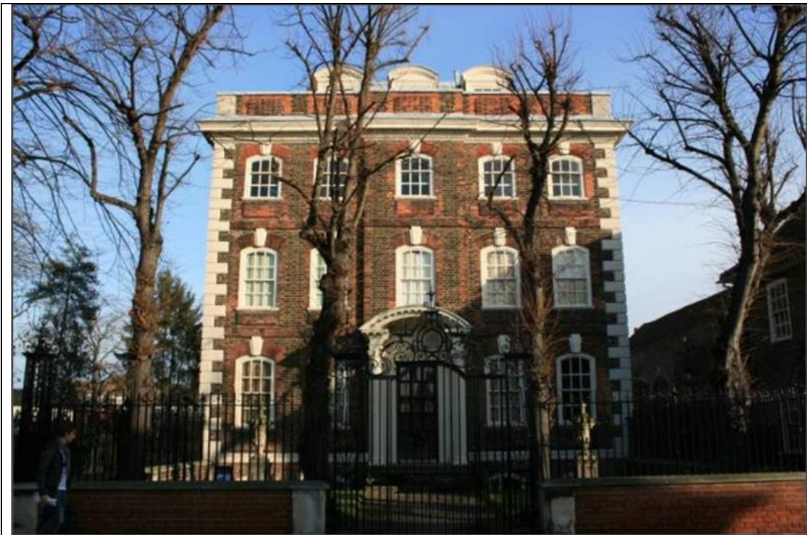
The Rainham Hall prior to the project (Photo: Nic Durston, National Trust).
