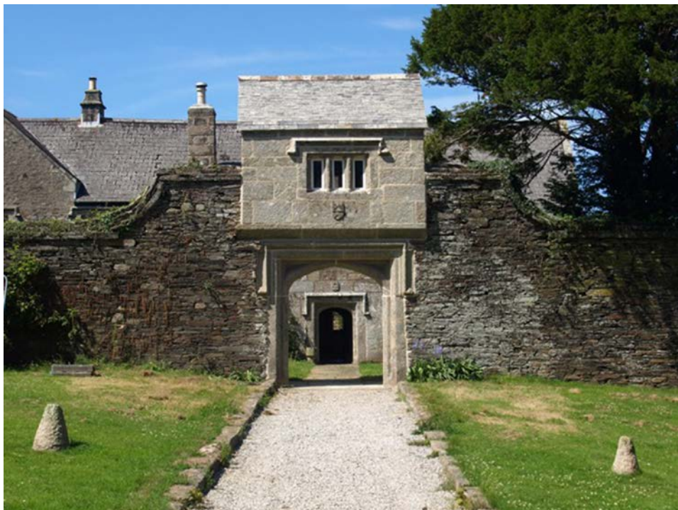
Trenethick Barton Gatehouse, Wendron (Eric Berry/Cornish Buildings Group ©)
