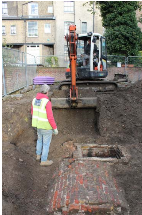
A digger on site at Breaker's Yard © National Trust
